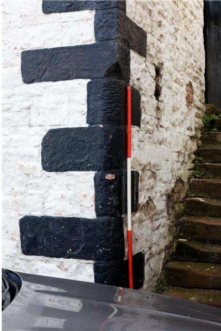
Plate 3: South-west corner of the building showing detail of chamfering.
