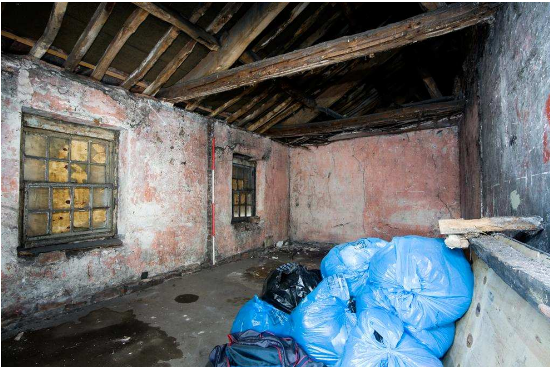
Plate 6: General view of Room 15
