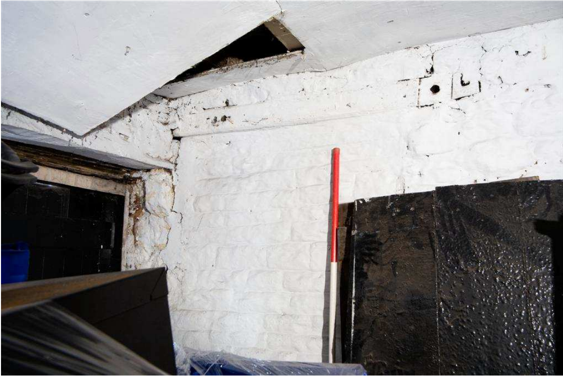
Plate 5: Blocked door within the north wall of Room 10
