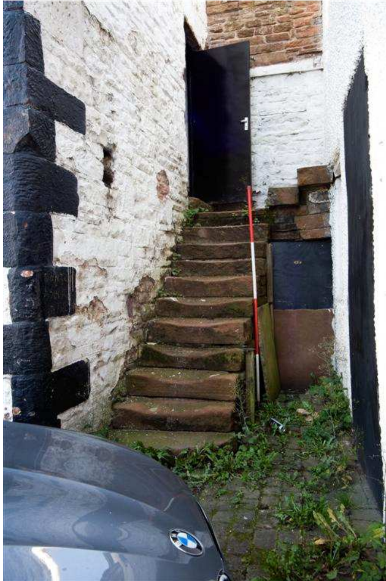
Plate 4: South elevation of the building showing the staircase
