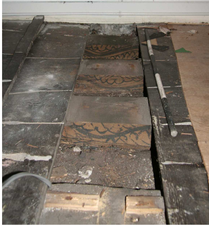
Plate 34: Decorated floor joists, Room 24
