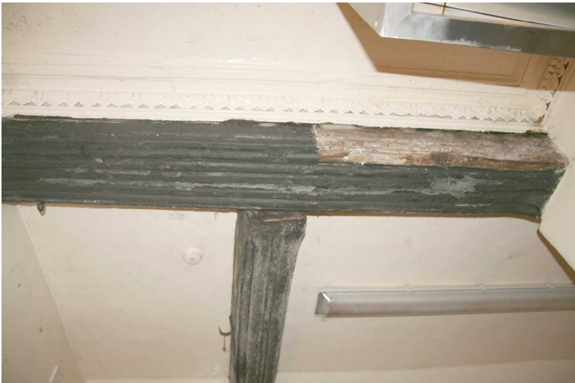
Plate 20: Detail of transverse beam, Rooms 2/4
