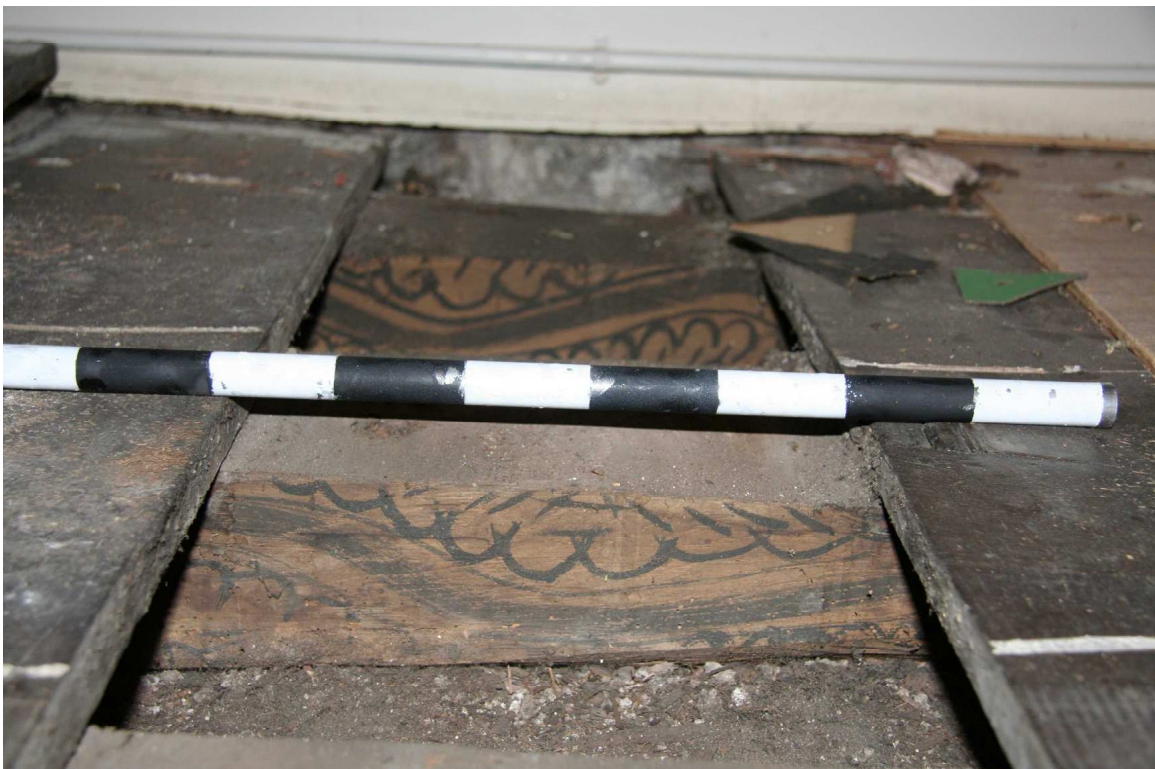
Plate 35: Detail of decoration of floor joist, Room 24
