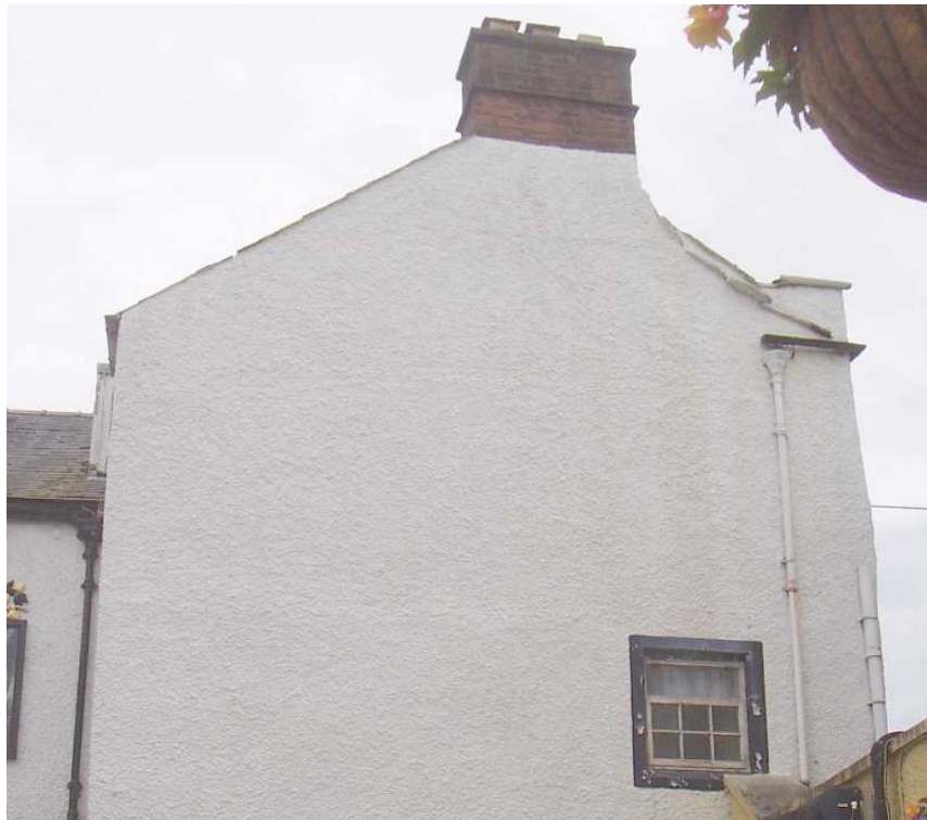
Plate 4: Detail of north gable of west range
