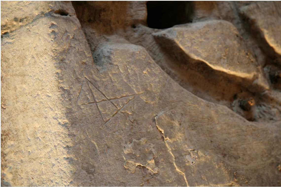
Plate 15: Detail of mason's mark
