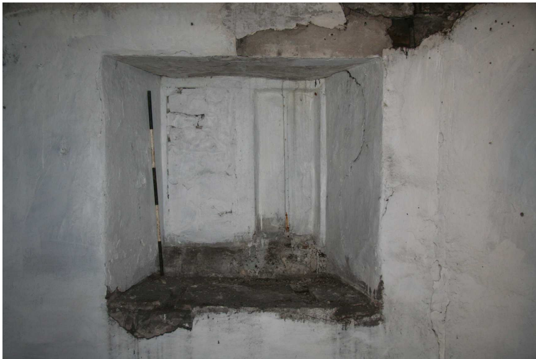
Plate 31: Blocked Phase 2 window, Room 16
