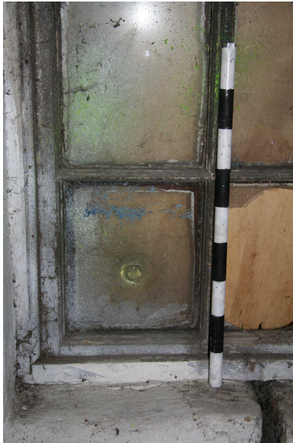
Plate 30: Horizontal, Yorkshire sash window, Room 16
