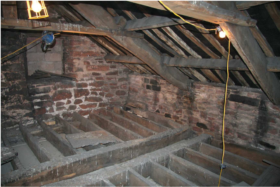
Plate 38: General view, Room 32
