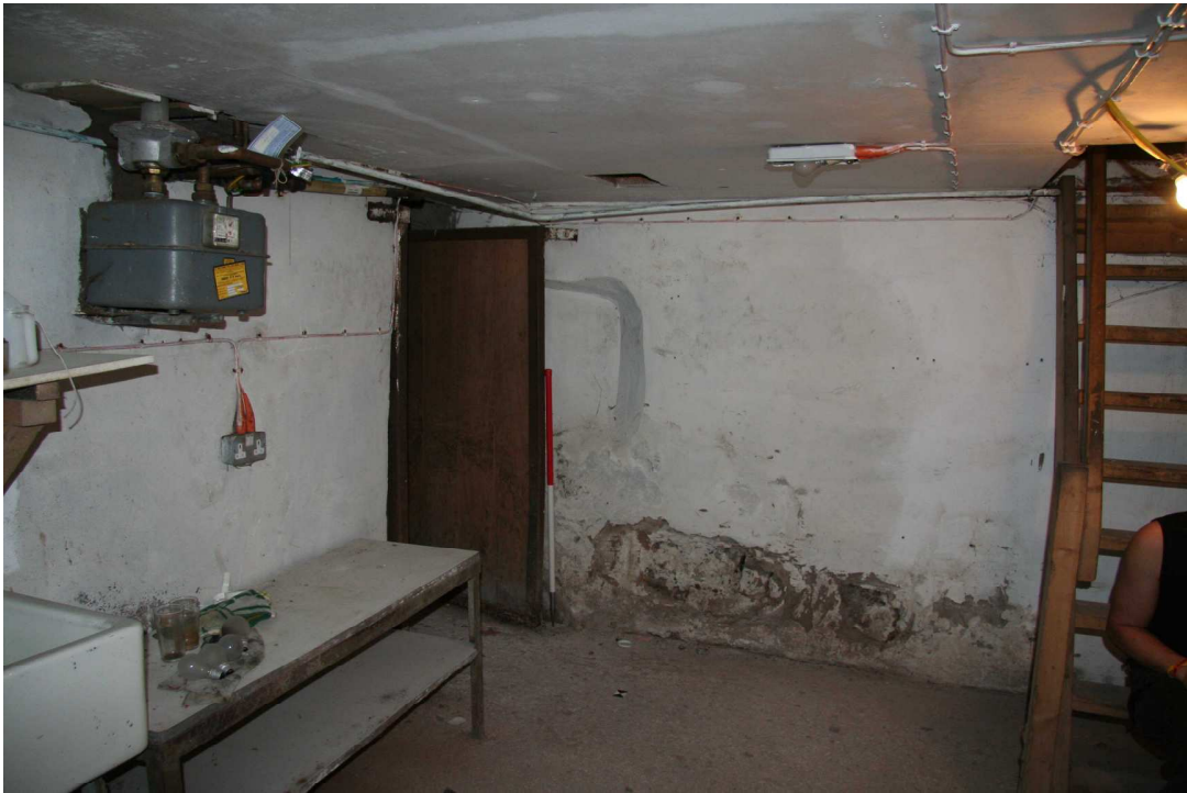
Plate 42: Recess in east elevation, Room 33
