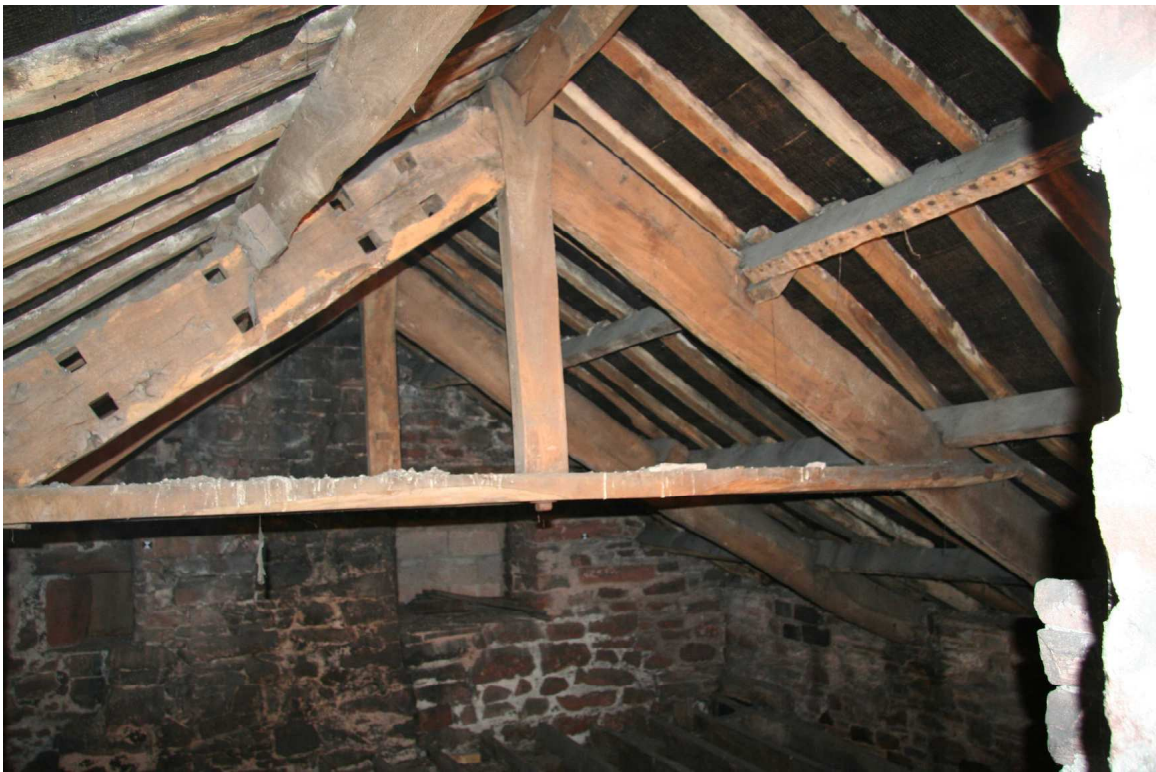
Plate 41: Western truss, Room 32
