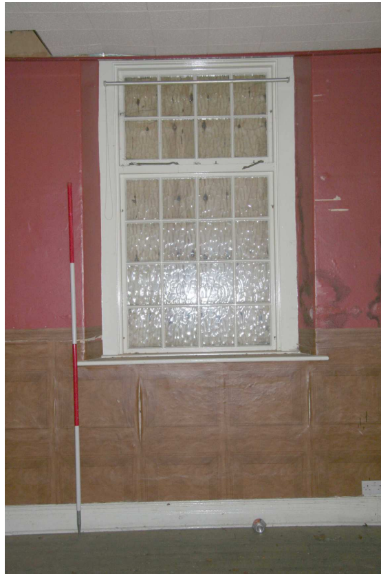
Plate 28: Window detail, Room 11
