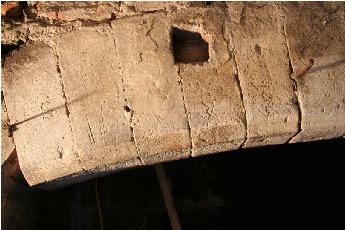
Plate 14: Mason's marks on dressed stones of inglenook fireplace, Room 1
