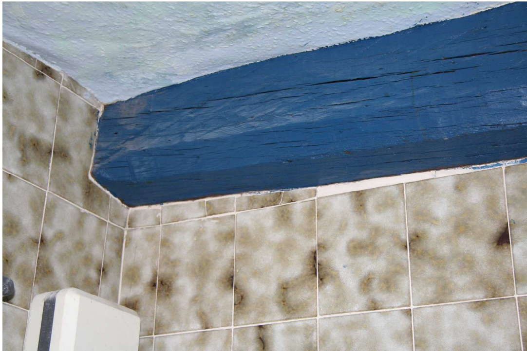
Plate 32: Detail of original first floor beam, Room 23
