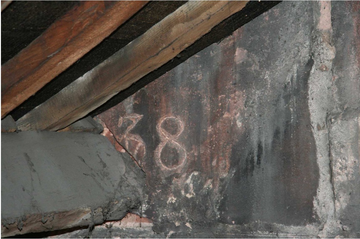
Plate 40: Datestone within western elevation, Room 32
