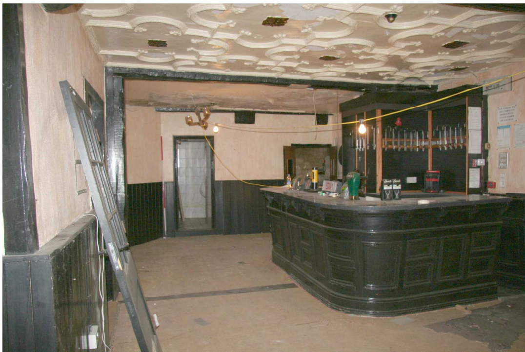
Plate 27: General view, Room 6
