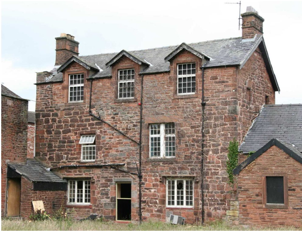
Plate 11: West external elevation
