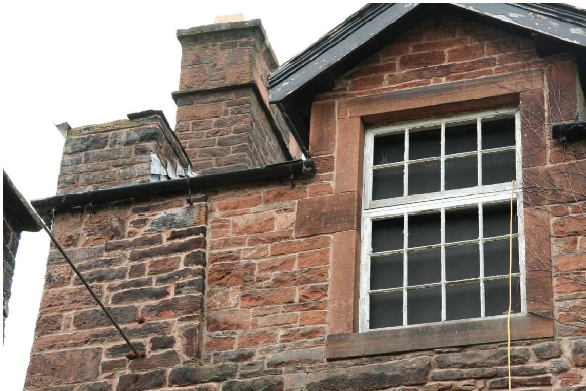
Plate 12: Detail of raised roof height, west external elevation
