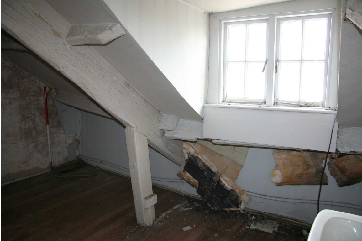
Plate 36: General view, Room 30
