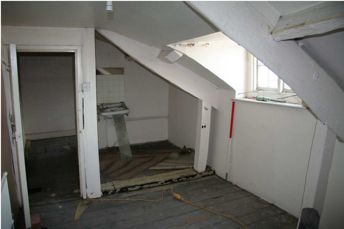
Plate 37: General view, Room 31
