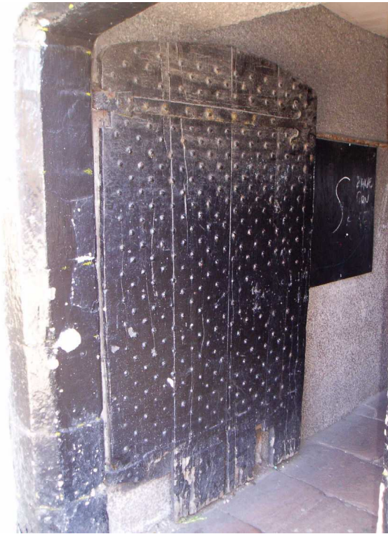
Plate 5: Detail of Phase 3 studded door
