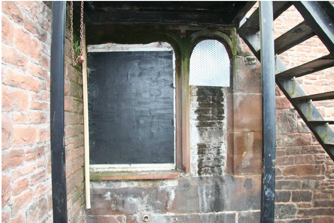
Plate 21: Detail of window mouldings, Room 4
