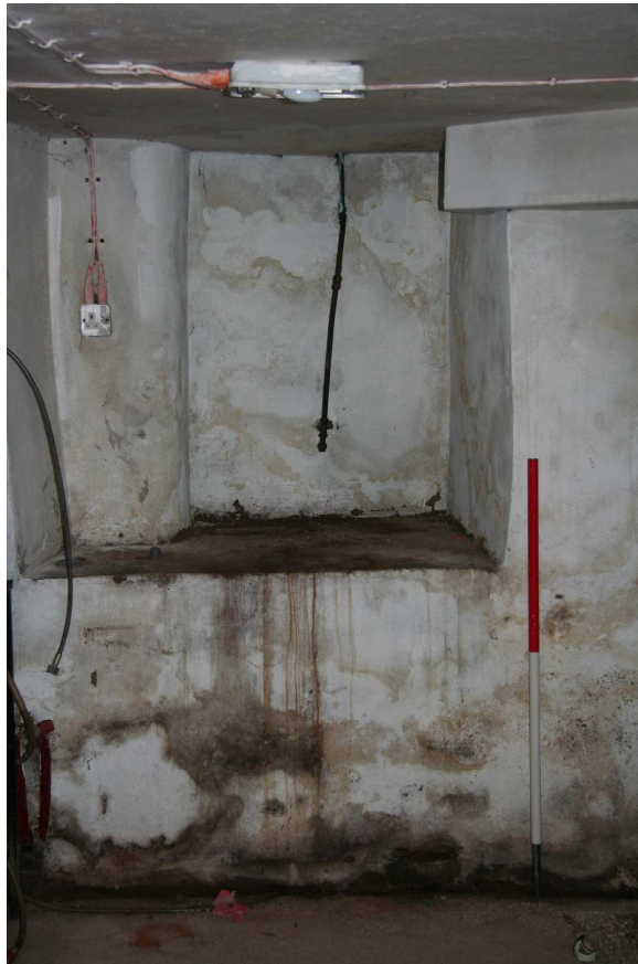
Plate 43: Window detail, west elevation, Room 33
