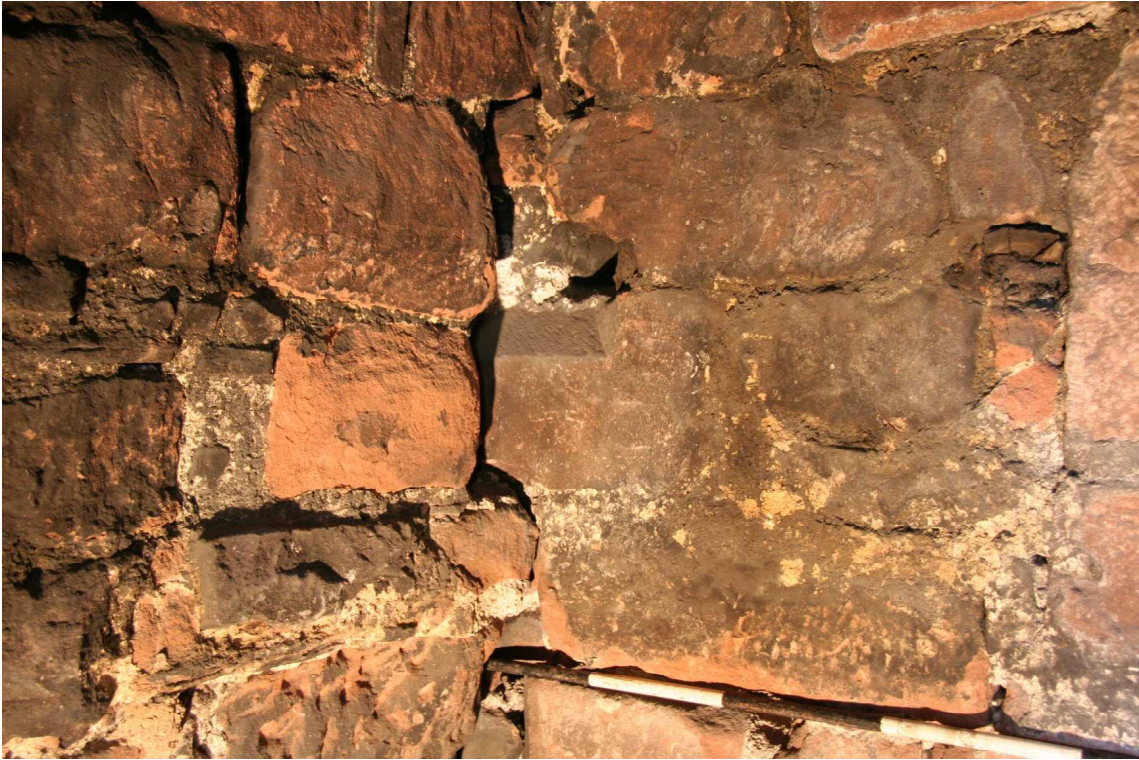
Plate 17: Re-used window surround within fire-back, Room 1
