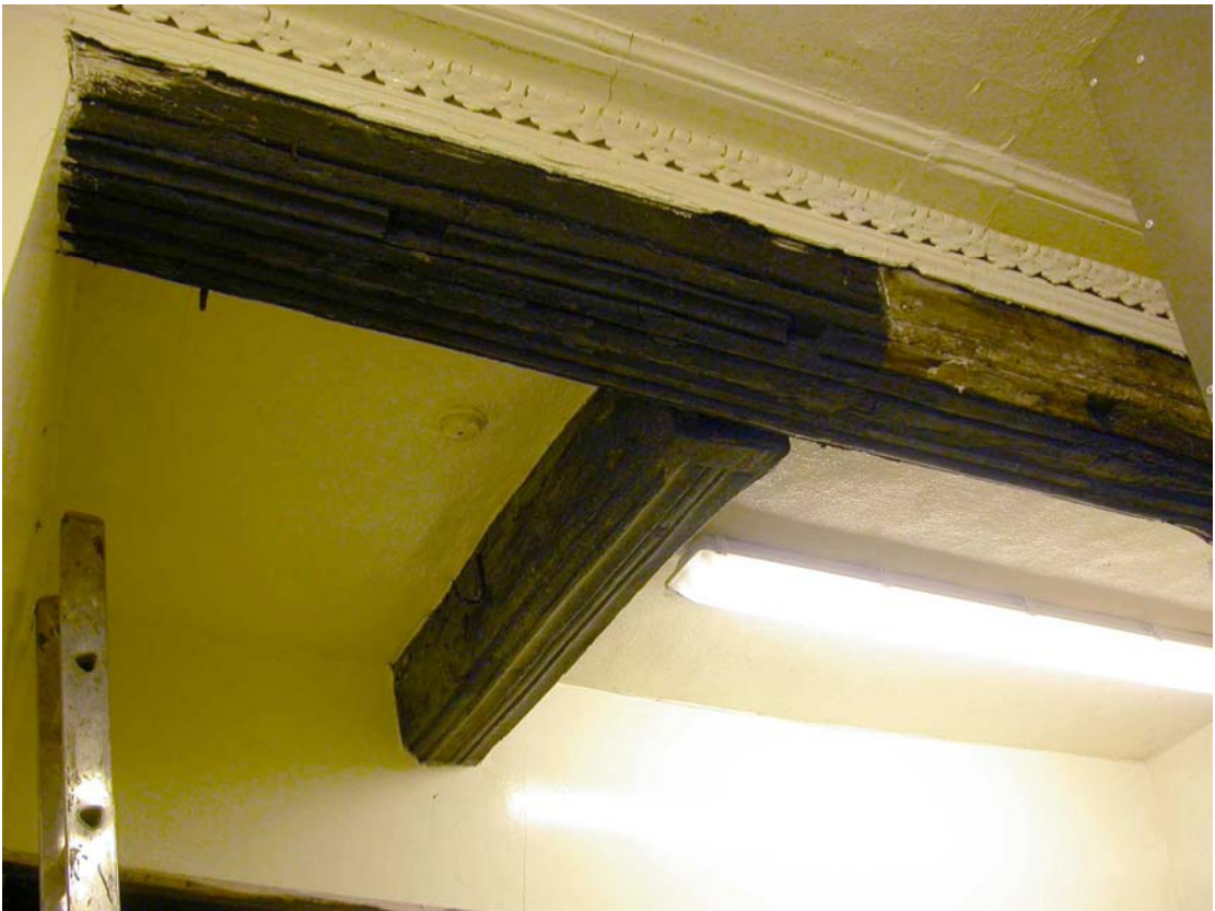
Plate 4: Original beams and position of original six-light window, Room 2
