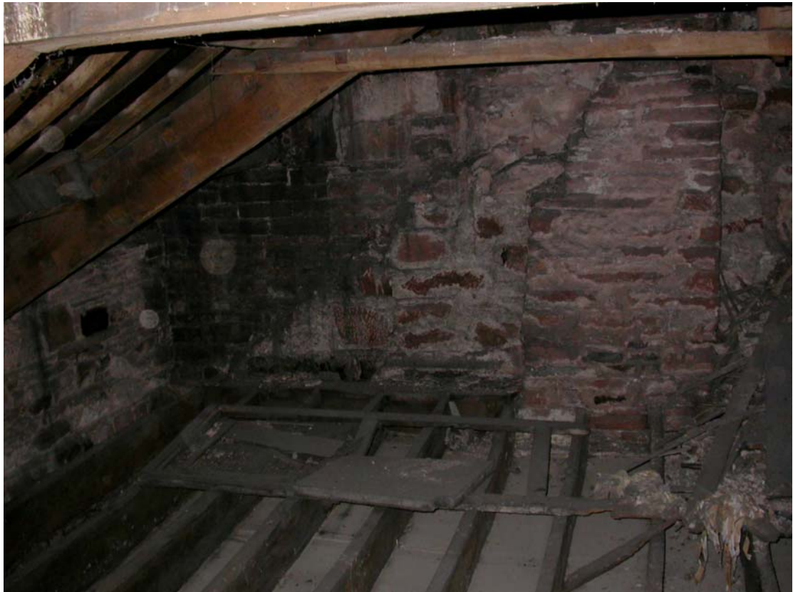
Plate 6: Chimney breast and roof scar, west elevation, Room 32
