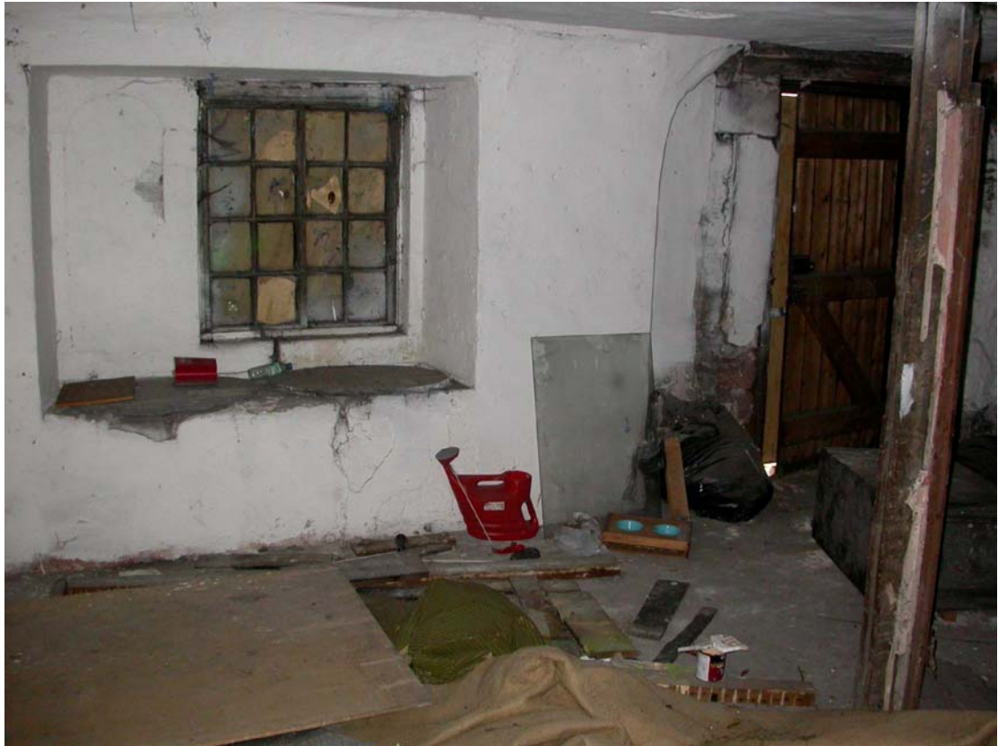
Plate 5: Partially blocked window and door arch, north elevation, Room 16
