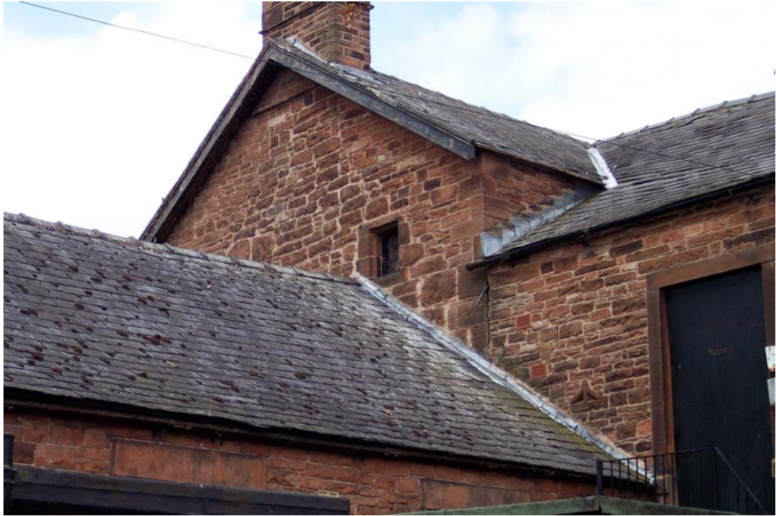
Plate 1: South external elevation gable end of late medieval hall, showing roof scar
