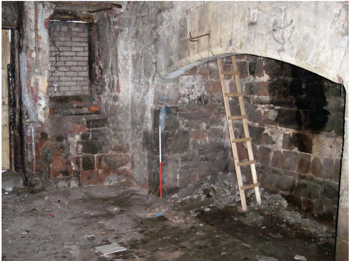
Plate 8: The original large inglenook fireplace on the east elevation in Room 1
