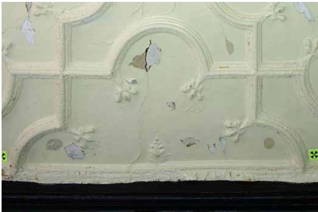
Plate 12: Example of moulded motif on one of the long edges of the ceiling
