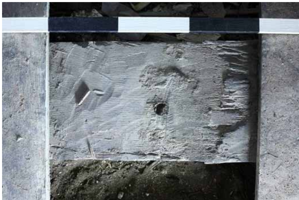
Plate 16: Example of adze marks on the upper face of Joist 11
