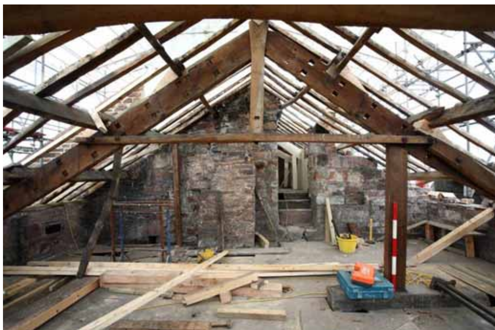
Plate 30: East roof section showing the truss construction
