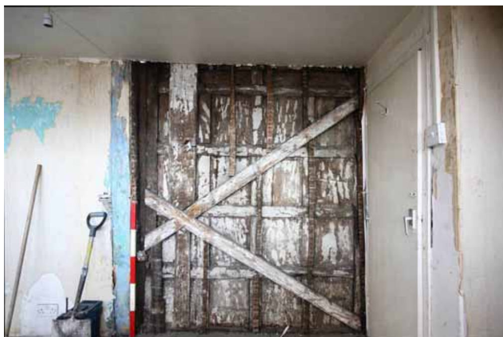
Plate 25: Timber panelling revealed in the wall between Rooms 30 and 31
