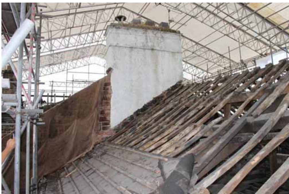
Plate 28: View of the step down on between the central and east roof sections
