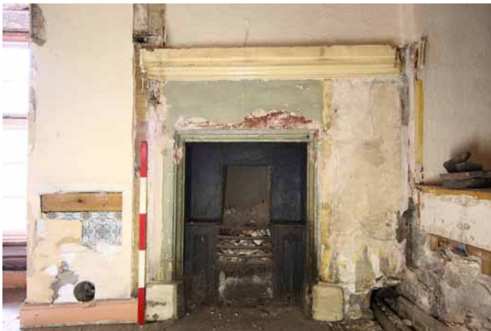
Plate 17: Fireplace revealed following stripping of Room 20
