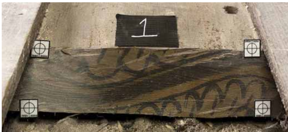
Plate 14: Example of a decorated joist below the floorboards in Room 24
