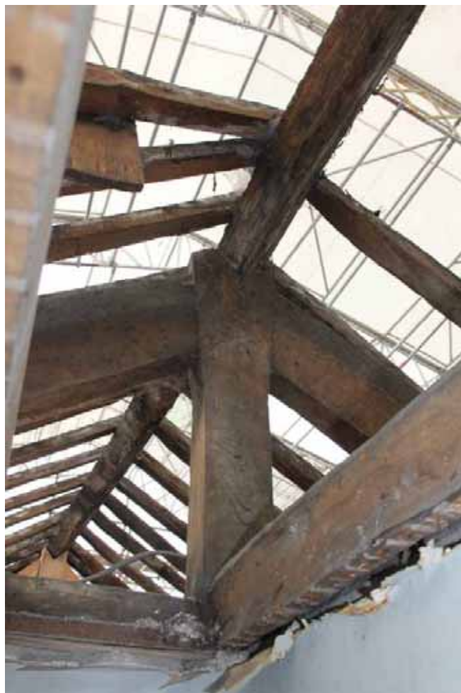
Plate 23: Visible king post above Rooms 30 and 31
