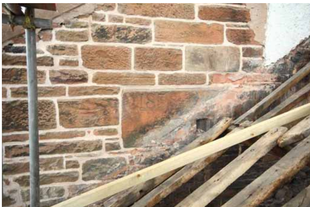
Plate 29: Inscribed date of 1838 in the east-facing gable of the central roof section
