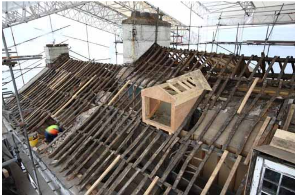
Plate 22: General view of the central and eastern roof sections
