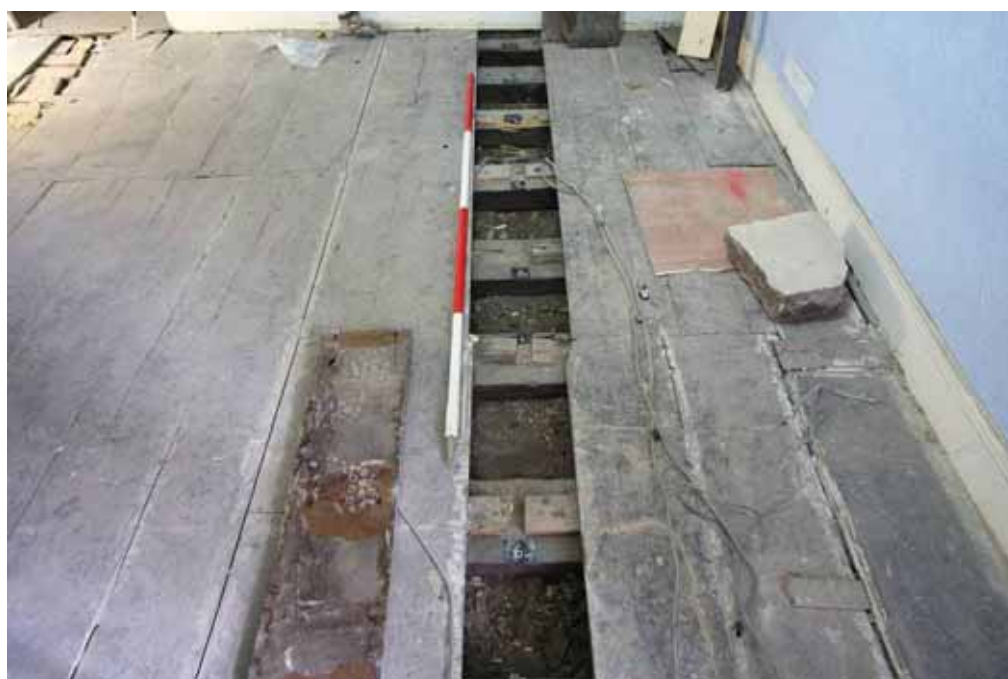
Plate 13: Removal of a floorboard revealed several decorated joists
