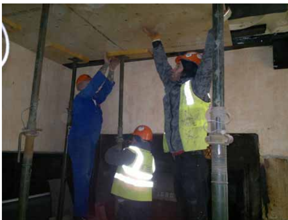
Plate 5: Removal of the protective covering on the plaster ceiling
