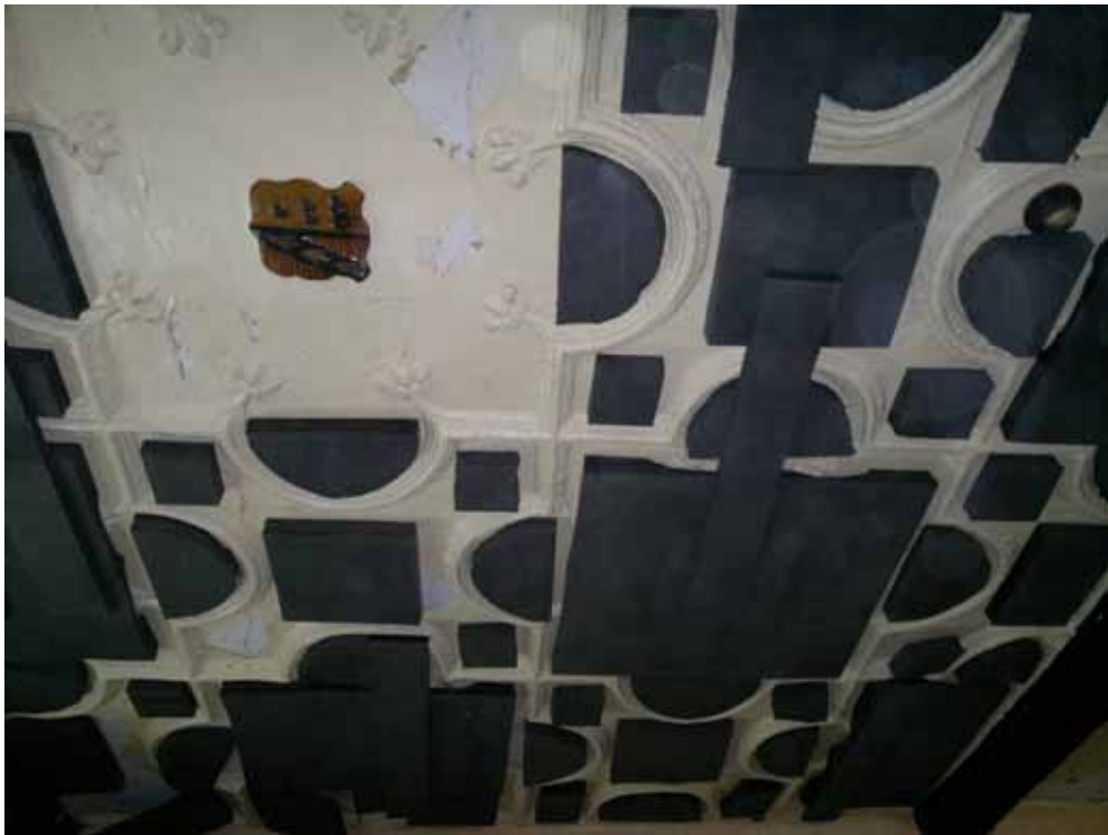
Plate 6: Protective foam in situ
