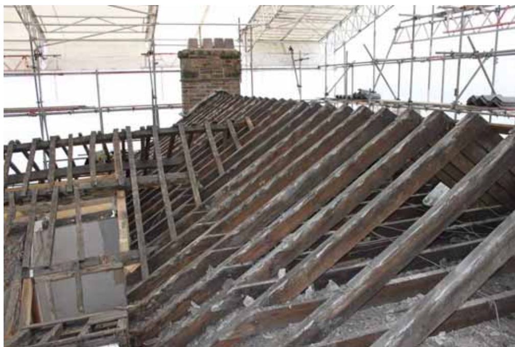
Plate 18: View of the western section of the roof, facing south
