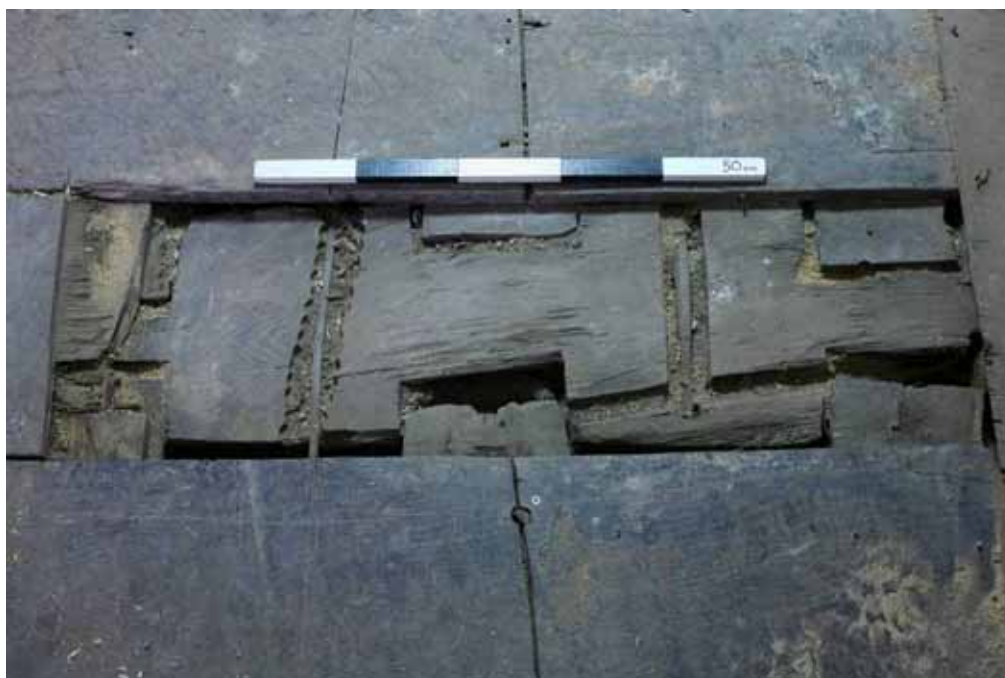
Plate 15: Central beam showing the ends of the decorated joists
