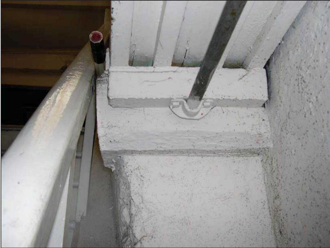
Plate 19: Original Floor Beam in Staircase
