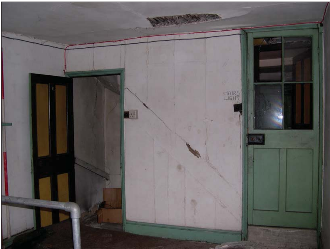
Plate 26: Doors in Room 7 North
