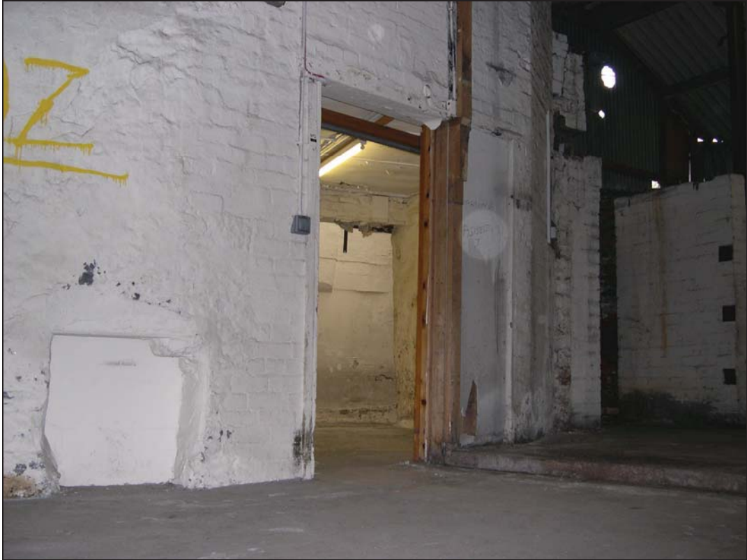
Plate 15: Fireplace and Doorway Room 2
