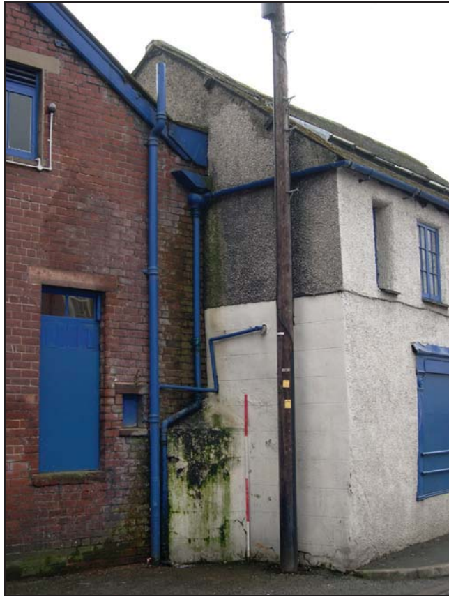
Plate 9: East Elevation of No. 9
