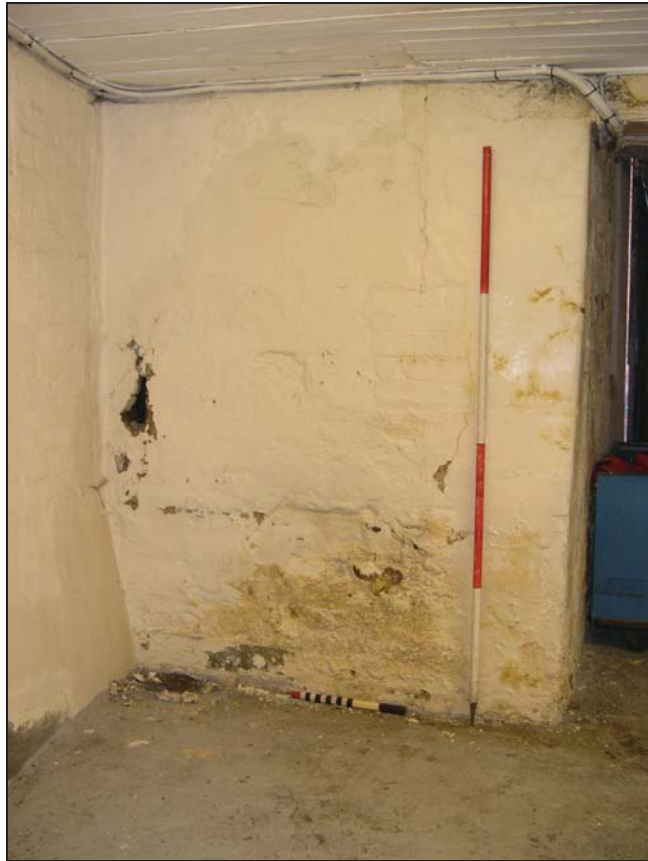
Plate 21: Blocked Fireplace in Room 4
