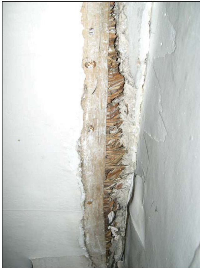
Plate 28: Reed Plaster in Room 7 South
