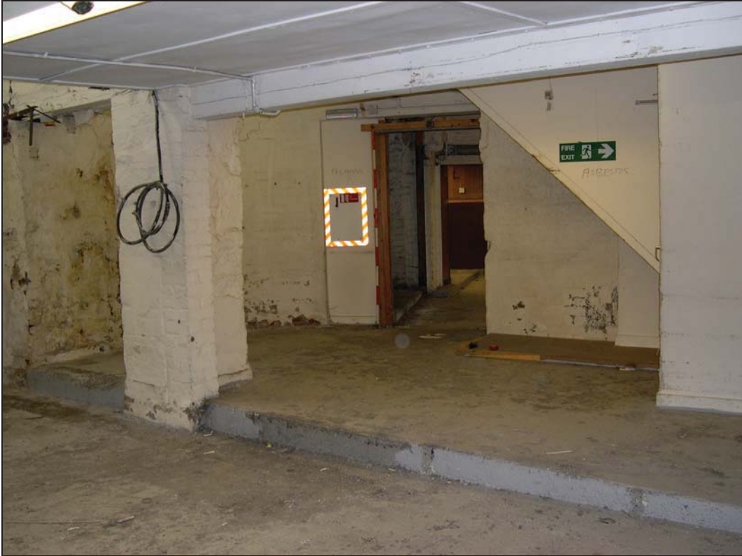
Plate 17: Room 3 facing west
