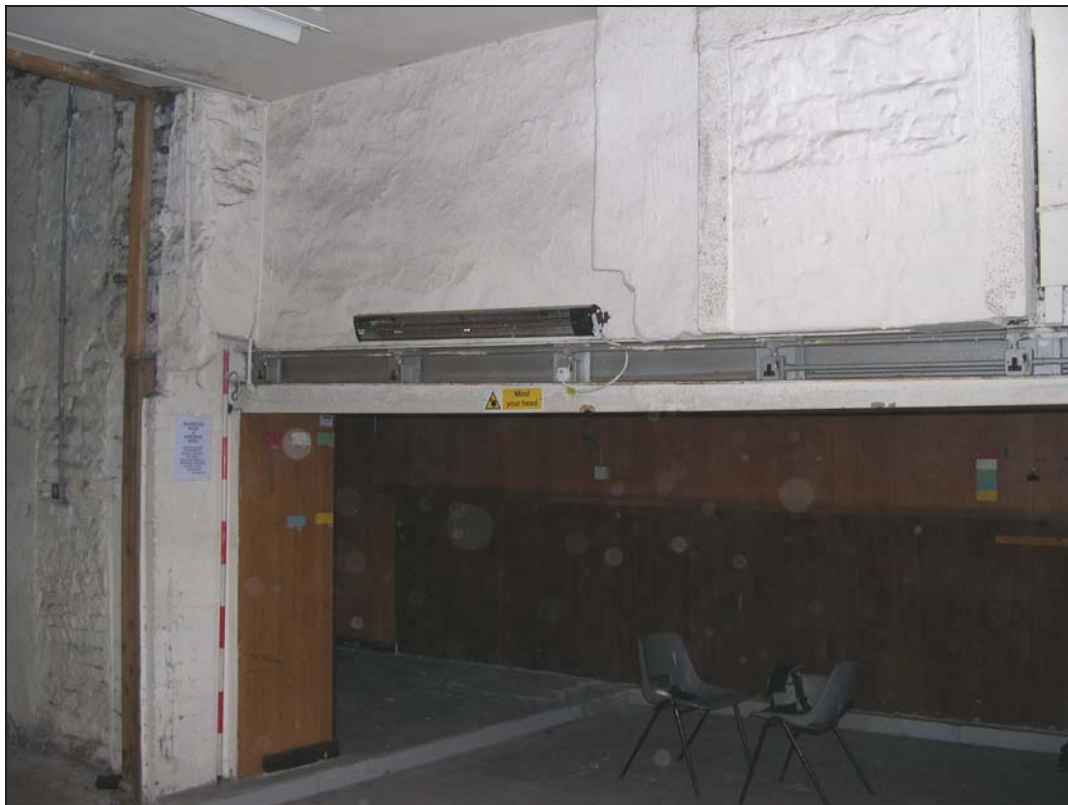
Plate 14: Fireplace and Original Floor Level Room 2
