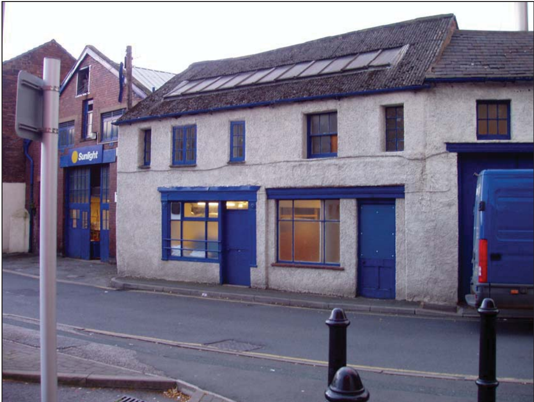
Plate 7: Elevation of Nos. 9 and 10 Prior to Boarding
