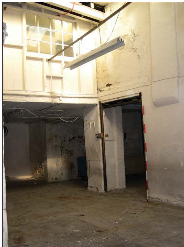
Plate 20: Room 4 Facing North
