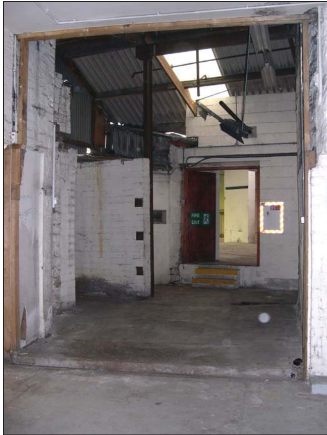
Plate 13: Rear of Room 1
