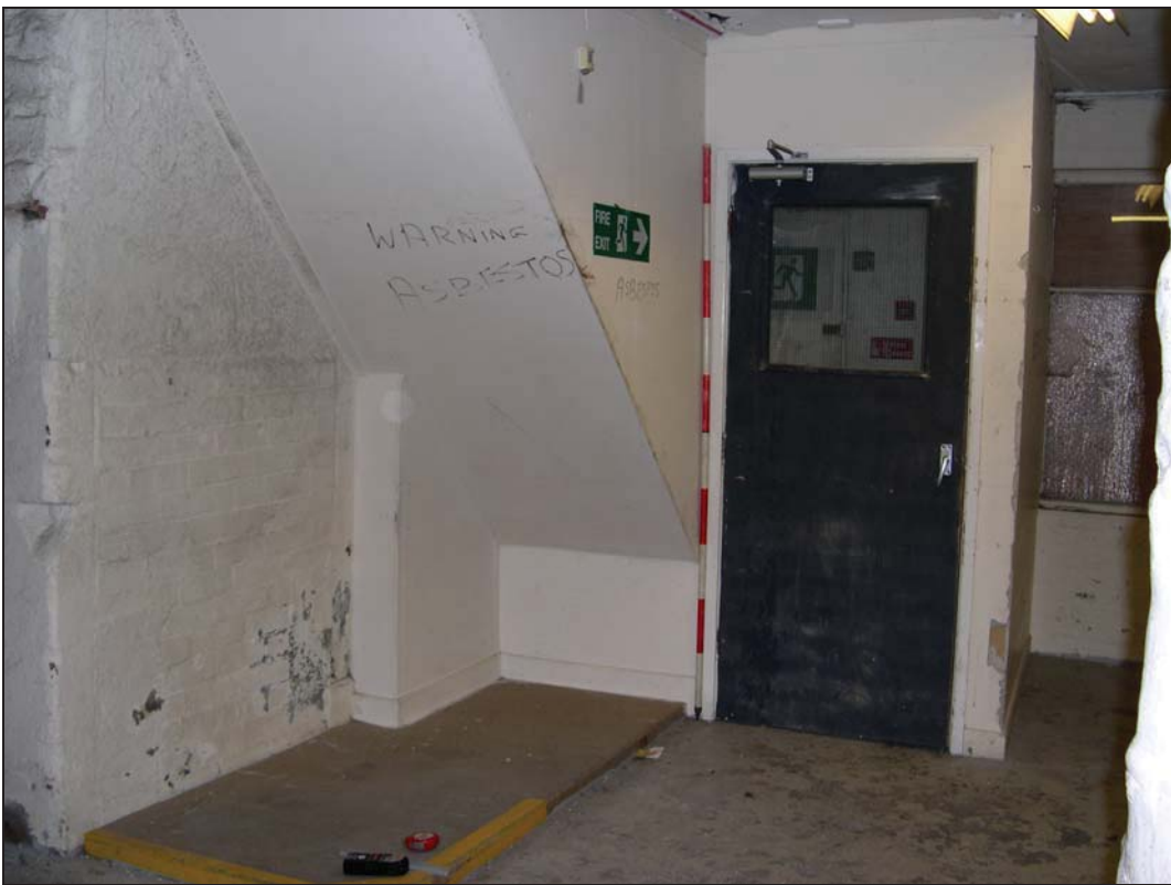
Plate 18 Room 3 Facing North
