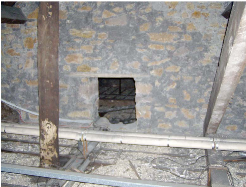
Plate 26: Aperture between roof spaces, facing east
