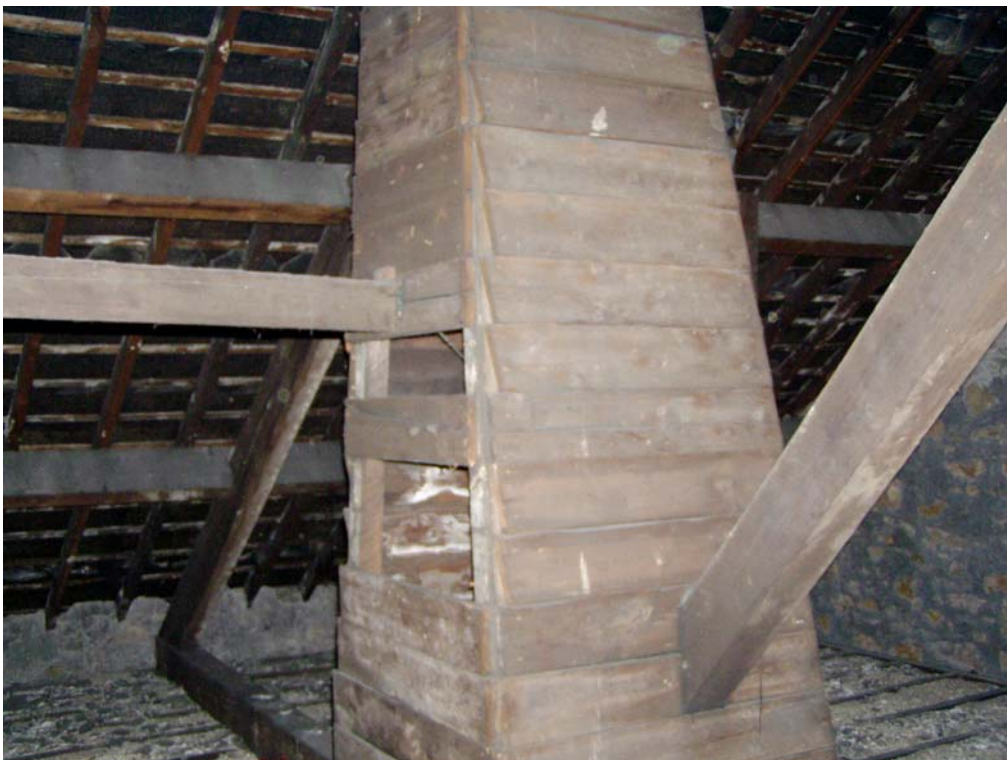
Plate 30: Boxed in king-post in east/west roof space
