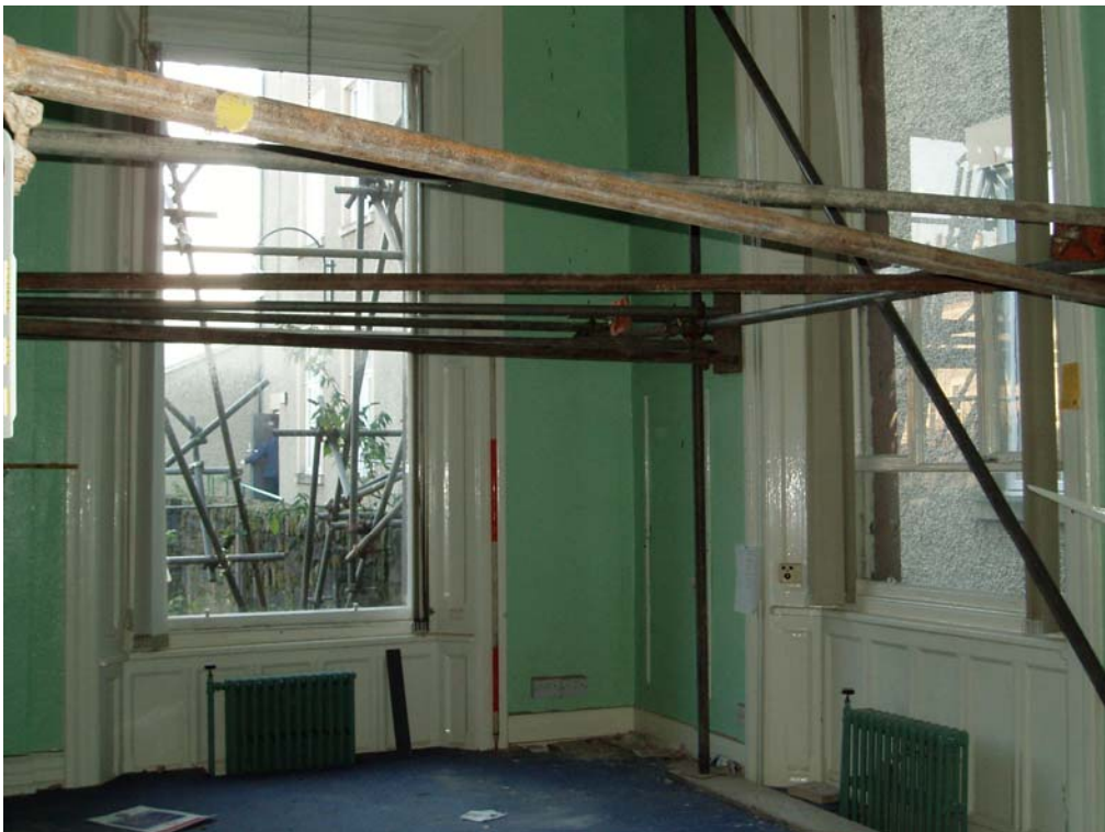
Plate 22: Room 9, facing south-east
