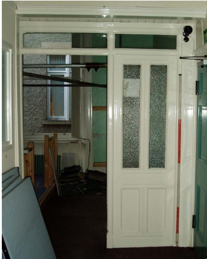
Plate 19: The doorway between Rooms 8 and 9, facing south
