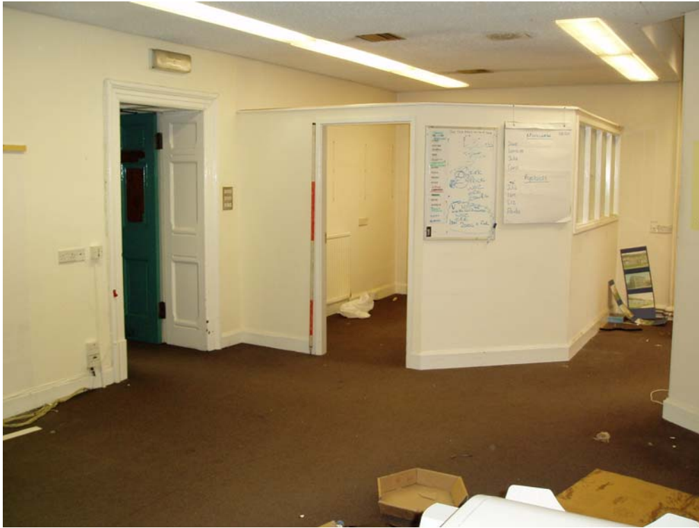
Plate 13: Room 3, facing south
