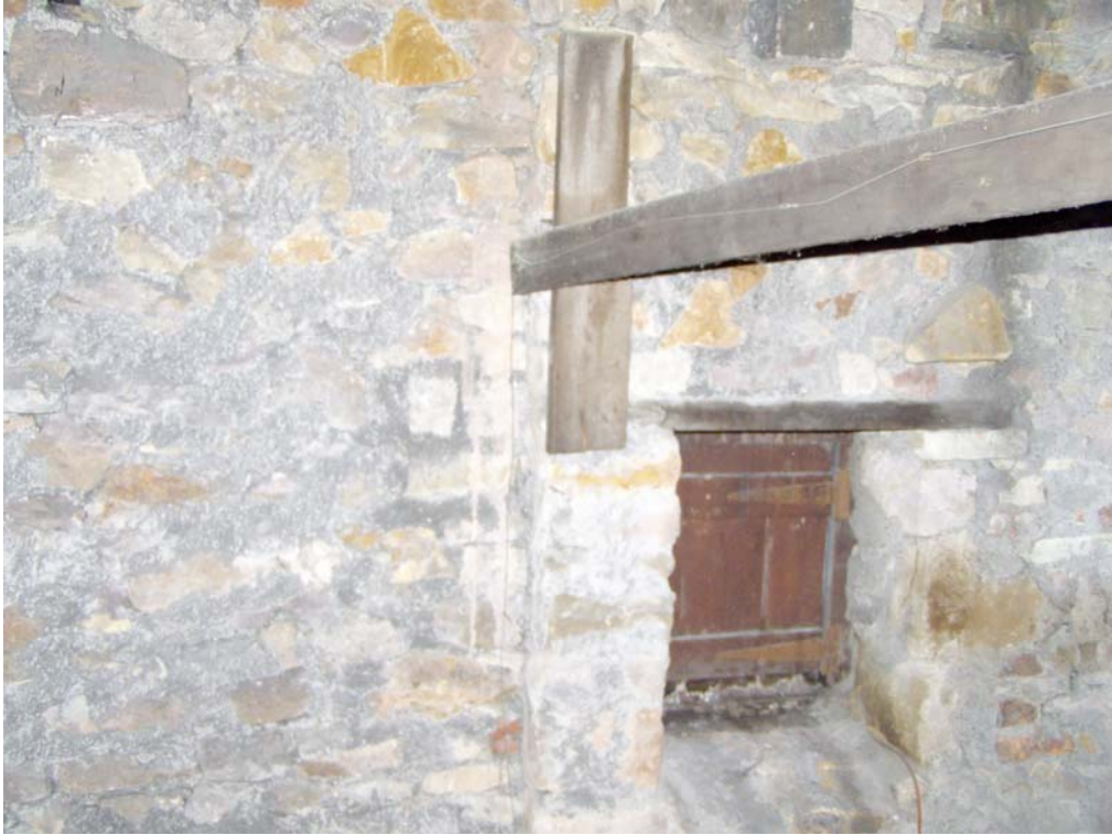
Plate 31: Hatch in east elevation of roof space
