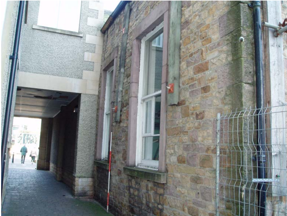
Plate 7: The south elevation
