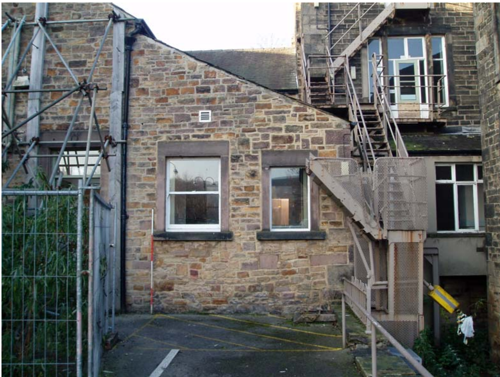
Plate 6: The outshut (rear) elevation
