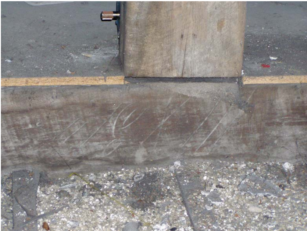
Plate 28: Baltic timber marks of southern truss, facing south
