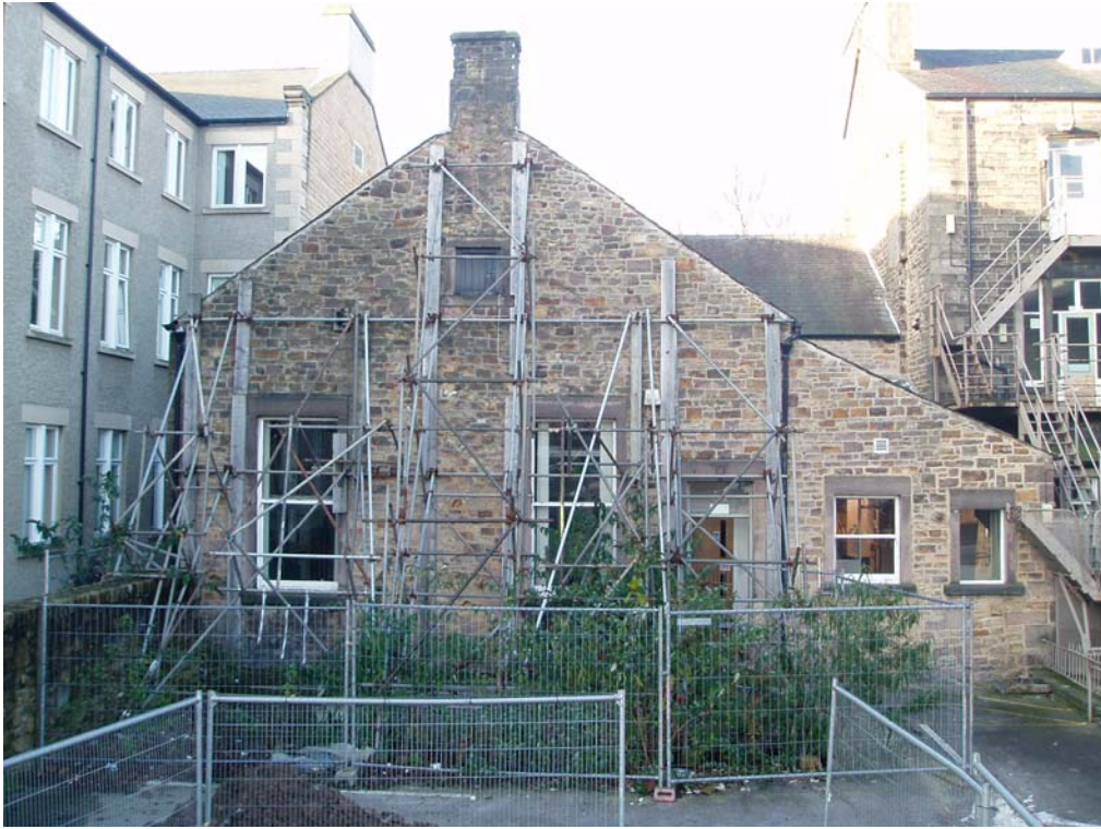
Plate 5: The rear (east) elevation
