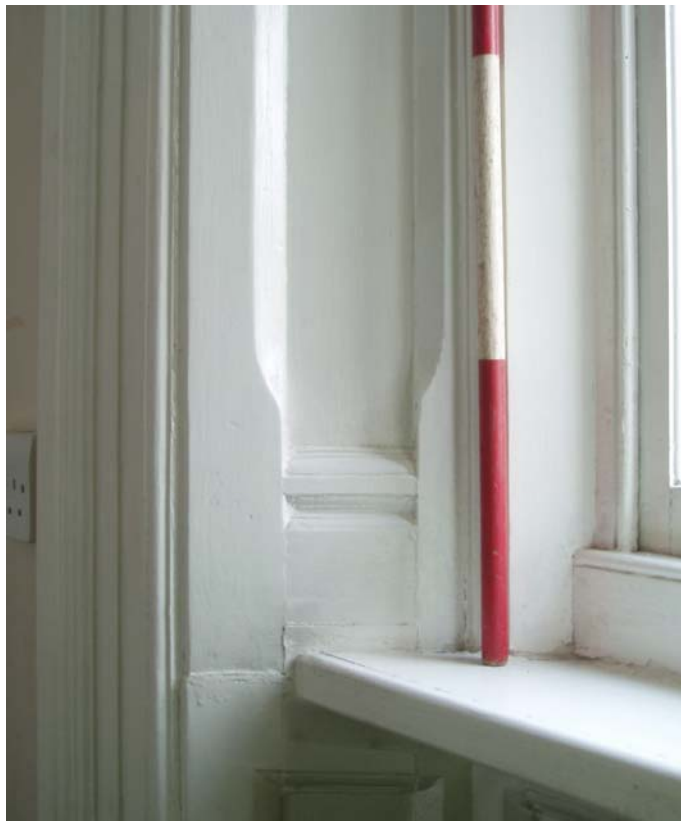
Plate 12: Chamfer detail on window reveal
