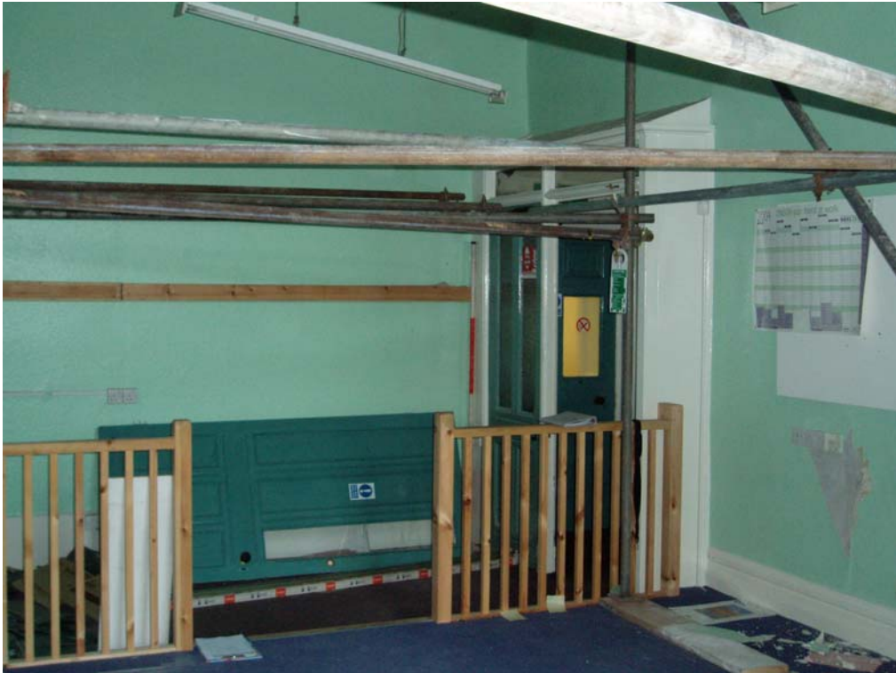
Plate 23: Room 9, facing north-west
