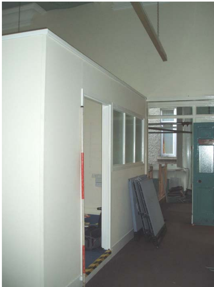
Plate 18: Room 8, facing south
