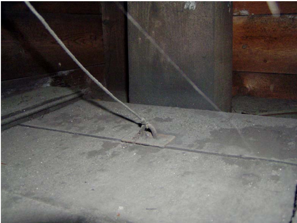
Plate 32: Flap within boxed-in king-post
