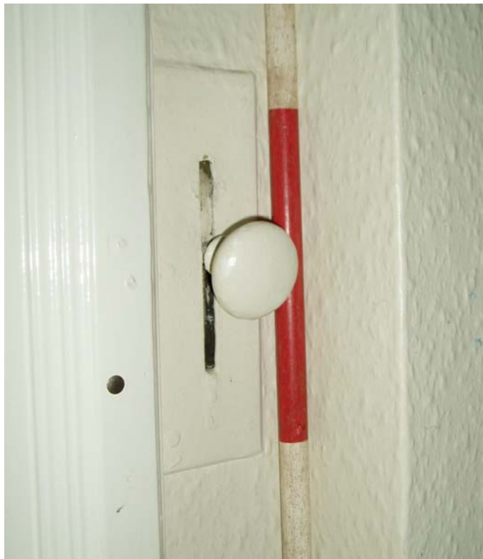
Plate 20: The knob adjacent to the window in Room 8
