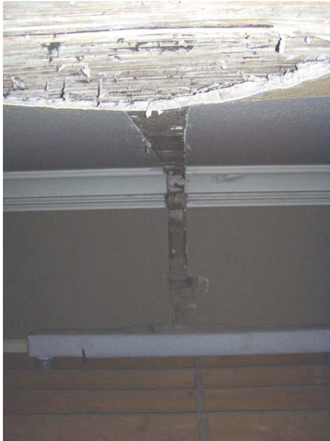
Plate 25: View above suspended ceiling, facing north
