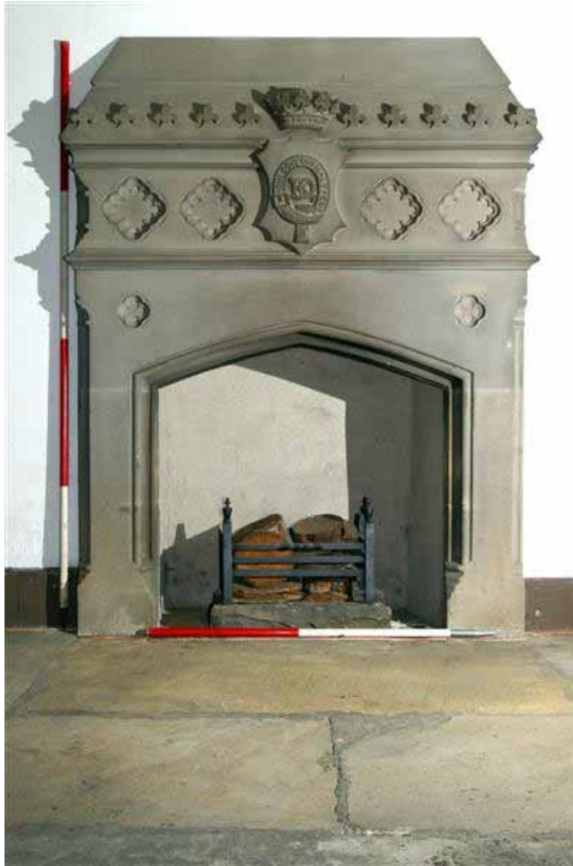
Plate 75: Fireplace in Room L109 of the Sound Archive
