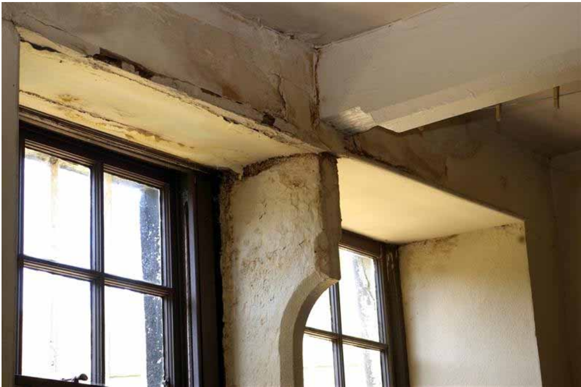
Plate 43: Beam and mullion in Room E008 illustrating cut-away section
