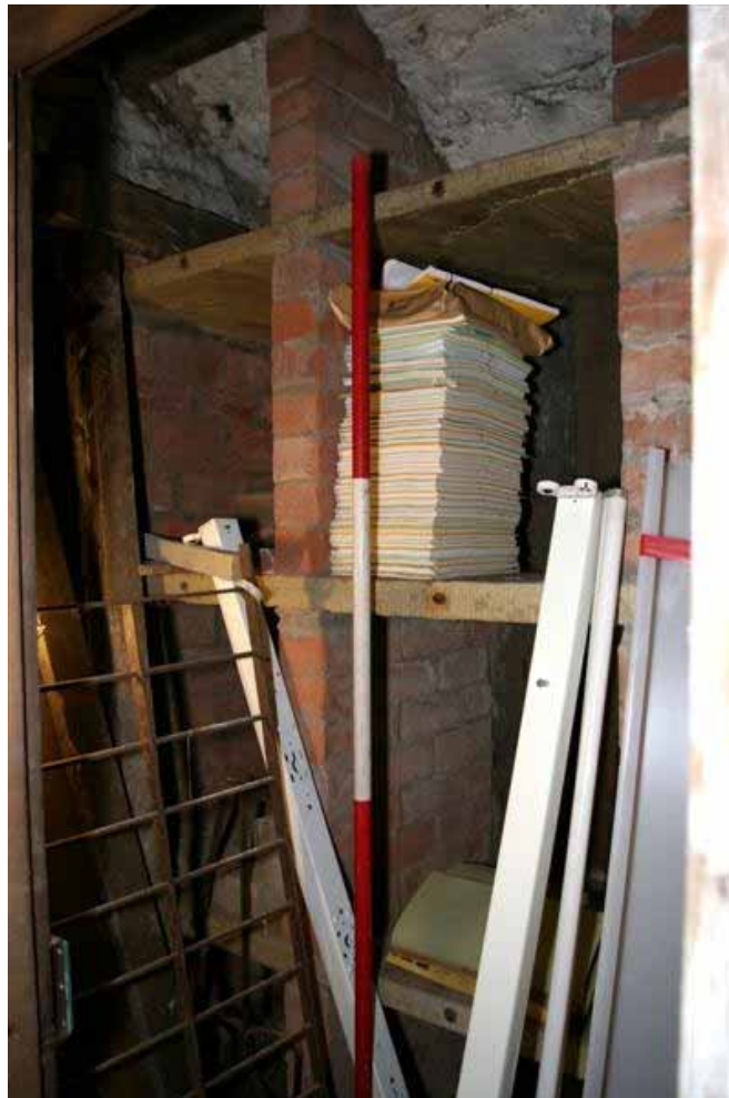
Plate 64: Shelving in the basement
