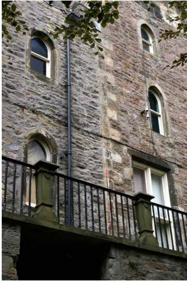
Plate 17: Quoins visible in the south-east elevation of the Museum
