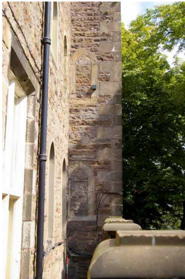
Plate 16: Blocked windows in the south face of the 'South-East Tower'
