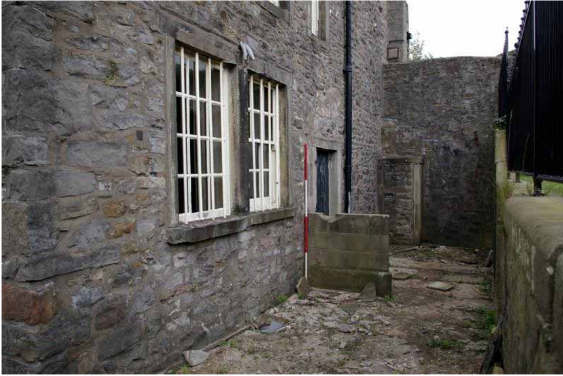
Plate 25: Walkway at the base of the Museum south-west elevation
