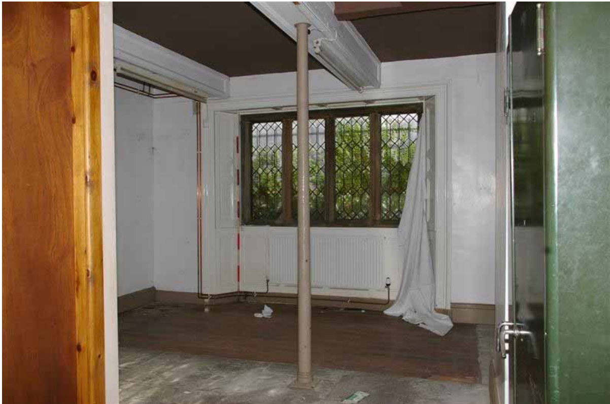
Plate 80: General view of Room L104 of the Sound Archive facing east
