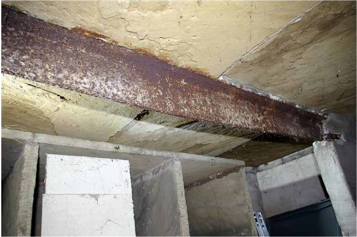
Plate 83: Cast-iron beam in Room L107 of the Sound Archive
