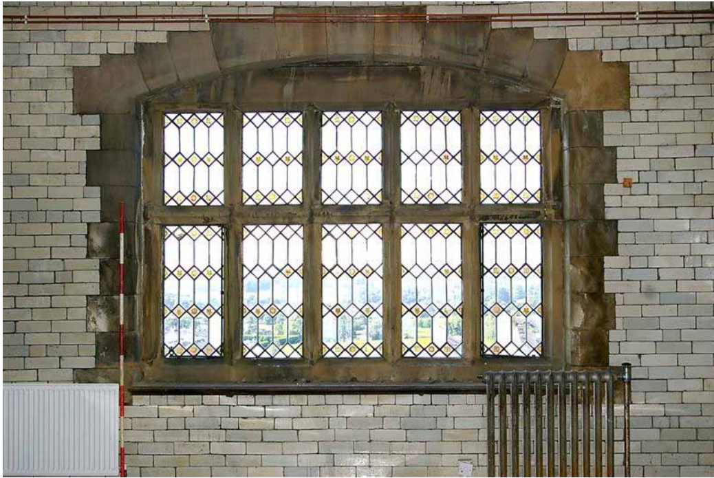
Plate 93: The west window in Room U107 of the Court House
