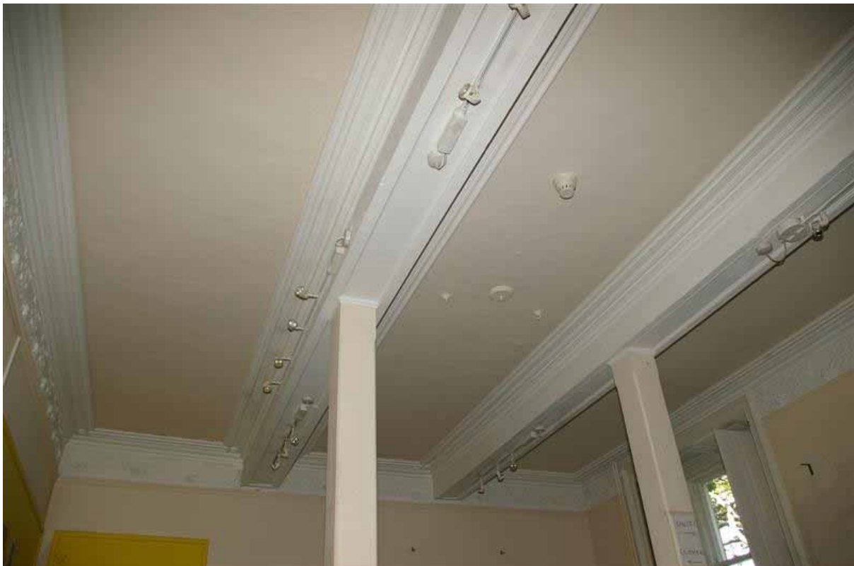
Plate 48: View of the ceiling of Room E012
