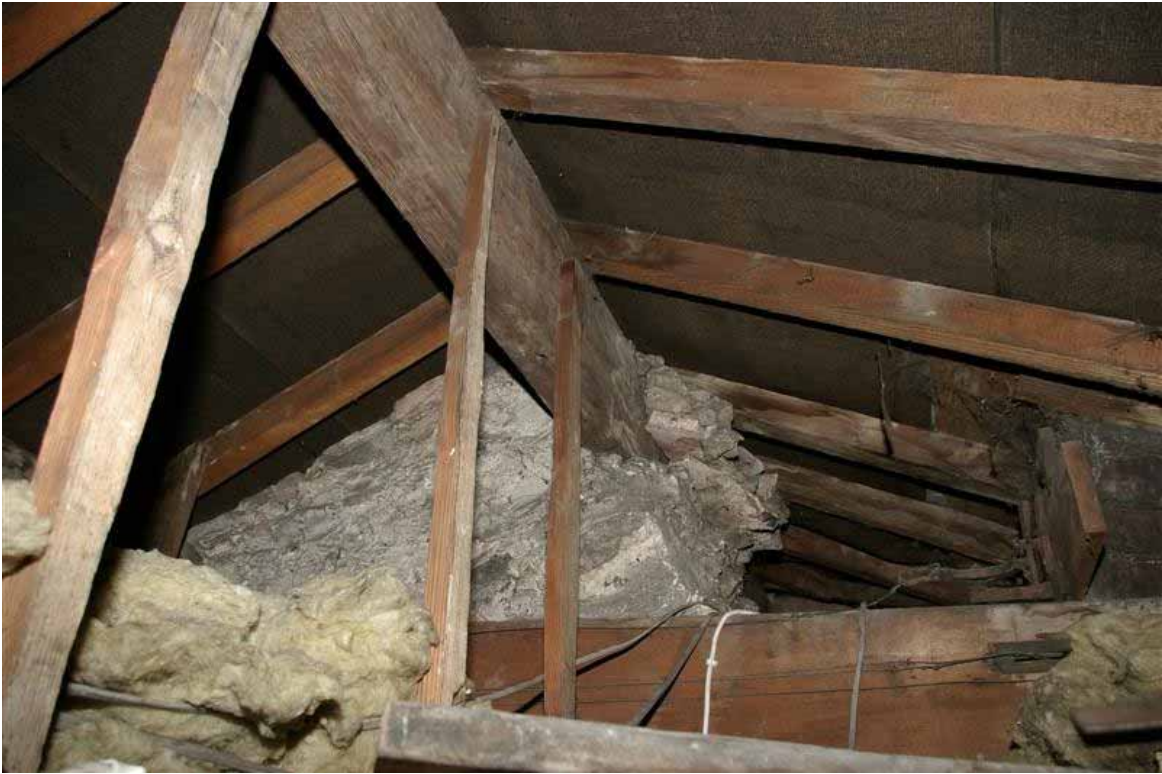
Plate 61: Roof space above Room U002
