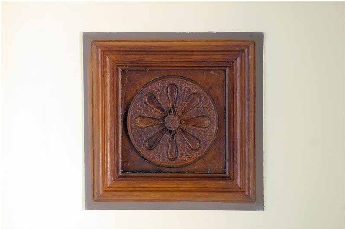
Plate 87: Ventilation opening in Room U105 of the Sound Archive
