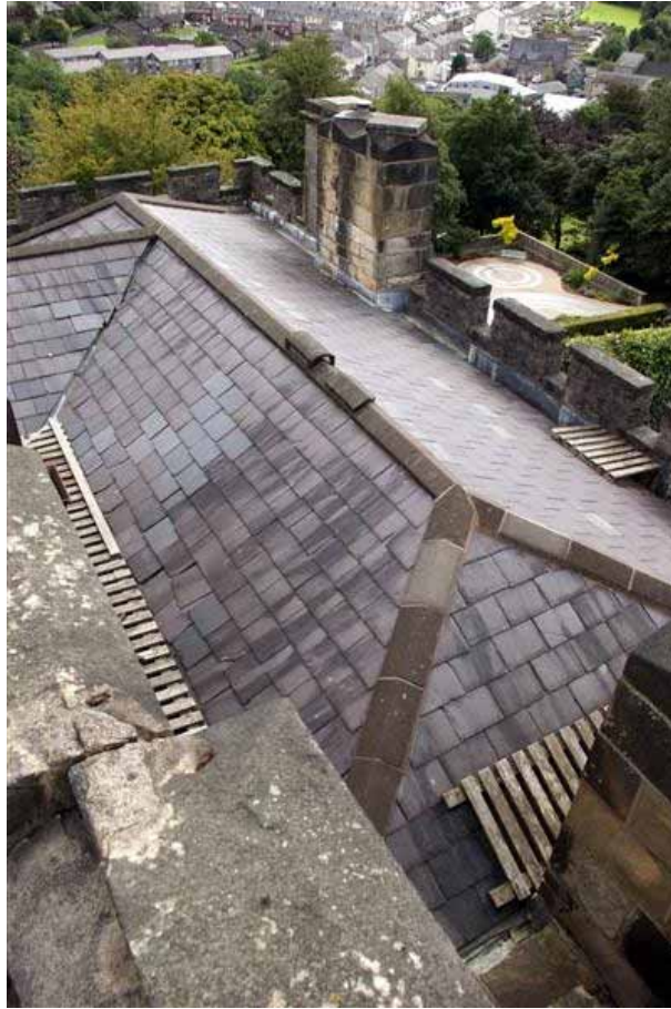
Plate 9: General view of the Museum roof looking north-east
