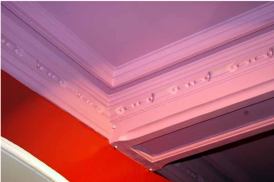
Plate 38 Detail of the decorative cornice in Room E005
