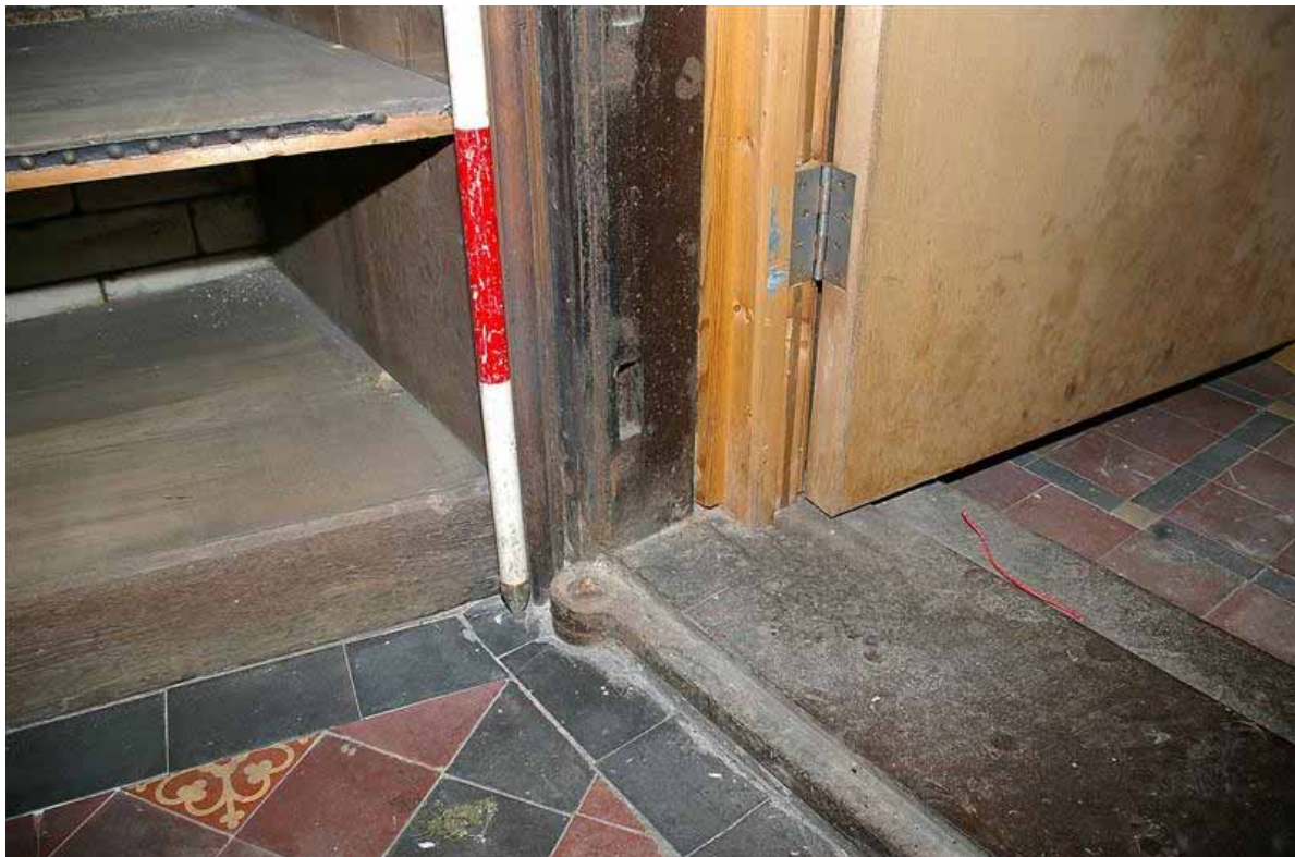
Plate 90: Iron door surround in Room U106
