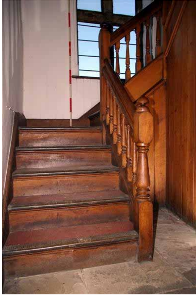
Plate 81: Oak staircase in Rooms L106/U104 of the Sound Archive
