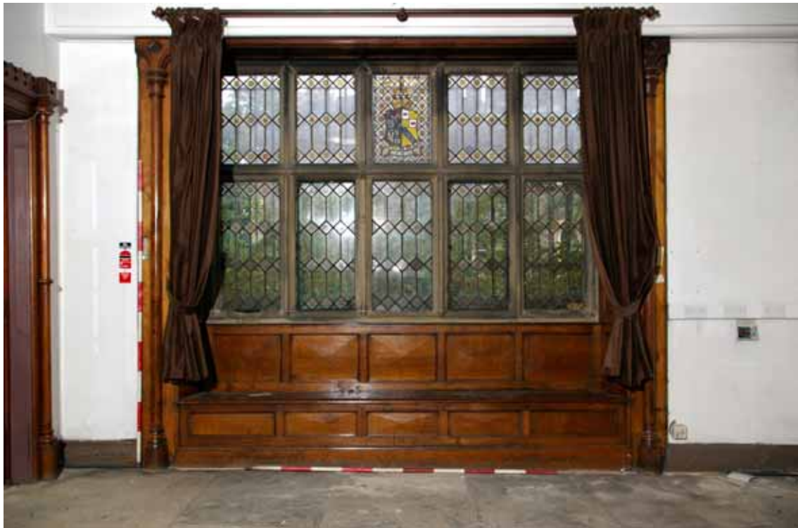
Plate 72: Window in Room L109 in the Sound Archive
