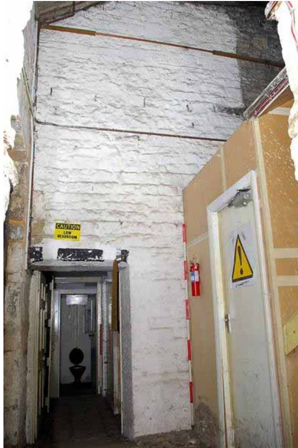
Plate 95: The north wall of the Court House from within Room L116
