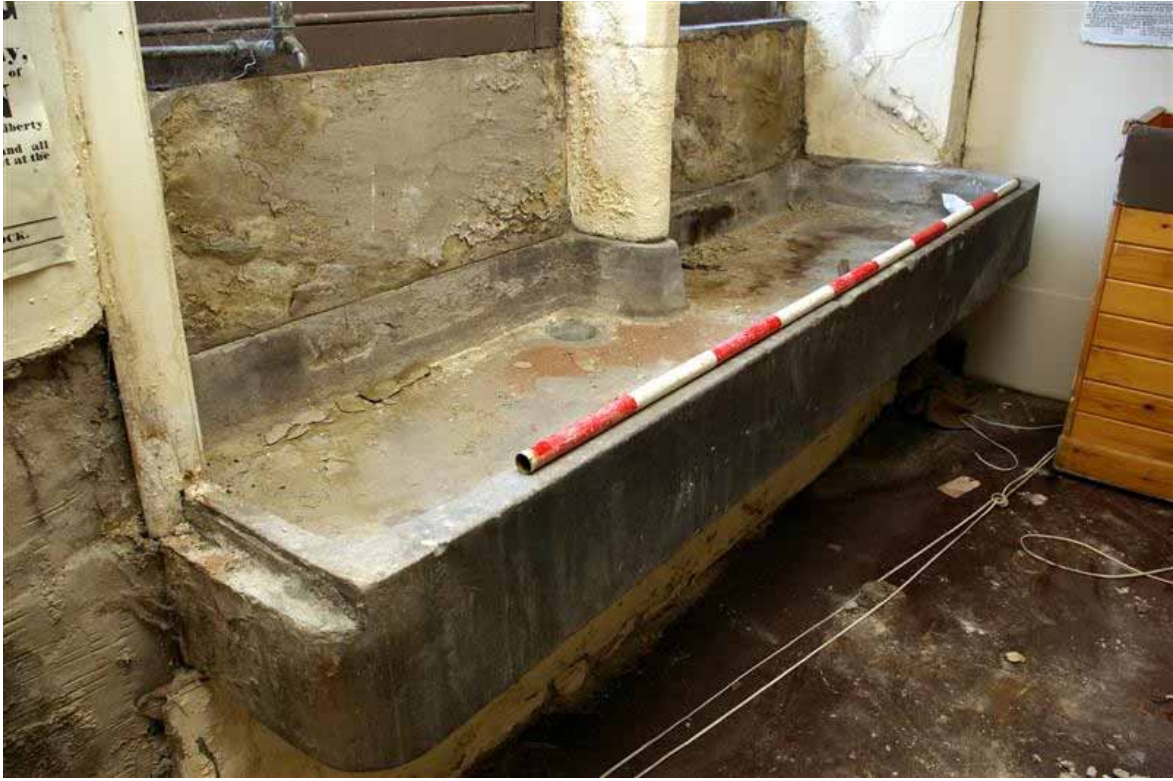
Plate 41: Stone sink in Room E008
