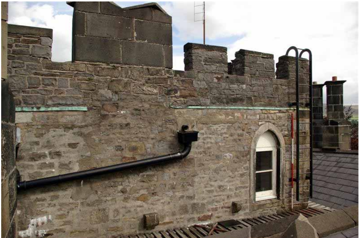
Plate 22: North-western side of the upper part of the Museum south-west elevation
