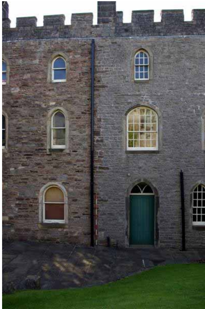
Plate 5: Difference in construction visible in the north-west elevation of the Museum
