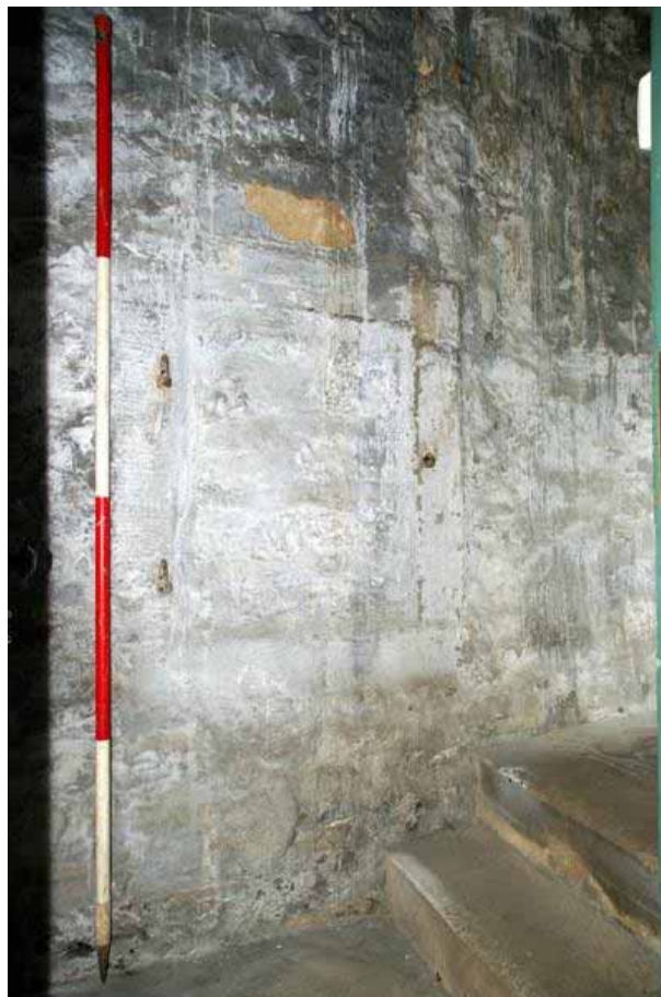
Plate 78: Blocked window in the west wall of Room L110
