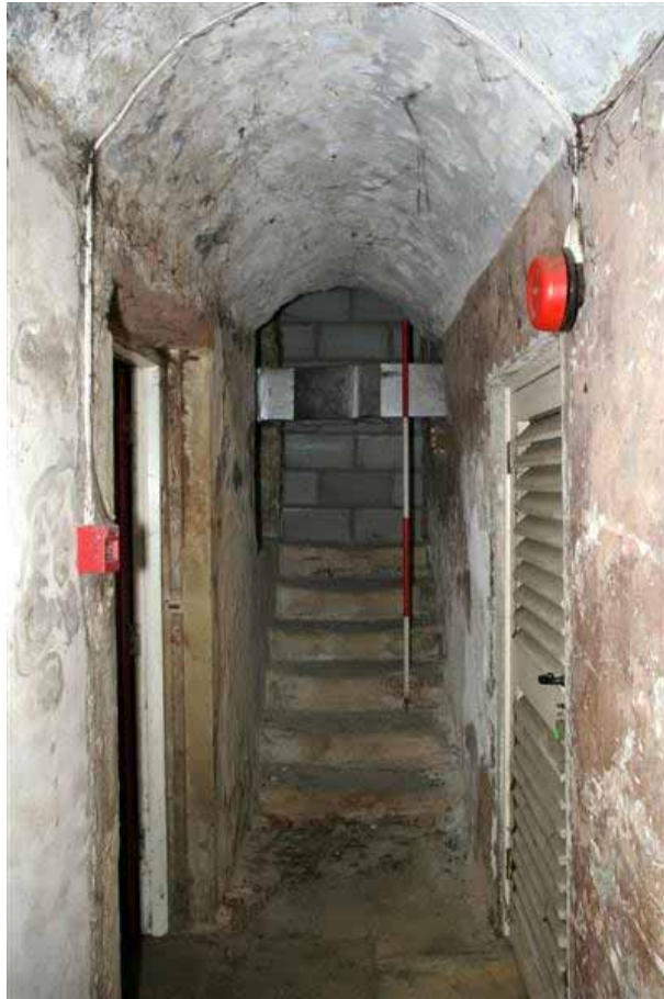
Plate 65: Steps from the basement which once led to Room E010b
