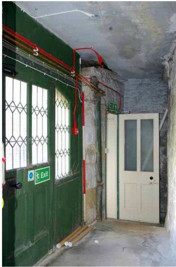
Plate 77: Room L110 facing south
