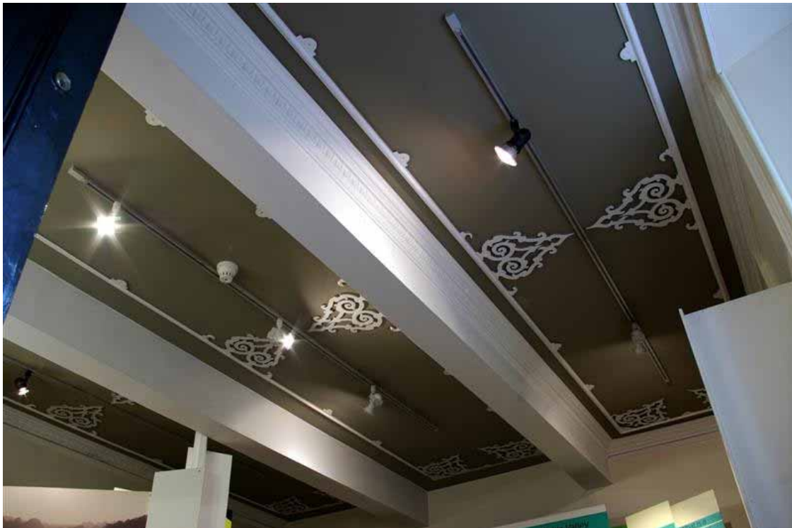
Plate 54: Decorative ceiling in Room L005
