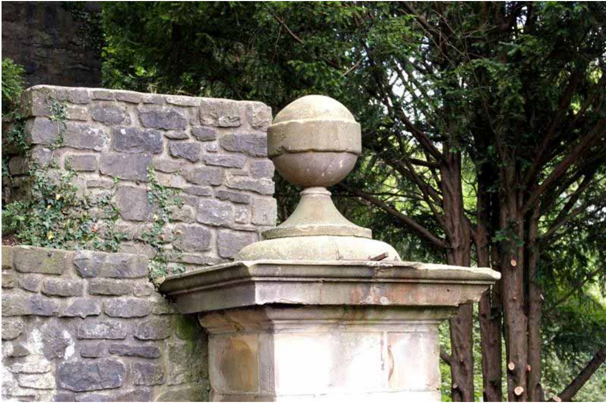
Plate 101: Detail of the top of the posts
