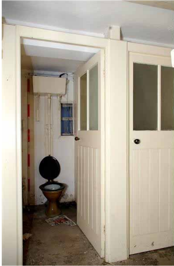
Plate 97: Toilets in Room L112 of the Court House
