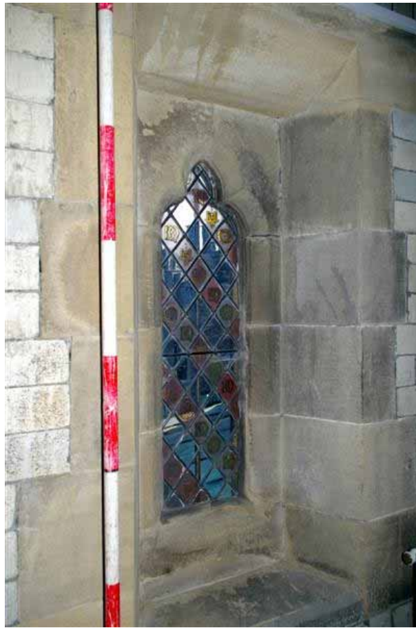
Plate 89: Window in Room U106
