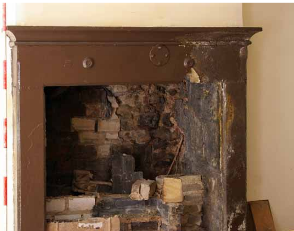
Plate 40: Fireplace in Room E007
