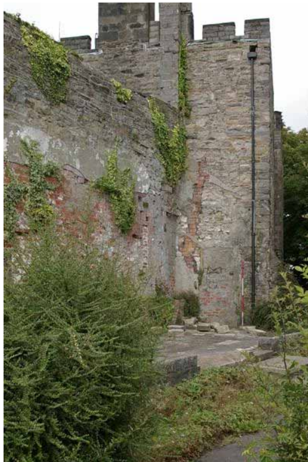
Plate 26: East side of the south-west elevation of the Museum south extension
