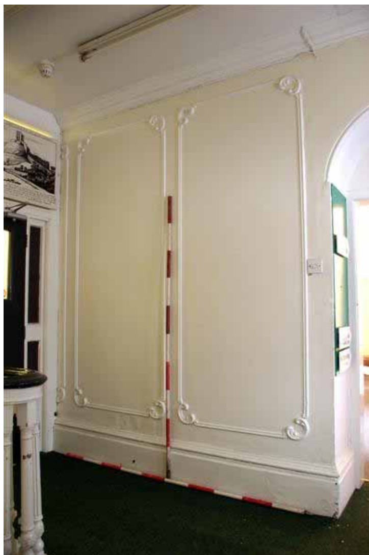
Plate 32: Panels in Room E001
