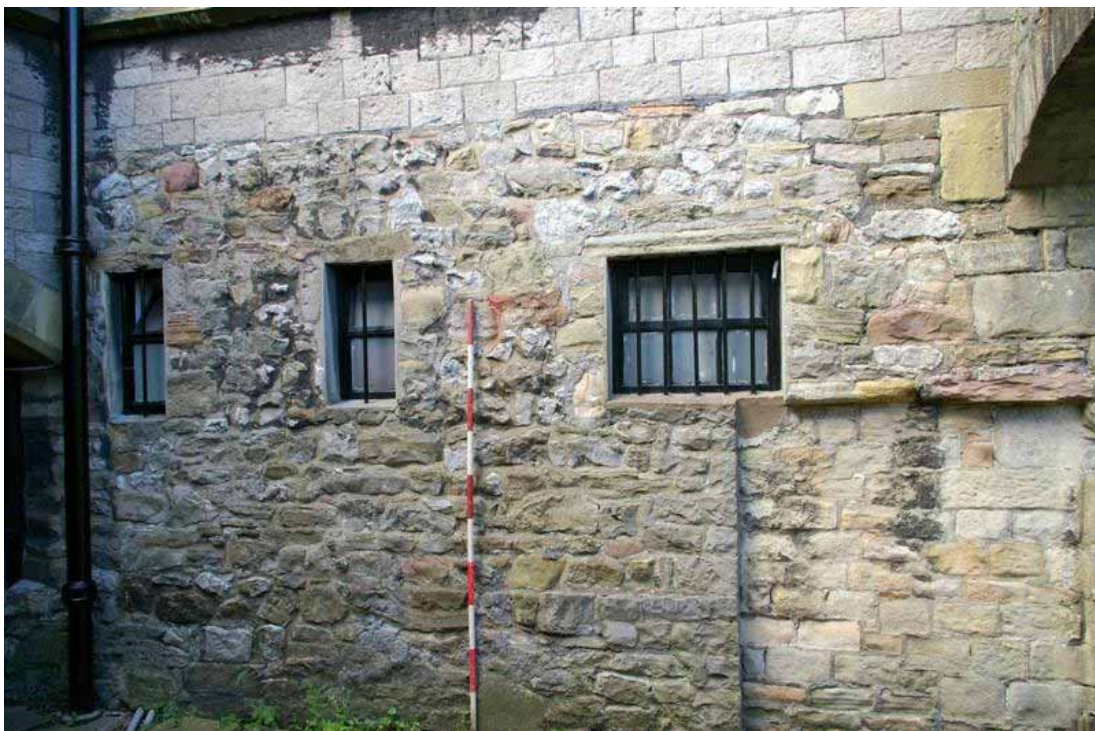
Plate 70: The lower part of Elevation 4 in the small courtyard
