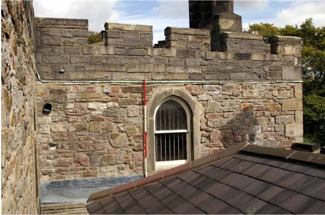
Plate 23: South-eastern side of the upper part of the Museum south-west elevation
