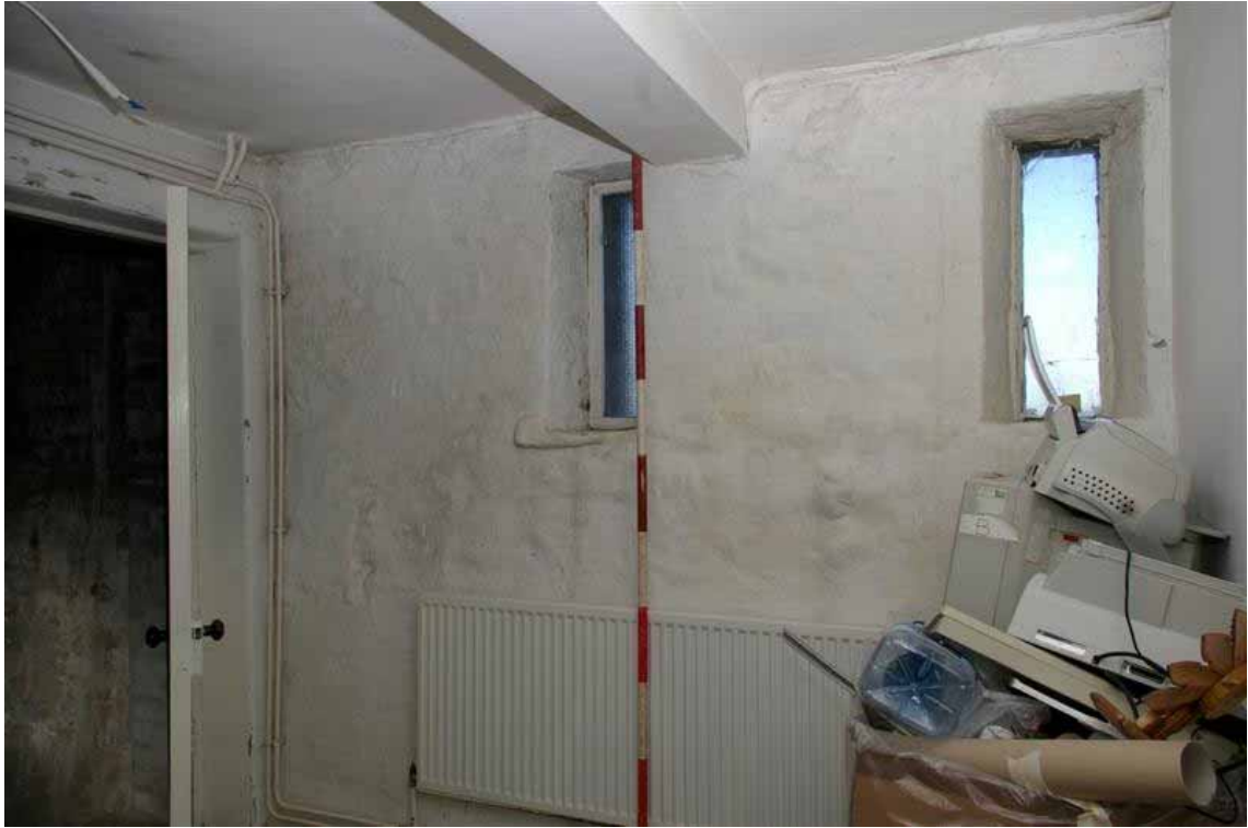
Plate 79: Windows in Room L111 of the Court House
