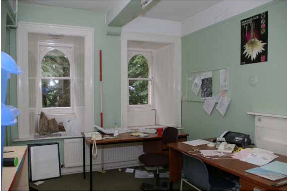
Plate 53: Fenestration in Room L007
