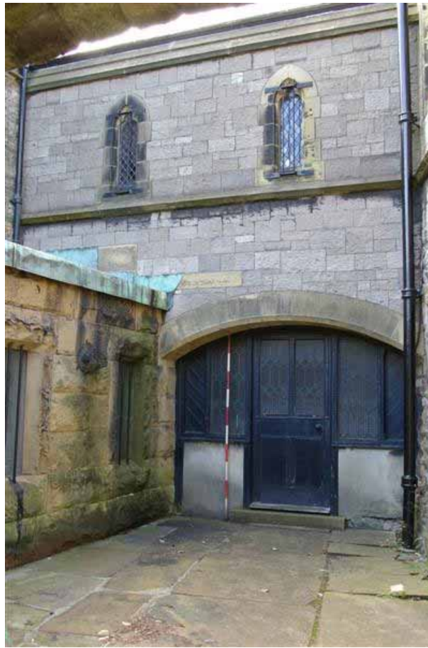
Plate 69: The east-facing elevation (Elevation 3) of the small courtyard
