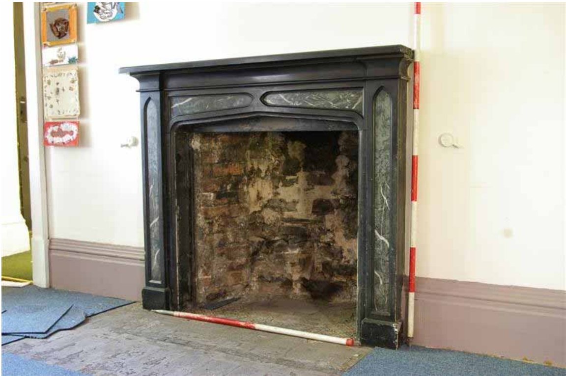
Plate 51: Fireplace in Room E012
