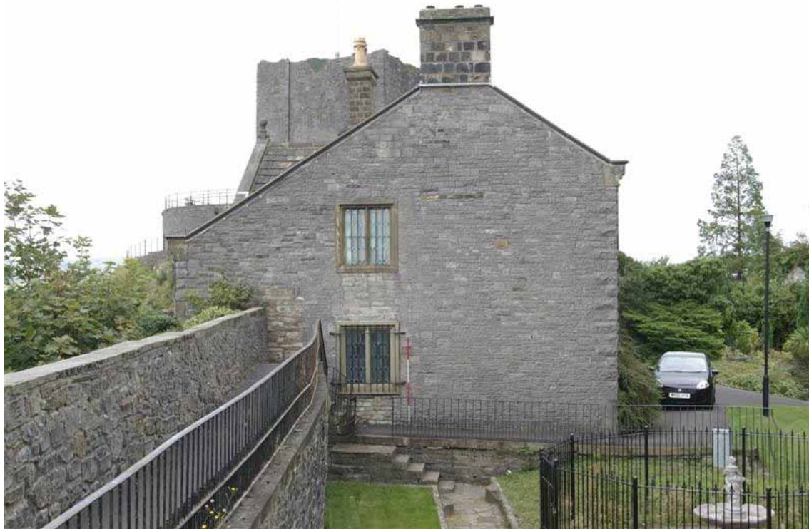
Plate 67: The south-facing elevation of the Sound Archive
