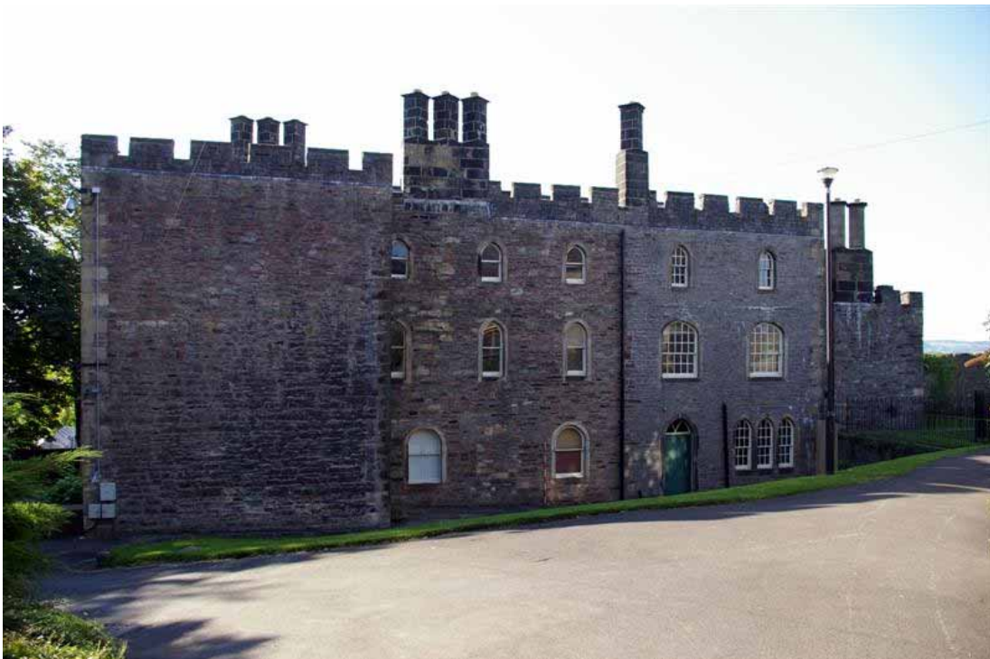
Plate 4: General view of the north-west elevation of the Museum
