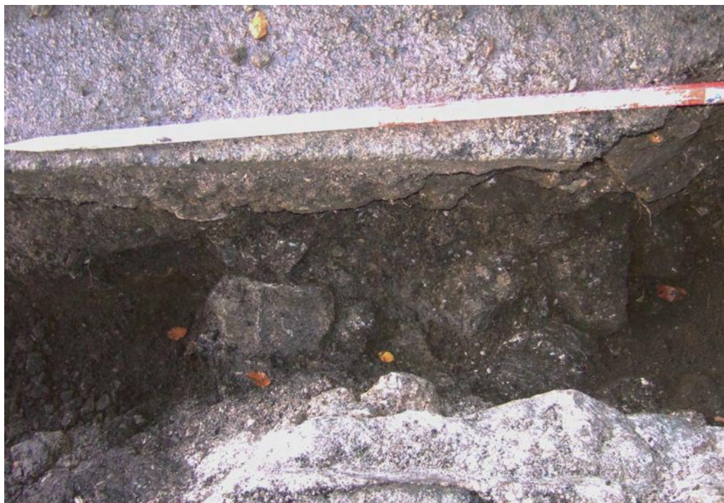
Plate 26: Stone exposed in base of trench
