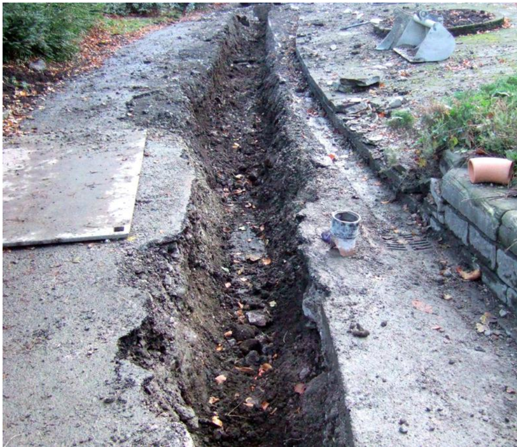
Plate 25: The service trench excavated along the upper part of the driveway
