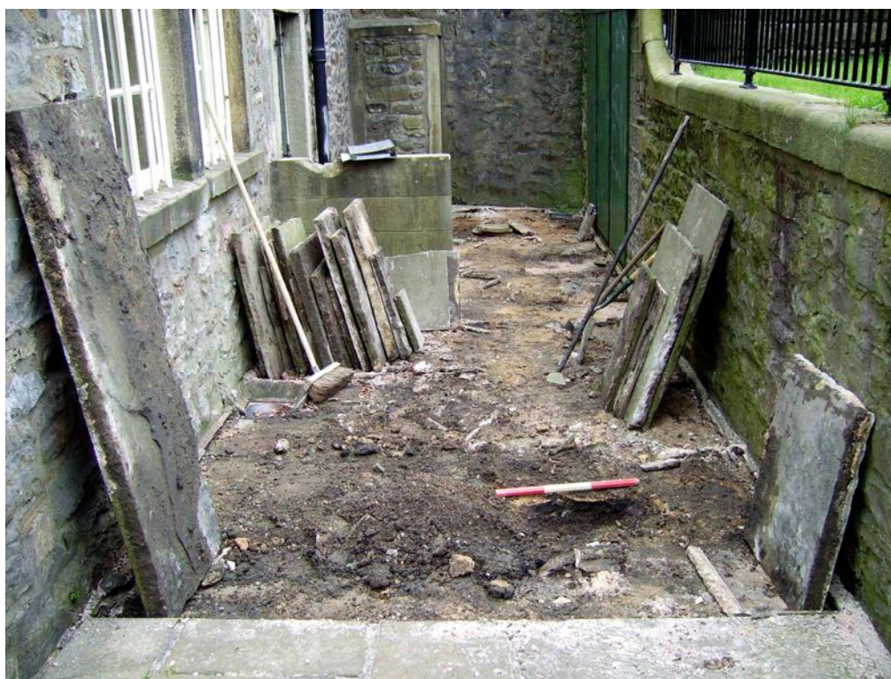
Plate 24: Removal of the flagstones to the rear of the museum in April 2007
