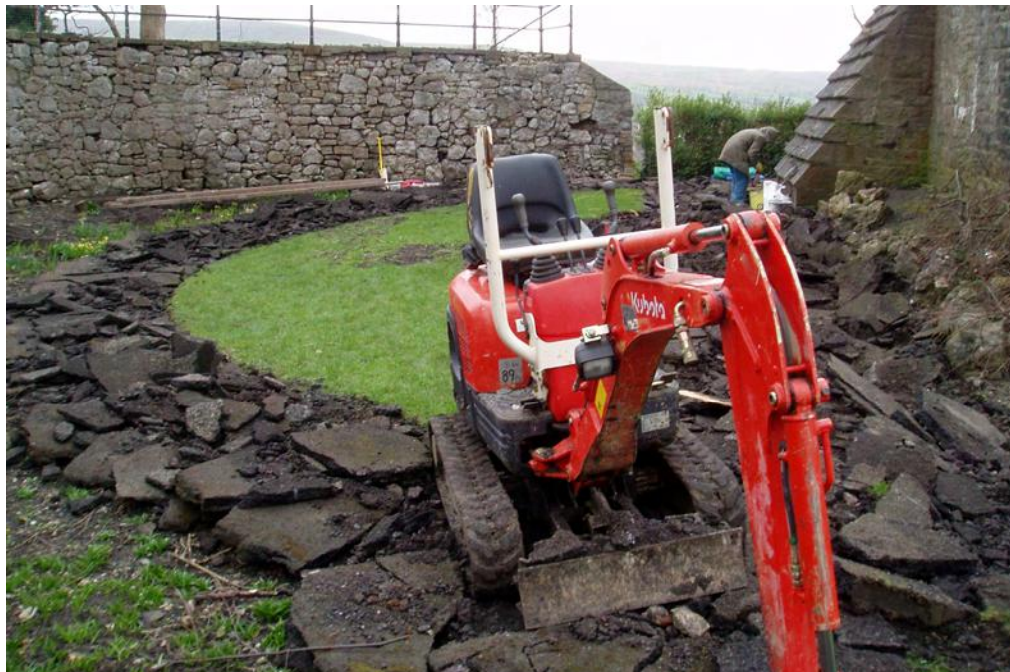
Plate 23: Removing the tarmac surfacing from around the castle keep
