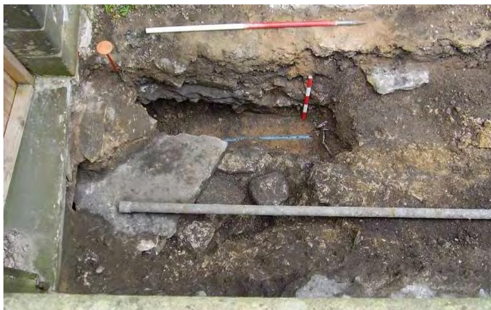
Plate 15: Culvert/conduit 1007 at the north-east end of the trench
