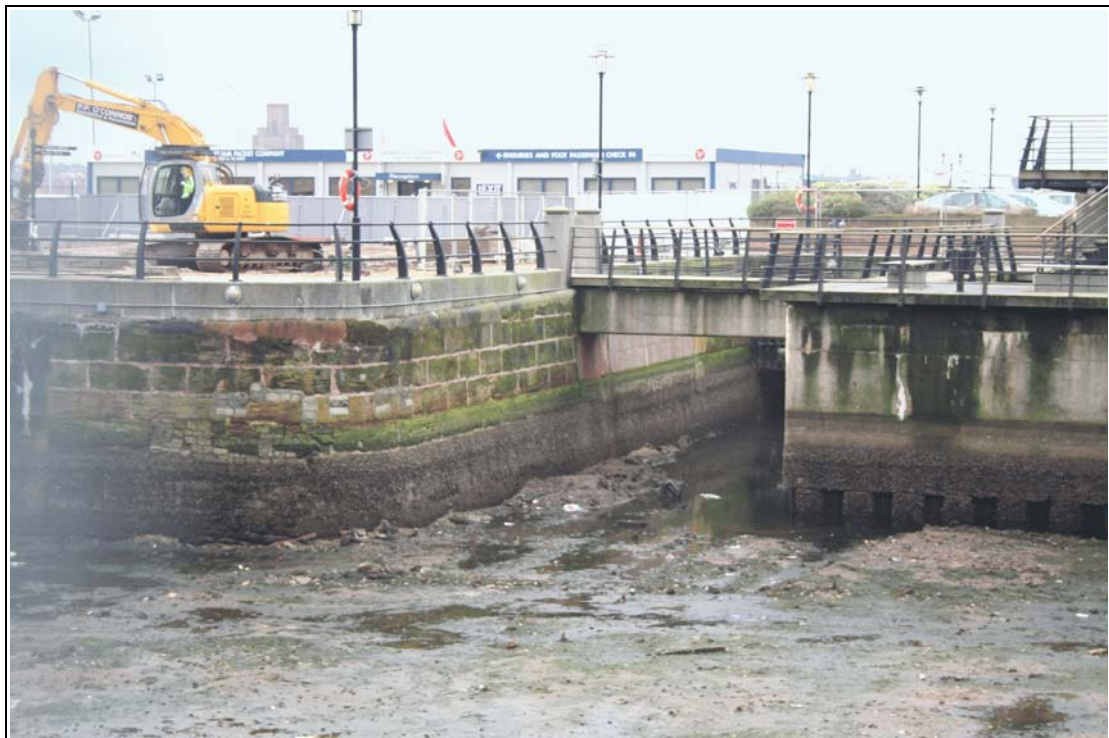
Plate 4: Princes Dock: south wall
