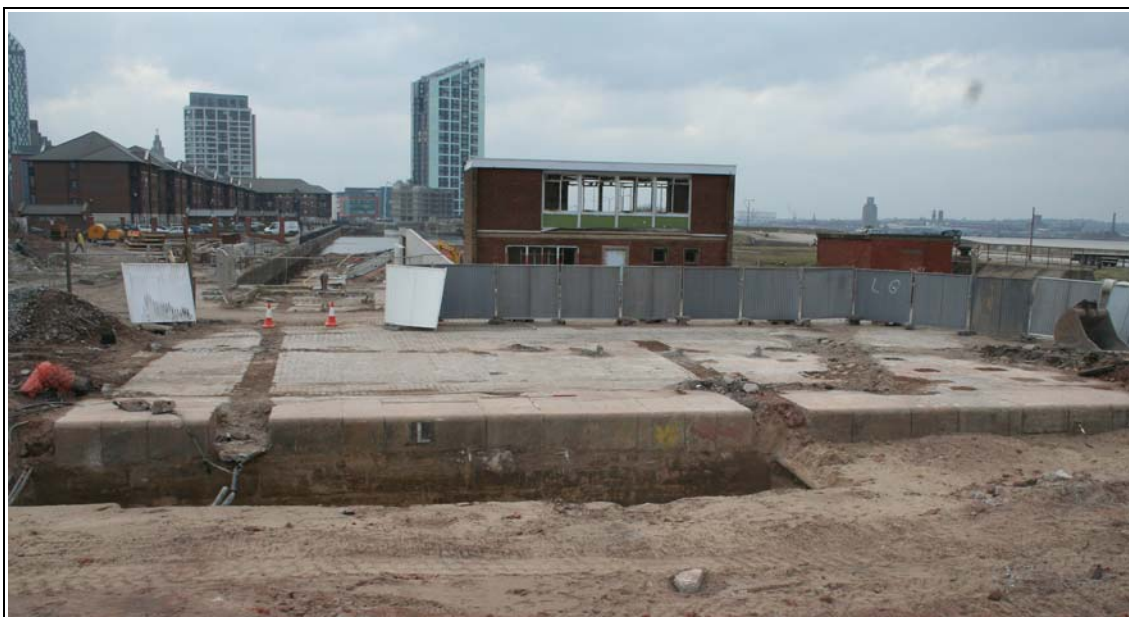
Plate 9: Office block at Trafalgar Dock
