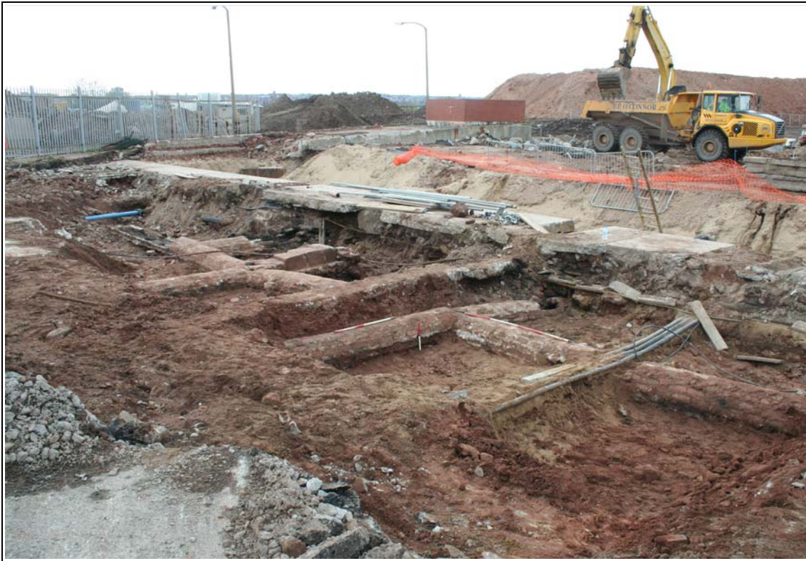
Plate 7: Brick-built culverts on the quayside between Trafalgar and Victoria Docks
