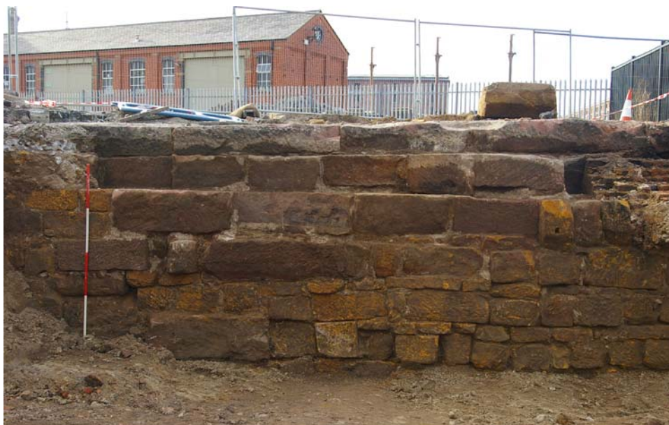
Plate 2: Trench 410 (LCL4), showing the north-facing, landward elevation of Manchester Dock wall
