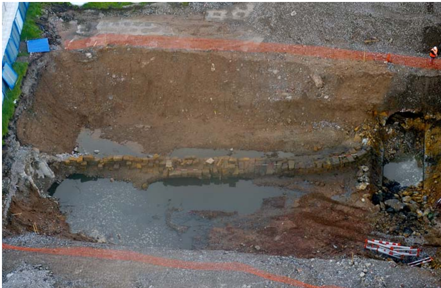
Plate 7: Trench 416 (LCL7), from the east, showing the mid-eighteenth-century sea wall truncated by the Liver Culvert
