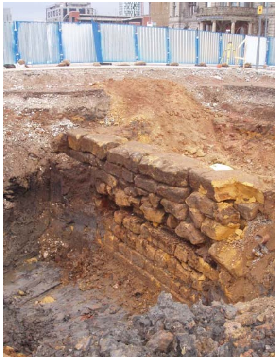
Plate 1: Trench 408 (LCL6), showing the west-facing elevation of the mid-eighteenth-century yellow sandstone sea wall
