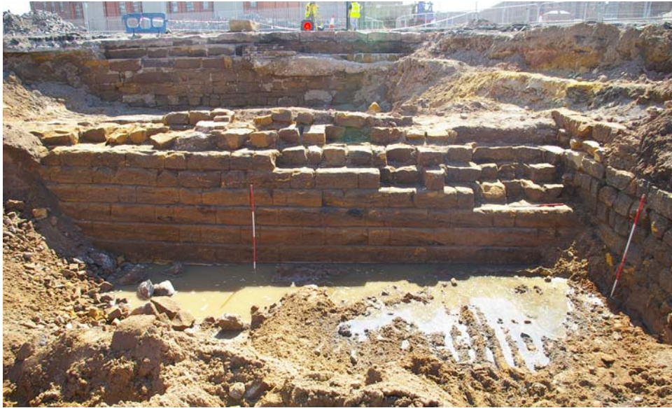
Plate 3: Trench 410 (LCL4), showing the Old Quay, and ( right ) the mid-eighteenth-century sea wall. The north-facing elevation of Manchester Dock is in the background
