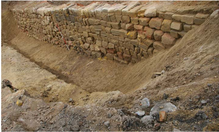
Plate 5: Trench 412 (LCL5), showing the north face of a temporary wall, constructed at an intermediate stage in land reclamation
