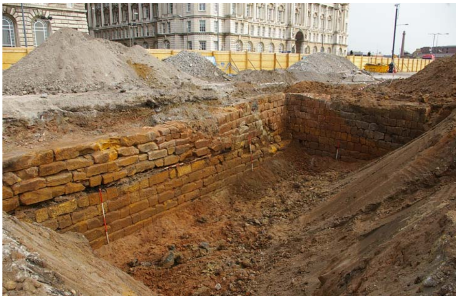
Plate 6: Trench 414 (LCL6), showing ( left ) the west-facing elevation of the mid-eighteenth-century sea wall, and ( right ) the north-facing elevation of a temporary wall, installed at an intermediate stage in a further phase of land reclamation
