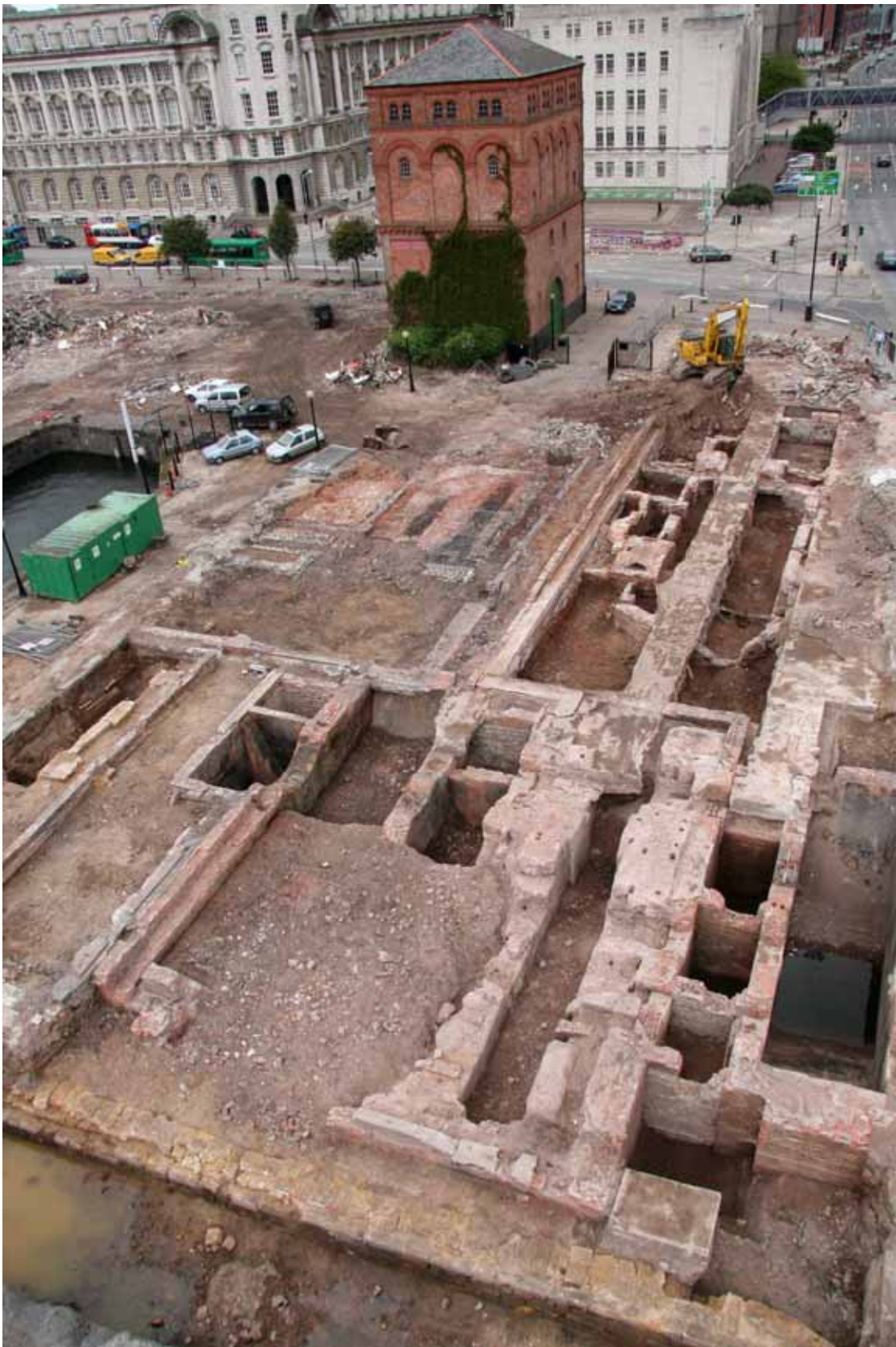
Plate 4: Aerial view of Area B looking north, with the yellow sandstone Dry Dock wall in the foreground and the Mersey Tunnel Ventilation Station immediately behind
