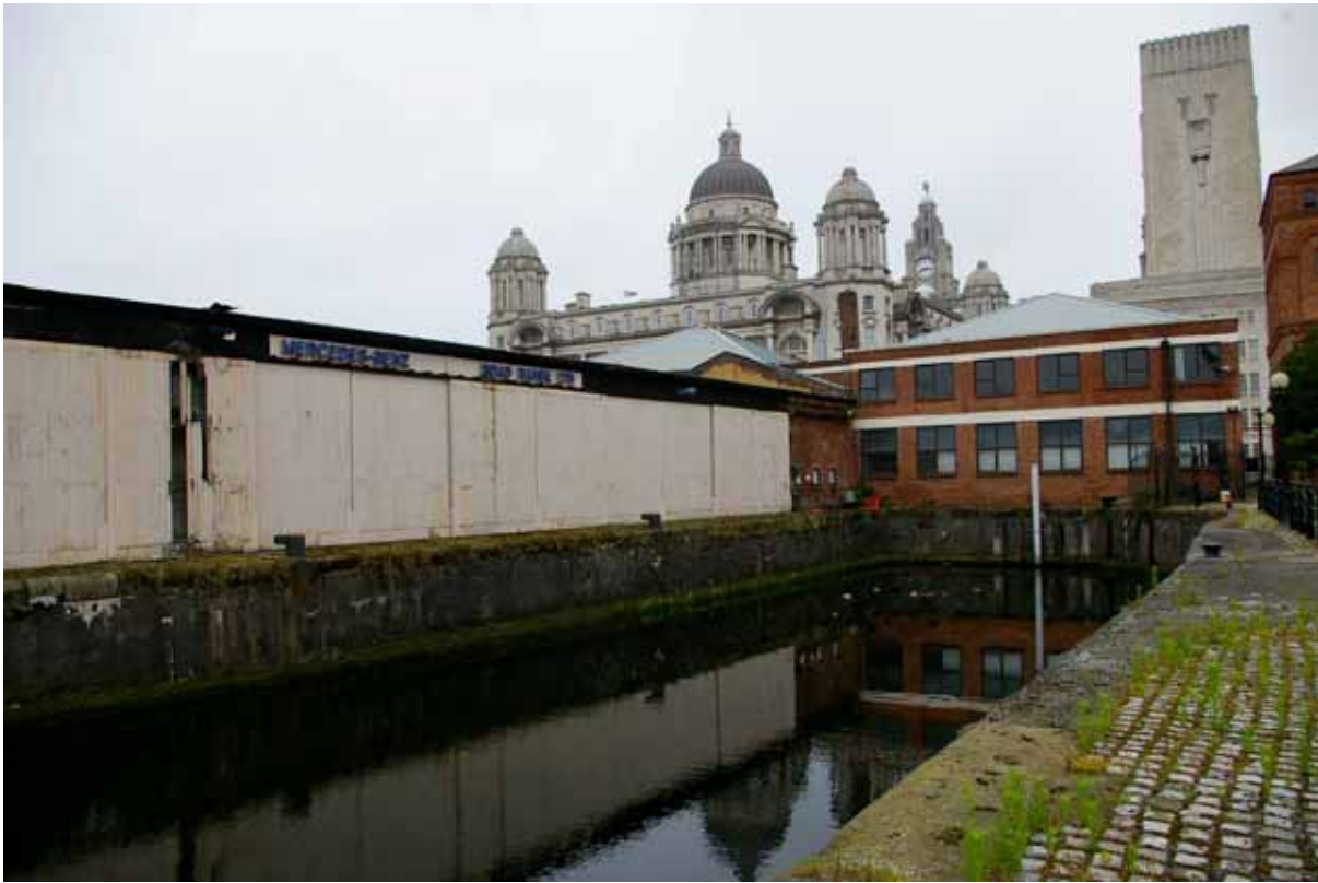
Plate 1: Transit Shed (left) and Voss Garage (centre) adjacent to George's Dock Passage, prior to excavation
