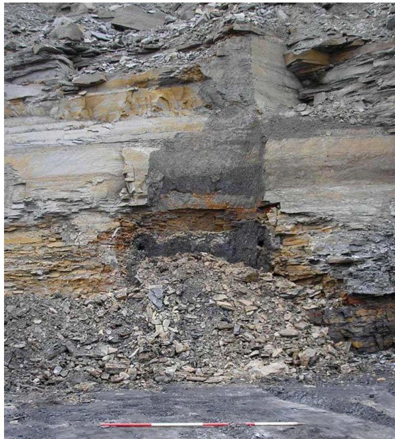
Plate 21: Unlined ventilation shaft uncovered in Area C
