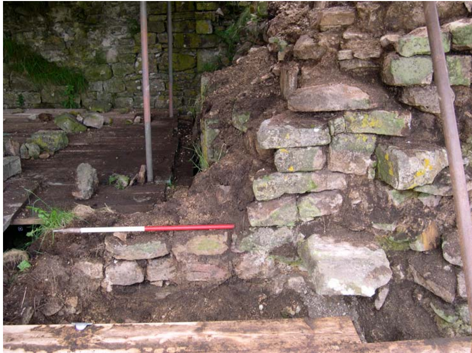
Plate 11: Remains of stair, west curtain wall, internal face
