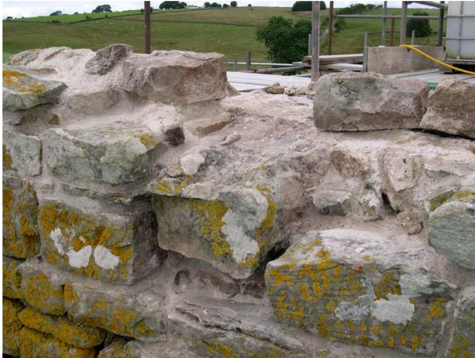
Plate 17: Floor-level drainage channel, south elevation of the barbican
