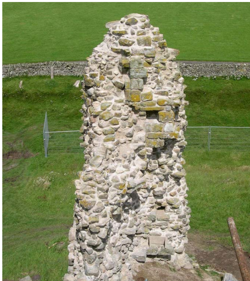
Plate 12: In situ door jamb, west curtain wall
