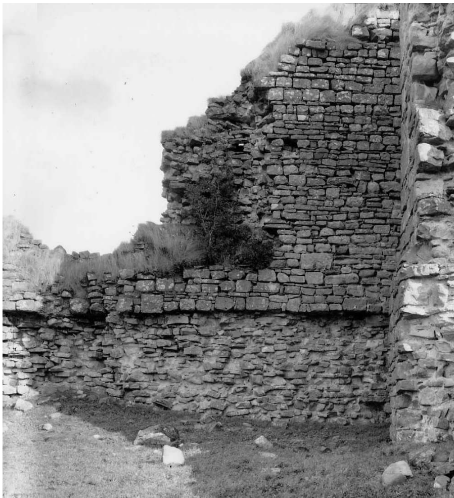
Plate 6: West curtain wall, external view, immediately north of the Phase 2 barbican
