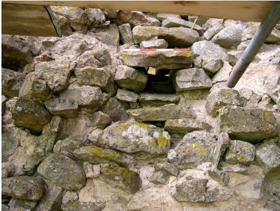
Plate 9: Probable loophole, west curtain wall, external face
