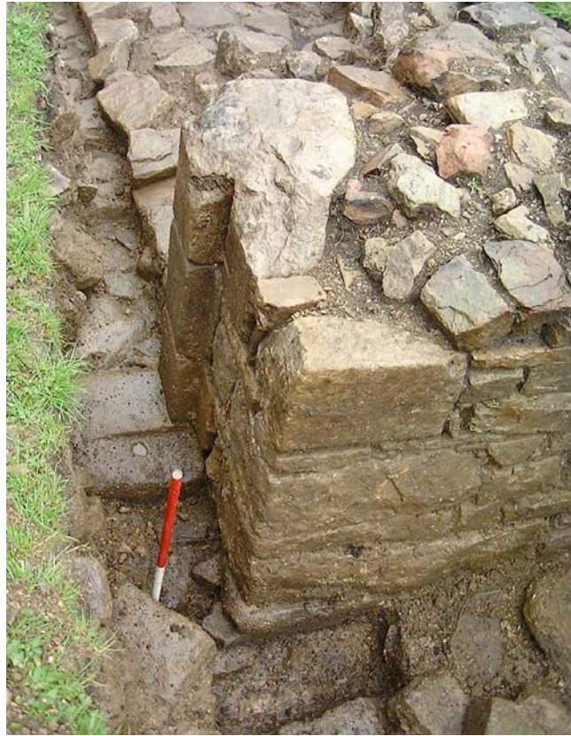
Plate 25: Rebated internal side of doorway, wall 06
