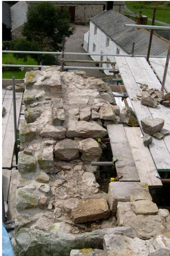
Plate 16: Parapet walkway, south elevation of the barbican
