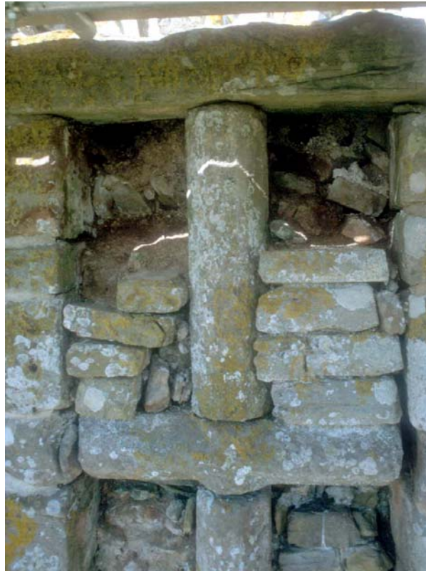
Plate 19: Phase 3 inserted window, west end of south curtain wall, external face
