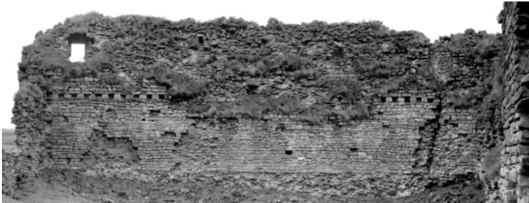
Plate 8: South curtain wall, internal view, showing flues
