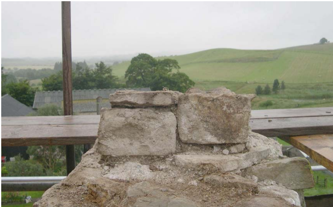
Plate 18: Parapet walkway, west elevation of the barbican
