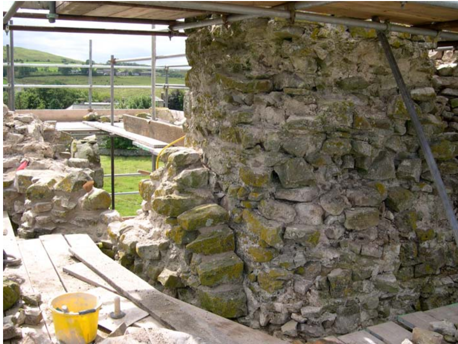
Plate 13: Straight joint between Phase 2 barbican and curtain wall
