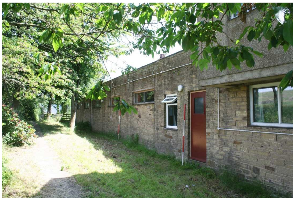
Plate 17: North-facing elevation of the communal part of the 1968 YHA building
