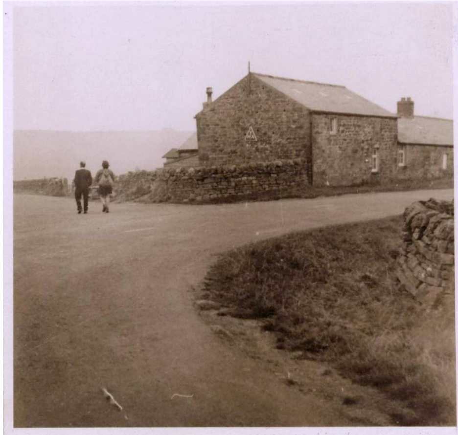
Plate 5: A view of the eastern end of the Once Brewed Youth Hostel at East Bog Farm. The B6318 runs across the image from left to right and the walkers are descending towards Henshaw
