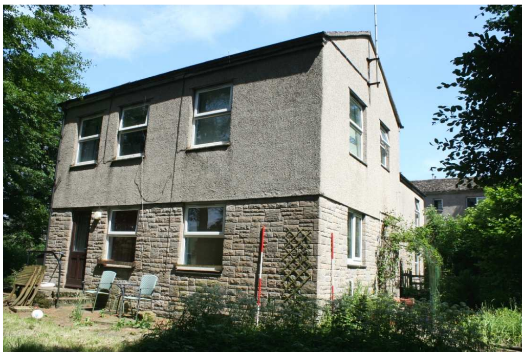
Plate 20: Manager's living accommodation, on the end of the western dormitory wing extension
