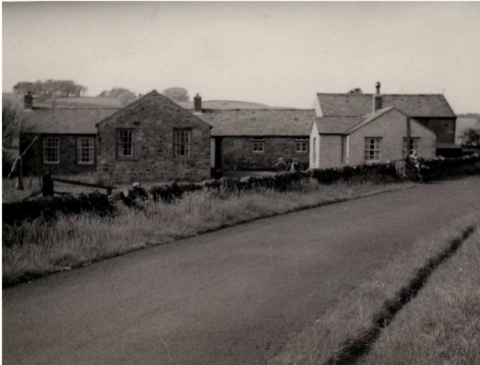
Plate 9: A view of the youth hostel looking north, following the addition of a rendered extension at the eastern end of the building between 1934 and 1968
