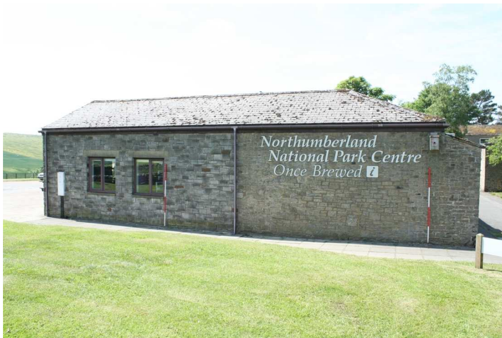
Plate 22: The east-facing elevation of the NNPA Visitor Centre, showing the wall scar where the east wing extension has been constructed (left of photo)
