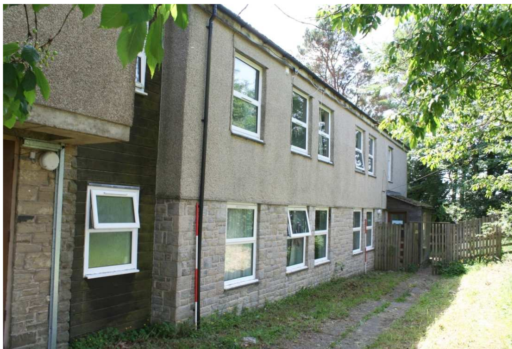
Plate 19: North-facing elevation of western dormitory wing extension and the wood-clad corridor adjoining it to the 1960s YHA building
