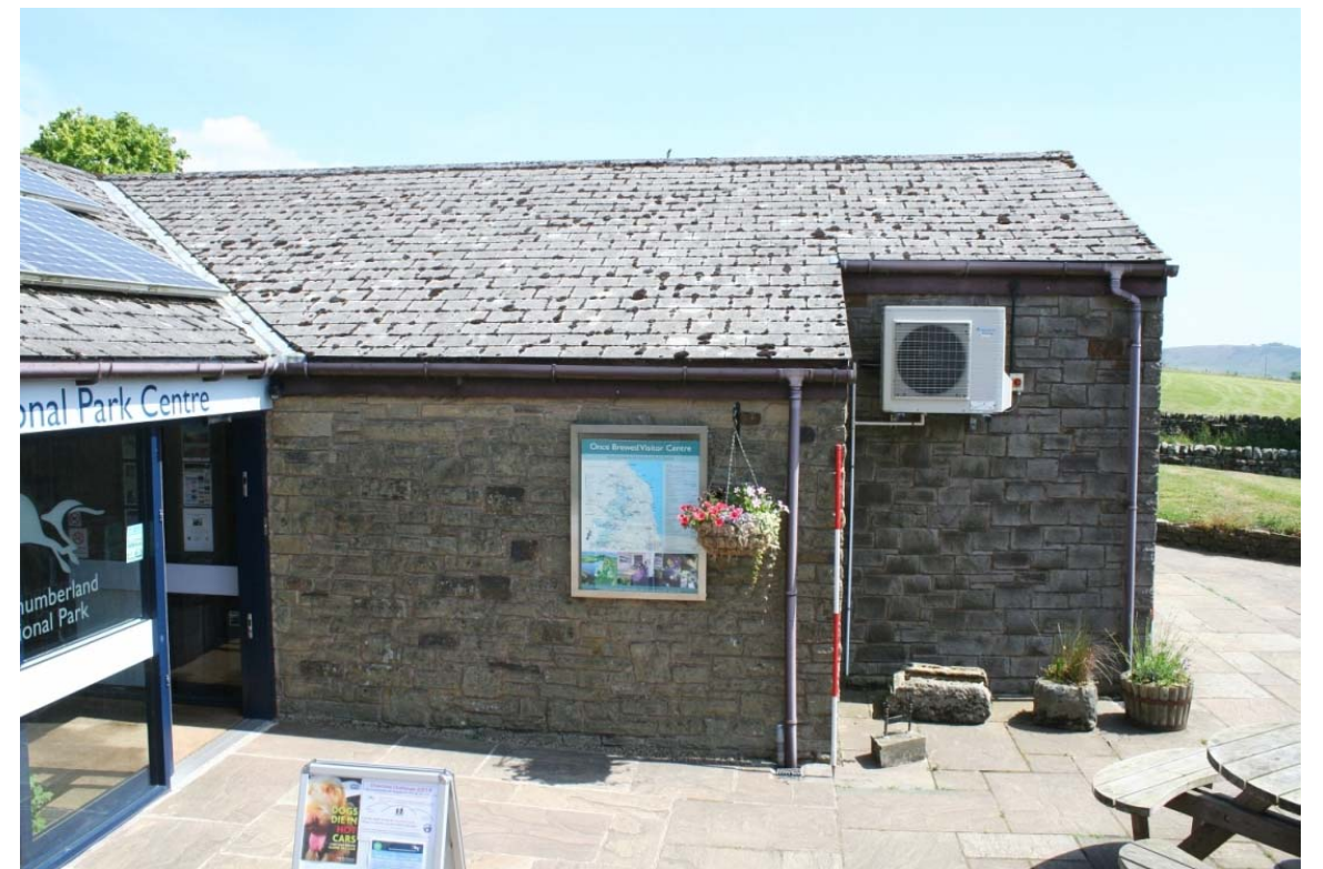
Plate 21: The west-facing elevation of the NNPA Visitor Centre, on the east wing
