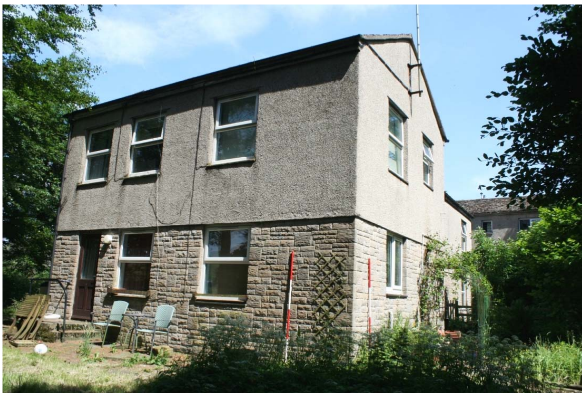
Plate 13: Manager's living accommodation, on the end of the western dormitory wing extension
