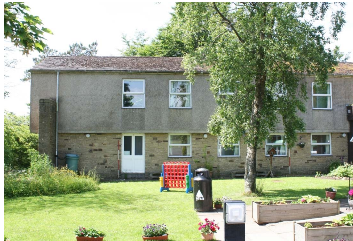
Plate 11: East-facing elevation of the original dormitory wing of the 1960s YHA building
