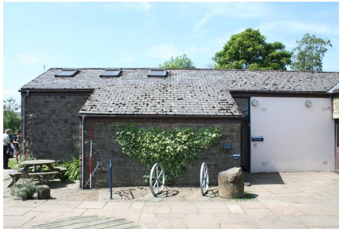
Plate 19: The east-facing elevation of the NNPA Visitor Centre, on the west wing
