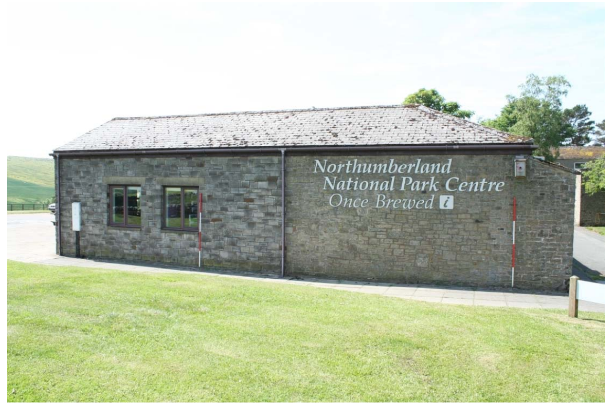
Plate 20: The east-facing elevation of the NNPA Visitor Centre, showing the wall scar where the east wing extension has been constructed (left of photo).
