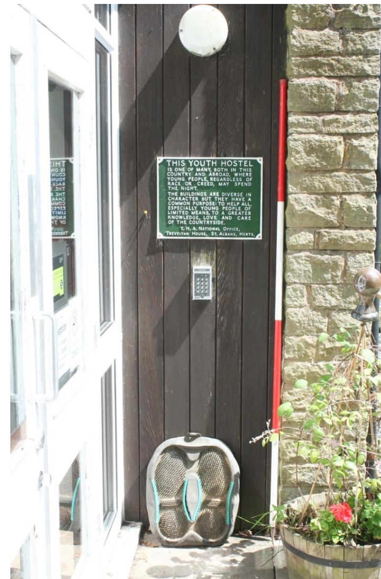
Plate 6: Detail of the metal signage at the main entrance to the 1960s YHA building
