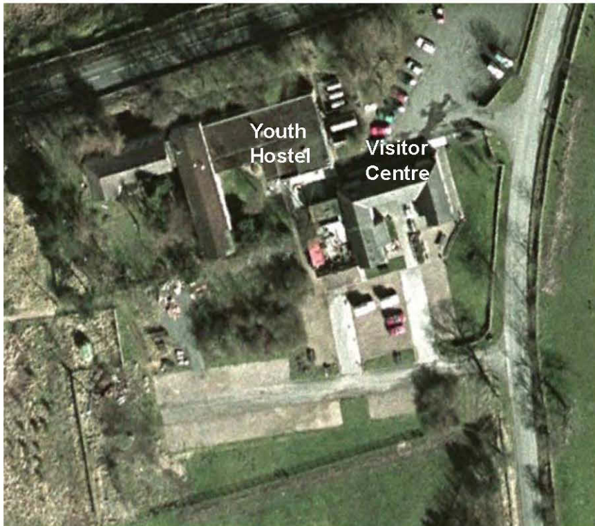
Figure 3 – Aerial photograph indicating the buildings on site. (Reproduced under licence from Google Earth Pro.)
