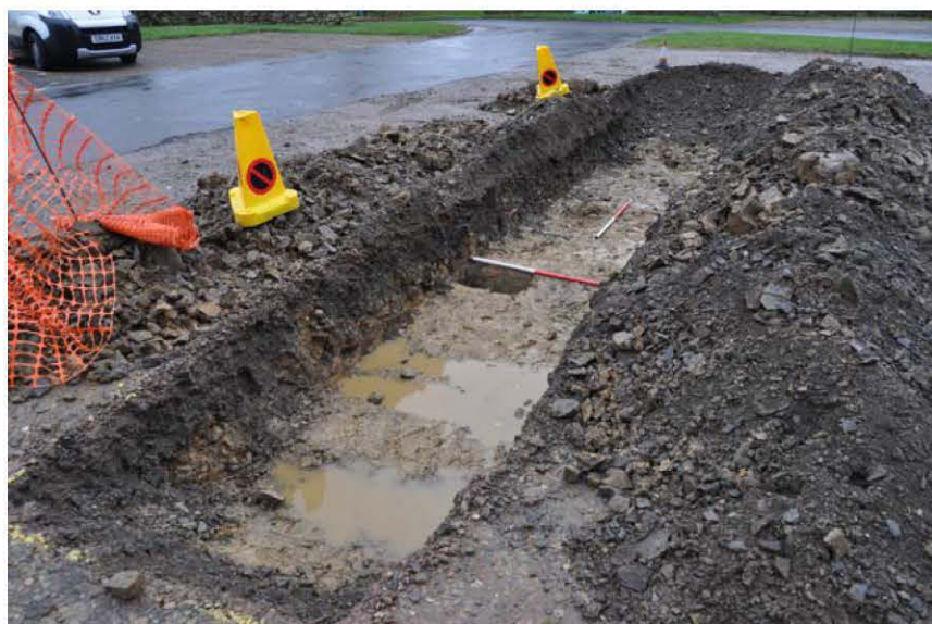
Plate 4: Trench 4 – Facing south-east, 2x1m scales
