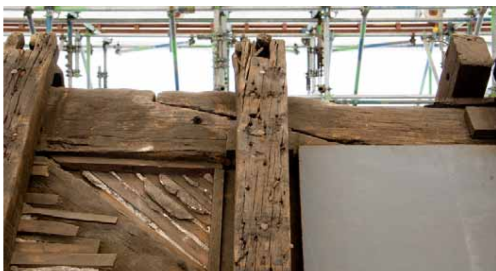
Plate 55: Bridled scarf joint in ridge purlin (Roof D)
