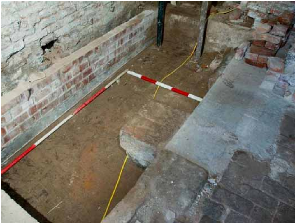
Plate 28: Footings of staircase and newel
