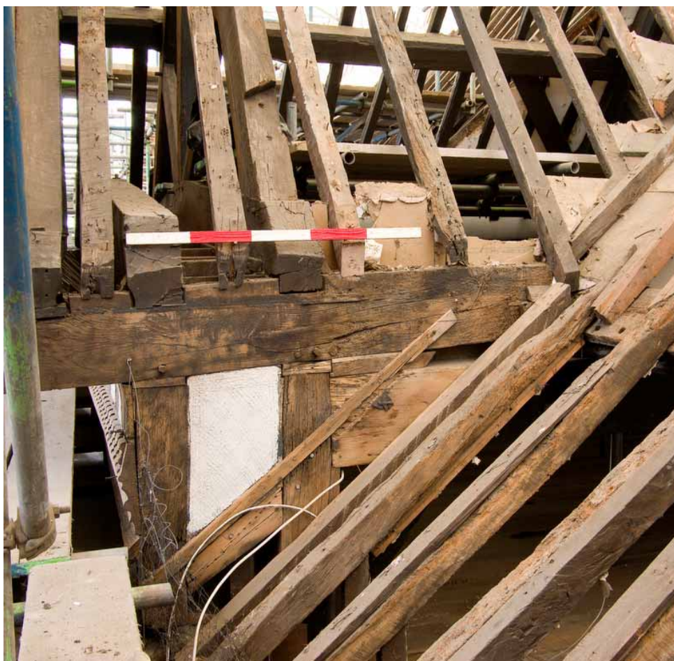
Plate 63: Triple-pegged wall frame, showing normal assembly, and with jetty bressumer beam to left (Roof F)
