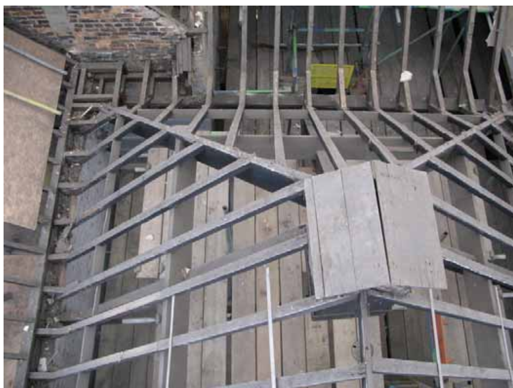
Plate 67: Late hipped Roof H, with raised timber louver
