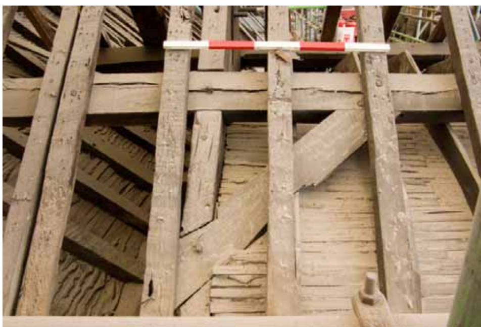
Plate 60: Detail of wind-brace jointing (Roof E)
