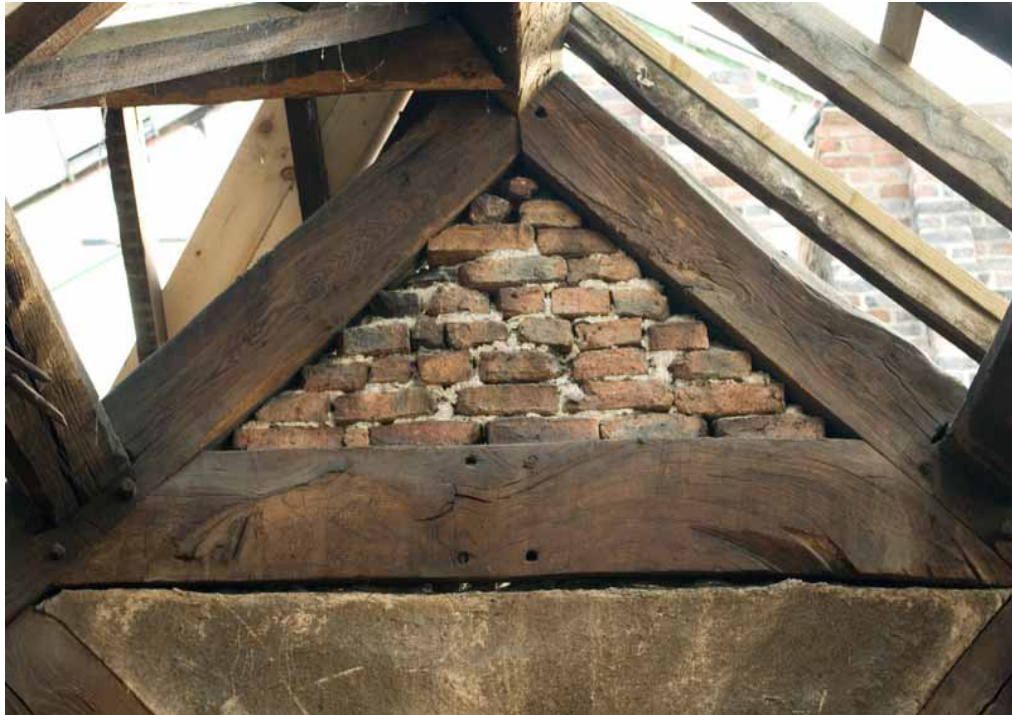
Plate 38: Detail of truss apex, showing ridge assembly, and brick noggin
