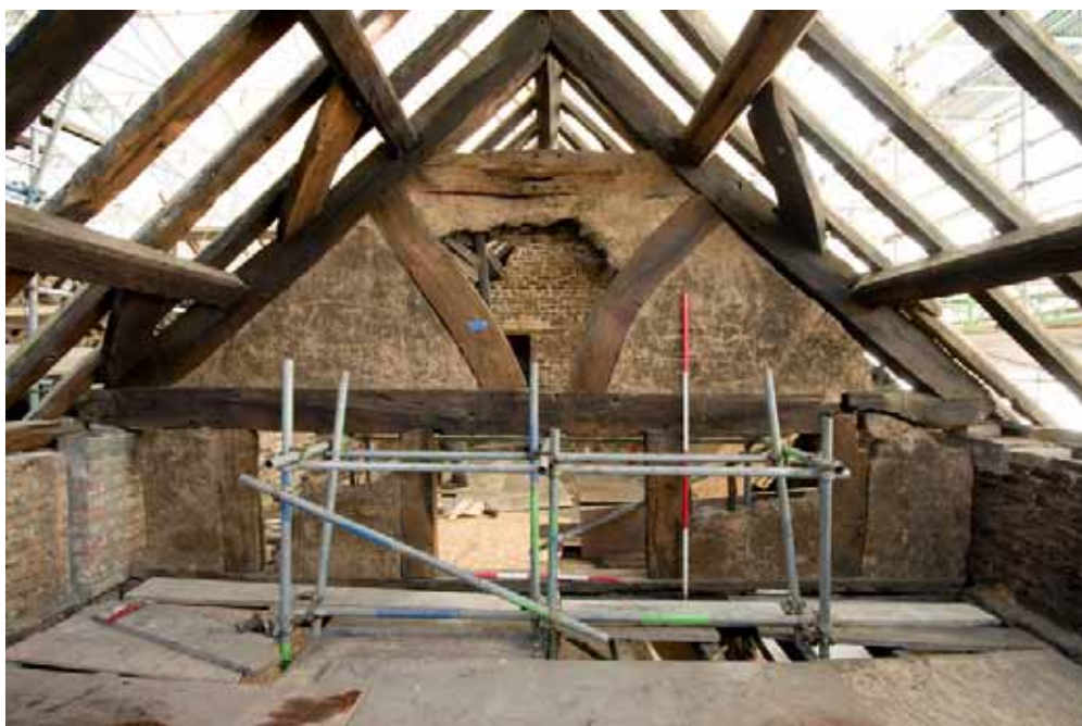
Plate 40: Southern truss of the west wing, with original wind braces
