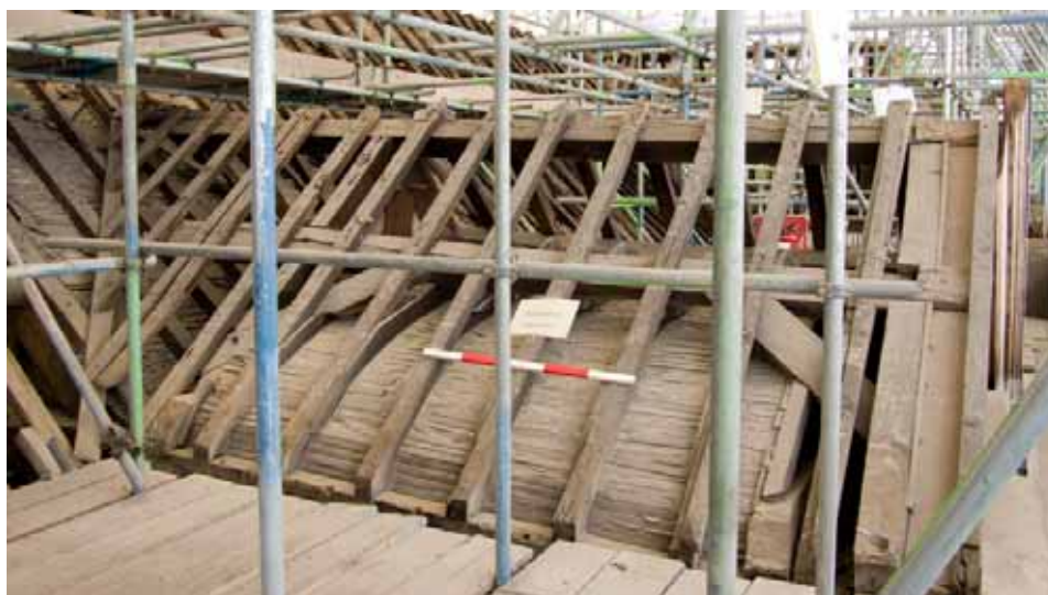
Plate 59: Roof E, with king-post truss either end, and vaulted ceiling
