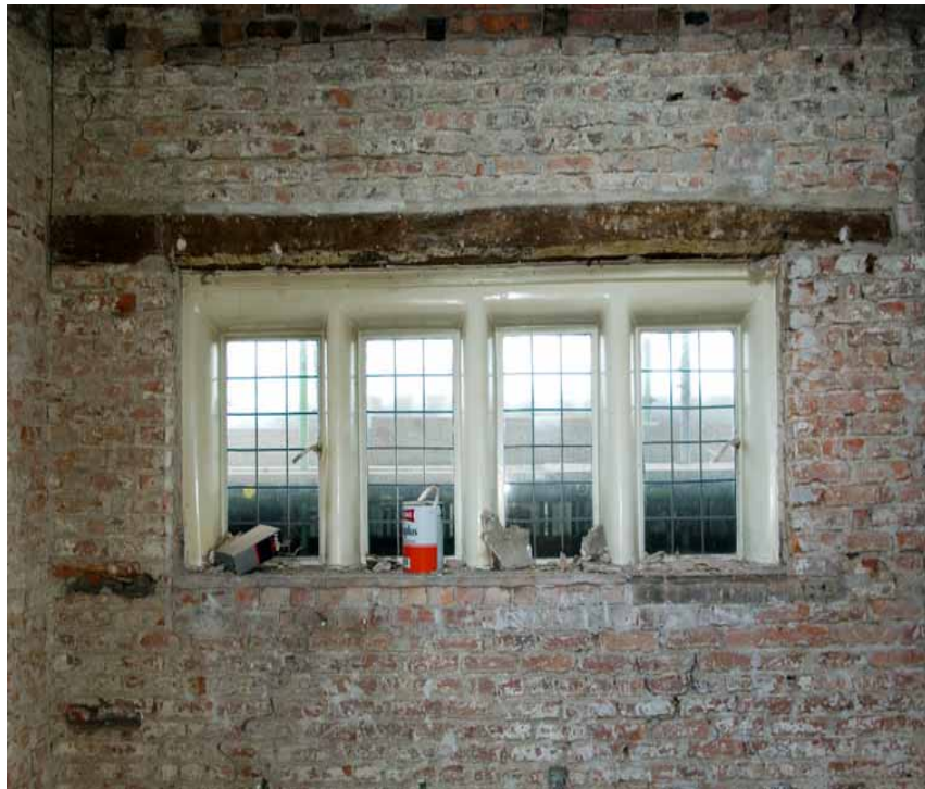
Plate 21: Remodelled first-floor window in Stair Tower
