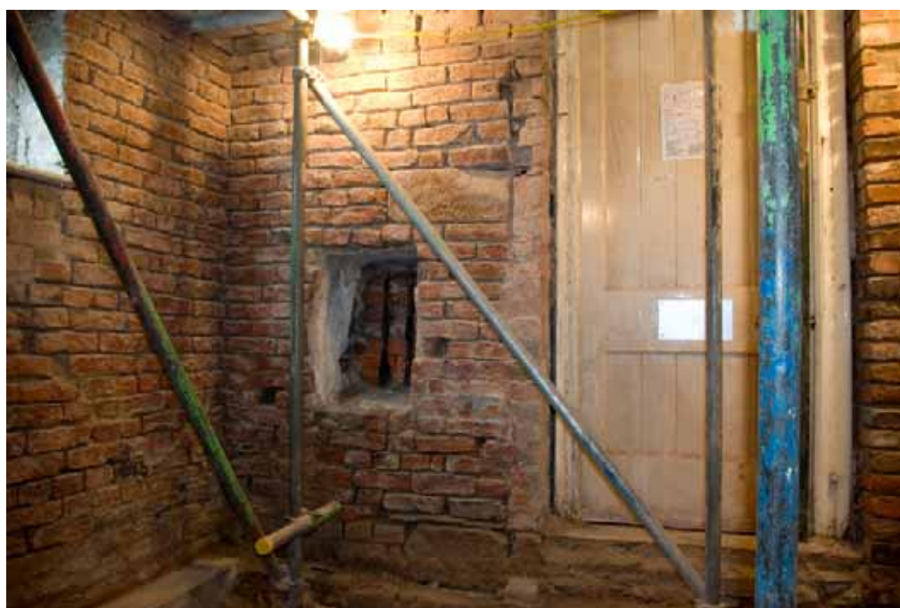
Plate 26: Small window with wrought-iron bars revealed at ground-floor level
