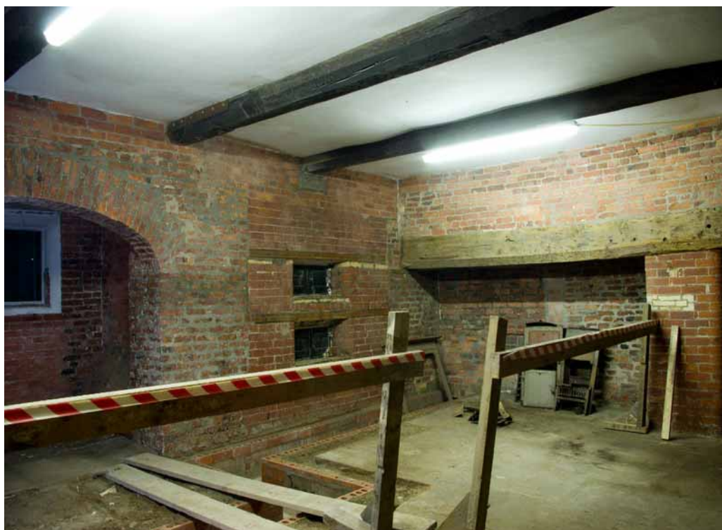
Plate 11: General aspect of the Kitchen (G10), with large inglenook fireplace and bread ovens
