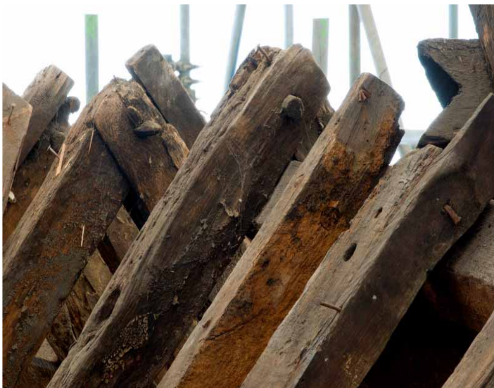
Plate 48: Halved and pegged common rafters, Roof C
