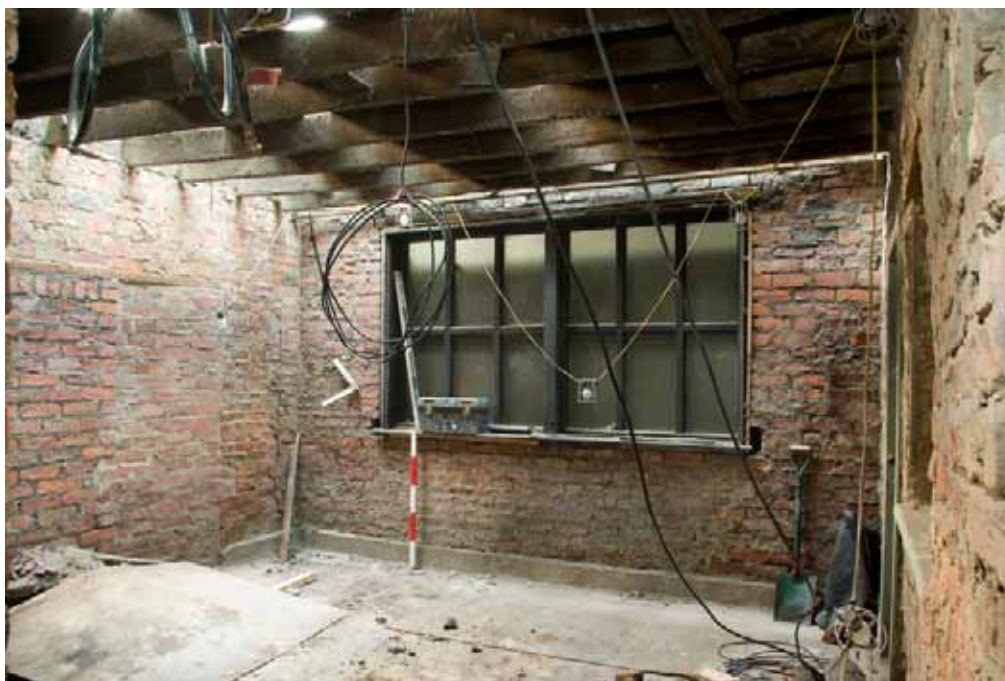
Plate 30: Rebuilt north wall of the Gardener's Office
