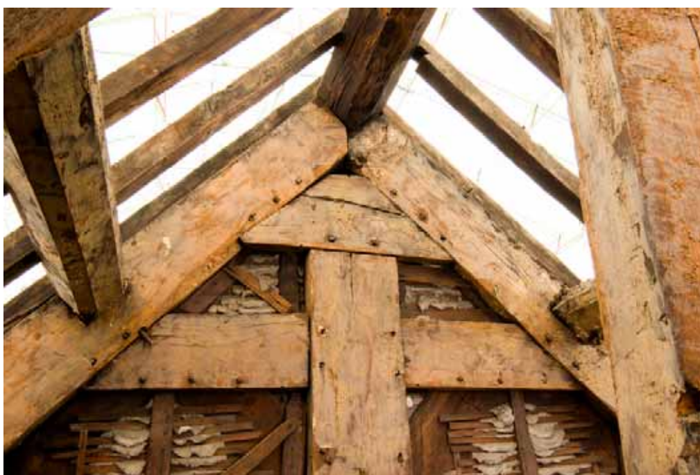
Plate 58: Saddle within truss construction, and pegging of decorative panelling (Roof D)
