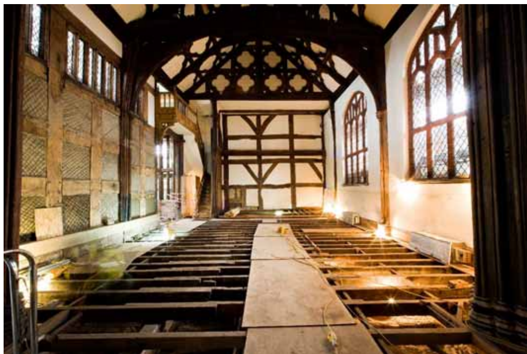
Plate 92: View of the Great Hall looking north-east
