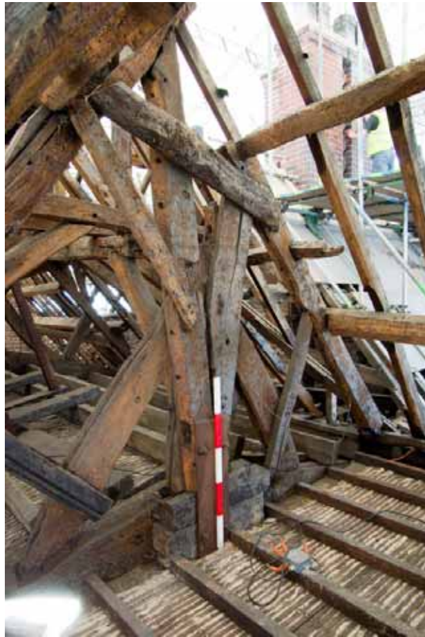
Plate 51: Remodelling of southern truss, Roof C, with inserted short principal rafters
