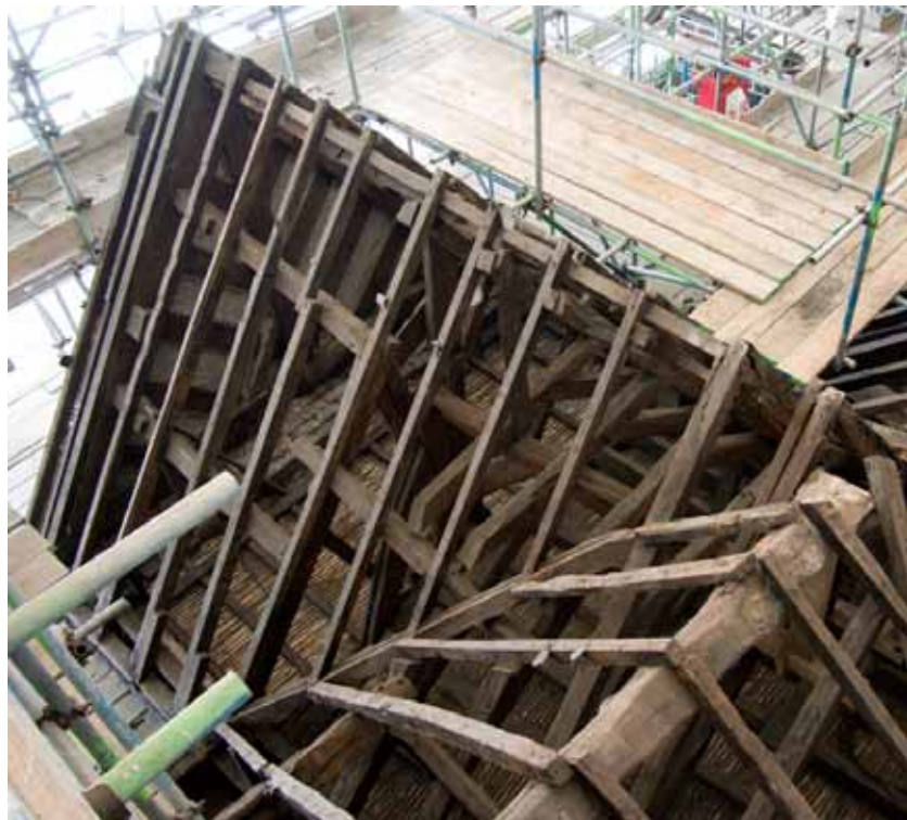
Plate 50: Remodelled southern part of Roof C
