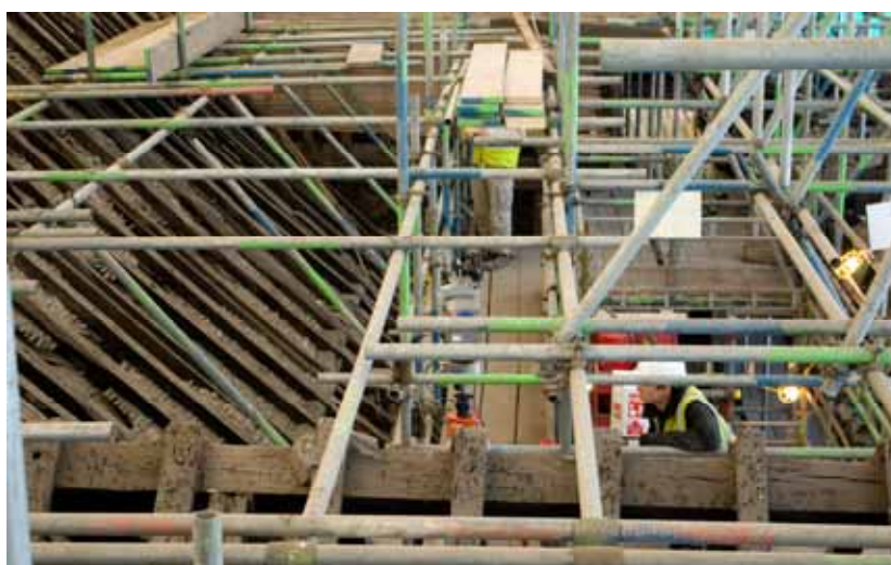
Plate 77: Laser scanning of the external roof structure
