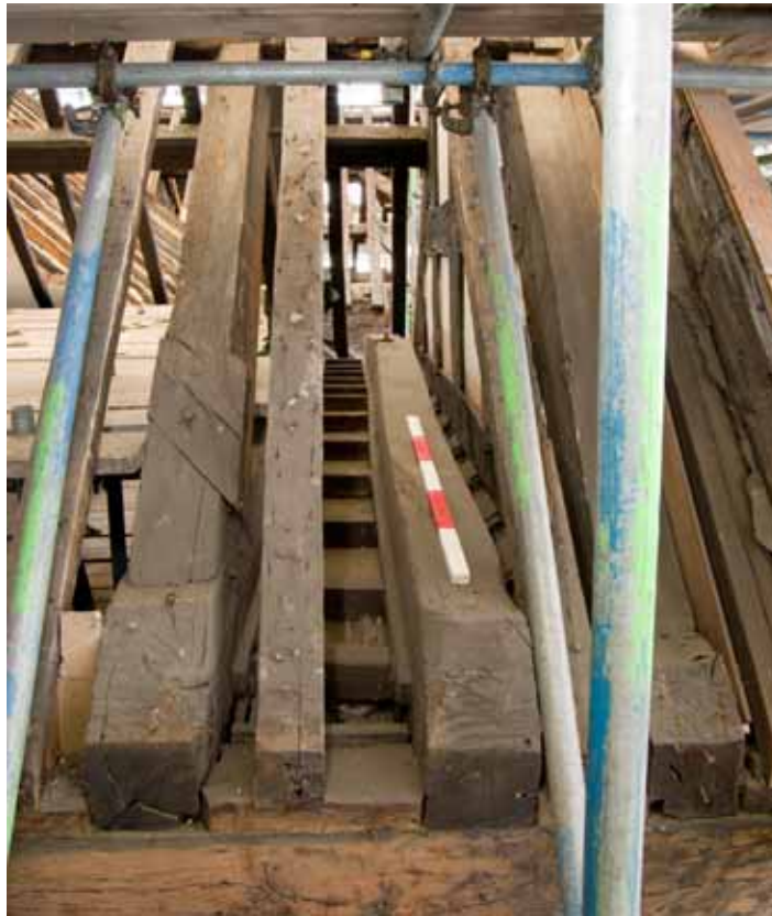
Plate 64: Jetty bressumer and trusses, northern end of Roof F
