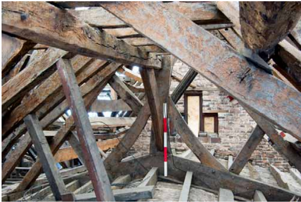
Plate 46: Northern truss, clasp crown post, Roof C
