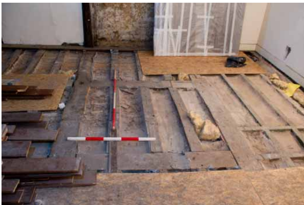
Plate 33: Area of floor structure exposed in the Lord's Chamber
