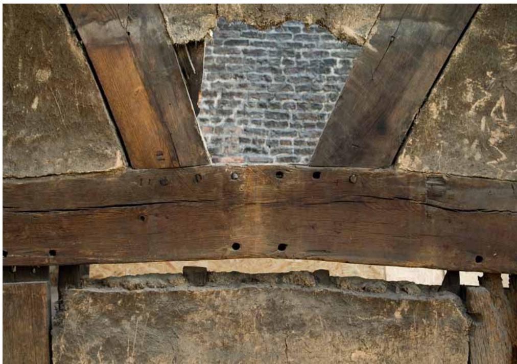
Plate 39: Assembly marks and redundant mortices, with wattle and daub panelling
