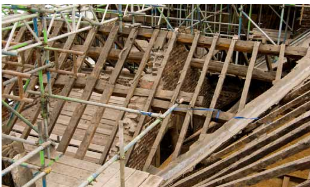
Plate 75: Trenched purlins and butt-jointed jack rafters, Roof L
