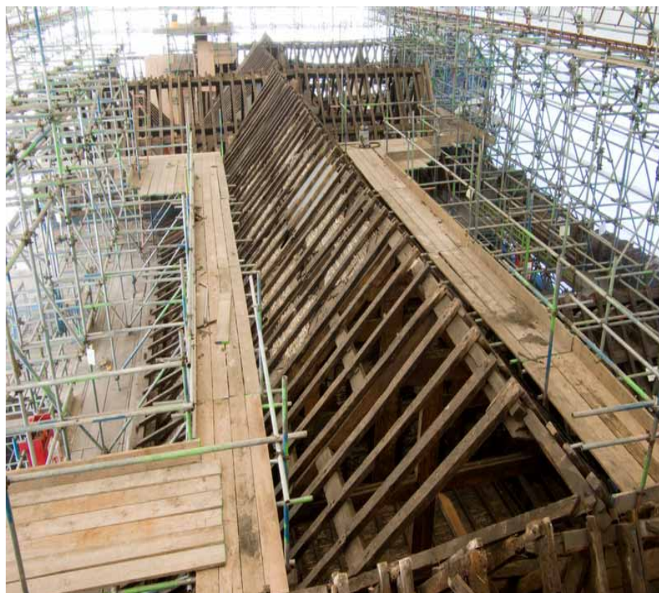
Plate 53: General view of stripped Roof D, with sprocketing to southern parapet
