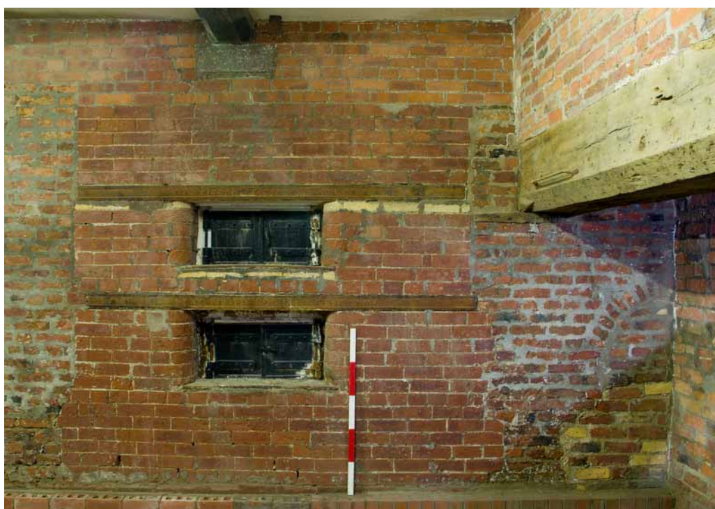
Plate 14: Detail of inserted bread ovens
