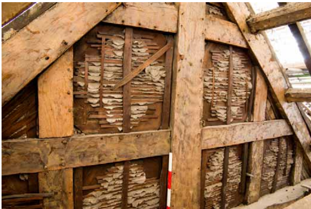
Plate 57: Lower face of truss forming Dais in Great Hall (Roof D)
