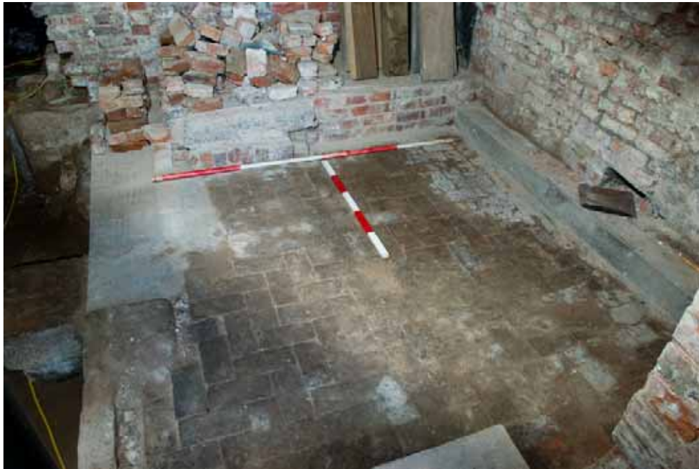
Plate 27: Herring-bone brick floor of Stair Tower
