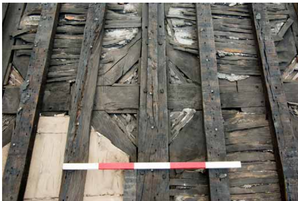
Plate 54: Pegged jointing of decorative timber panels on Roof D
