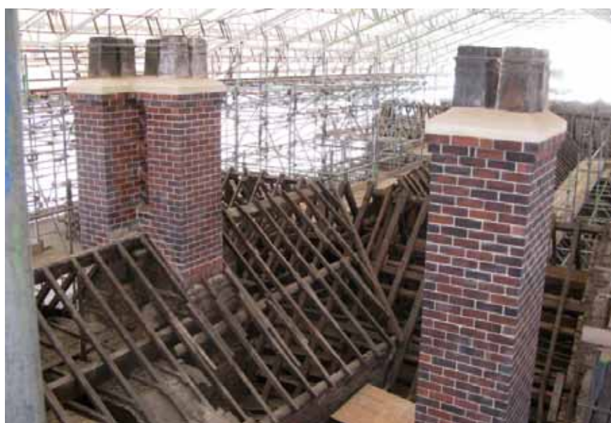
Plate 43: Roof A, with triple-pillared chimney-stack and remodelled purlins and rafters
