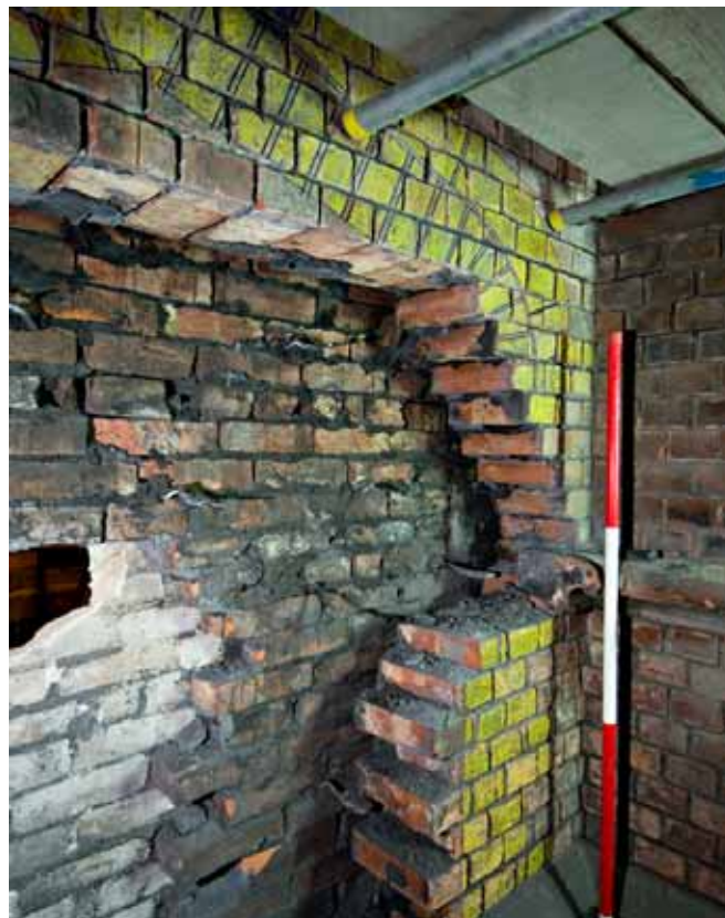
Plate 7: Detail of cavity wall construction
