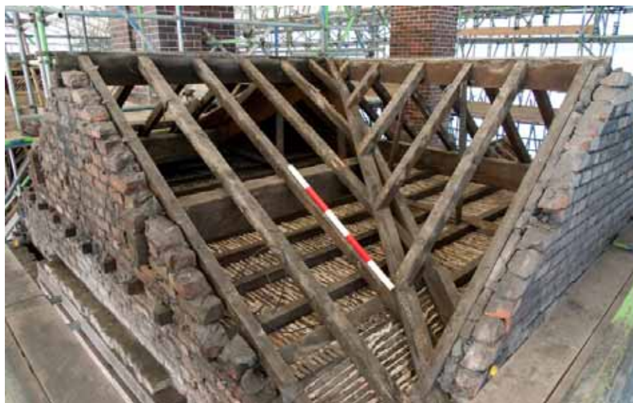
Plate 42: Roof A, with timbers projecting through single-skin southern gable (left)
