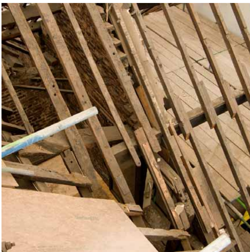
Plate 66: Brick gable, incorporating tie beam with normal assembly to wall post (Roof G)
