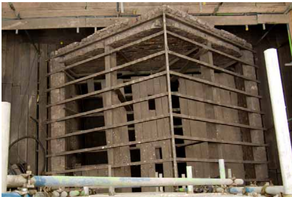
Plate 76: Slender timbers of late Roof M
