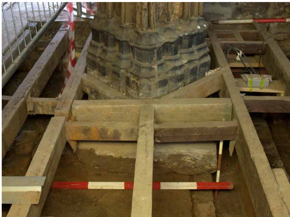
Plate 5: Detail of the Spere Post, with sandstone pad below
