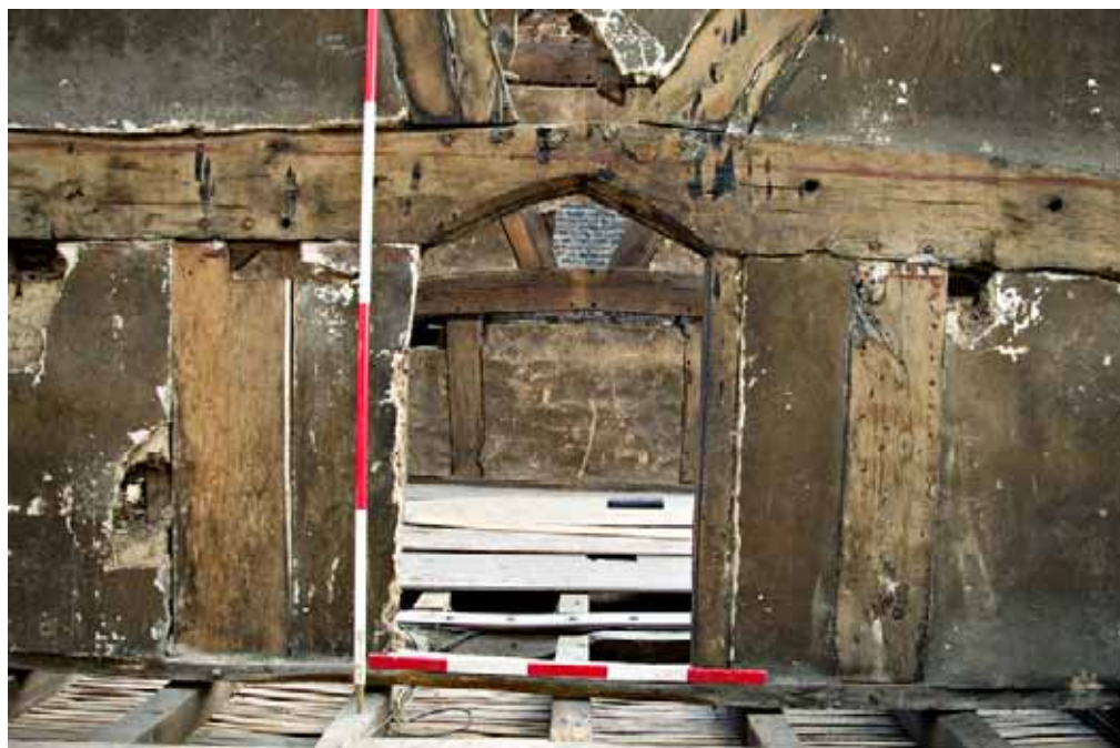
Plate 37: Detail of truss within Room S9, showing pegged assembly
