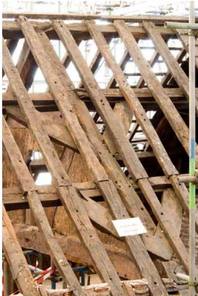
Plate 71: Simple splayed scarf joint in ridge purlin above truss, Roof J
