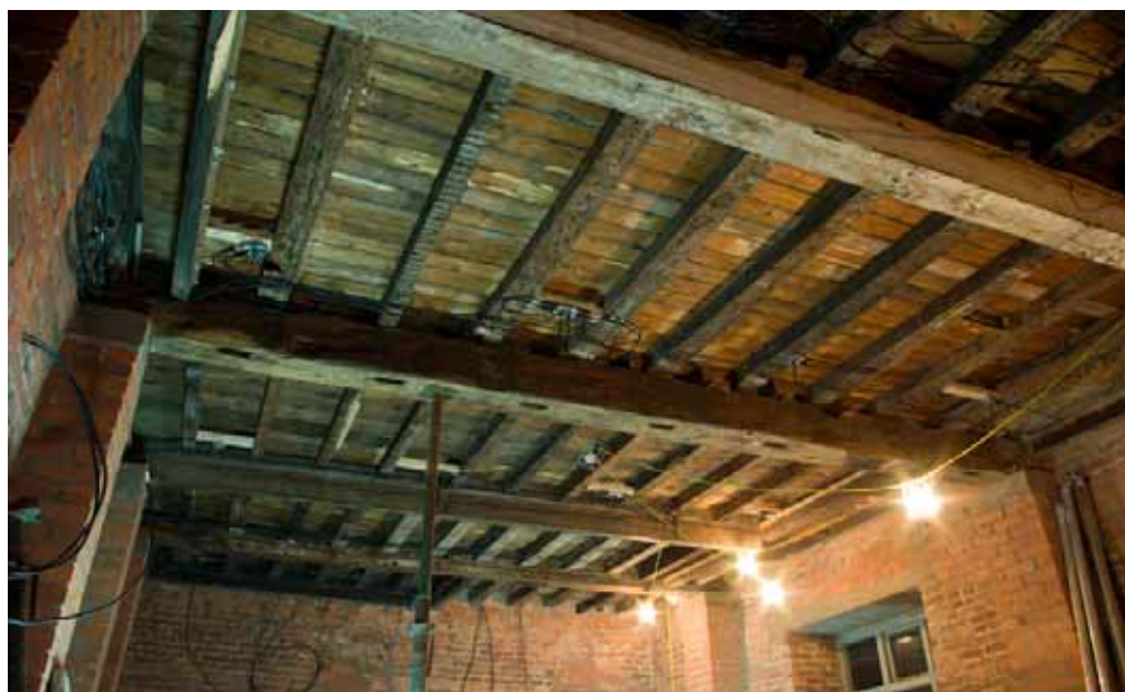
Plate 17: Ceiling within the Radclyffe Room (G11B), showing re-used beams
