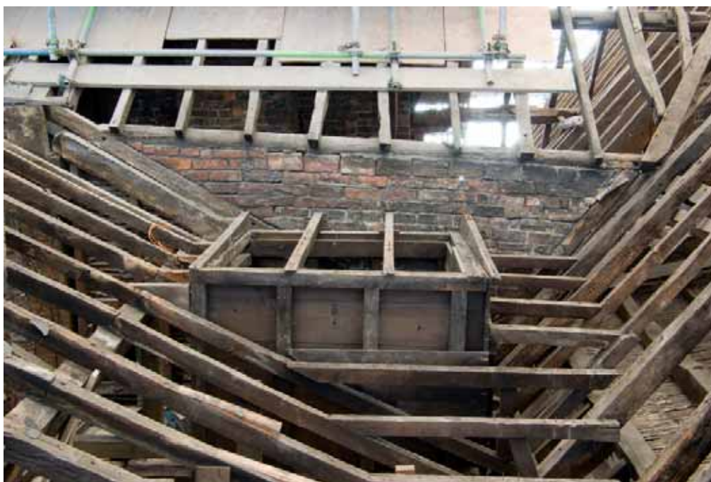
Plate 45: Timber water tank between Roofs B (left) and C (right)
