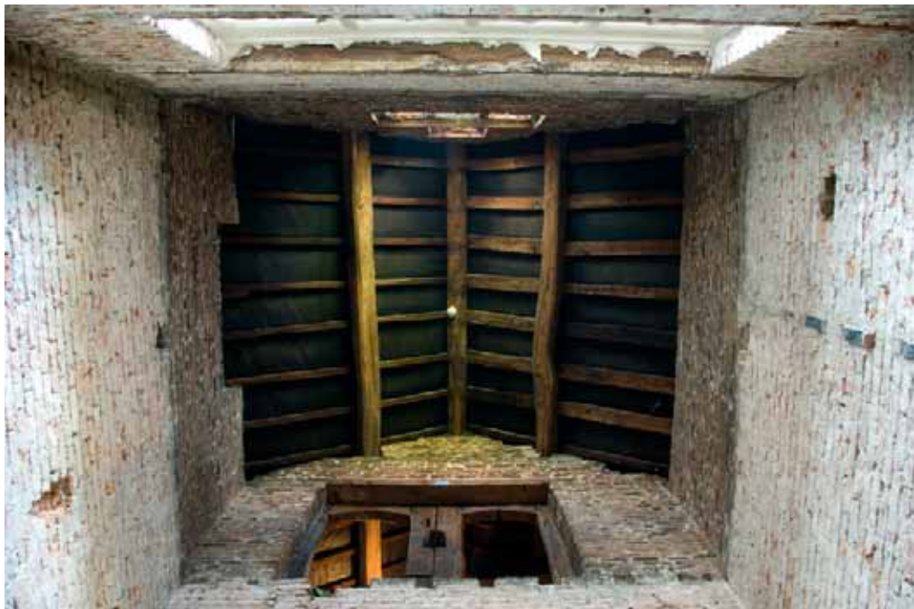
Plate 25: Timber-framed doorway to second floor, with roof detail above
