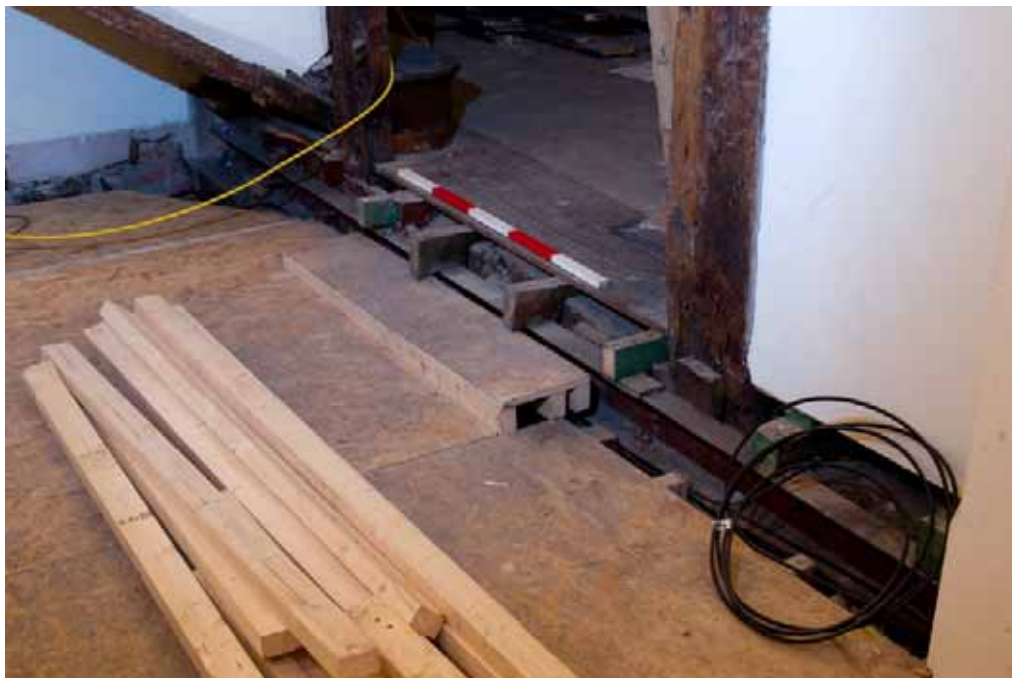
Plate 35: Steel beam inserted to support wall frame and floor
