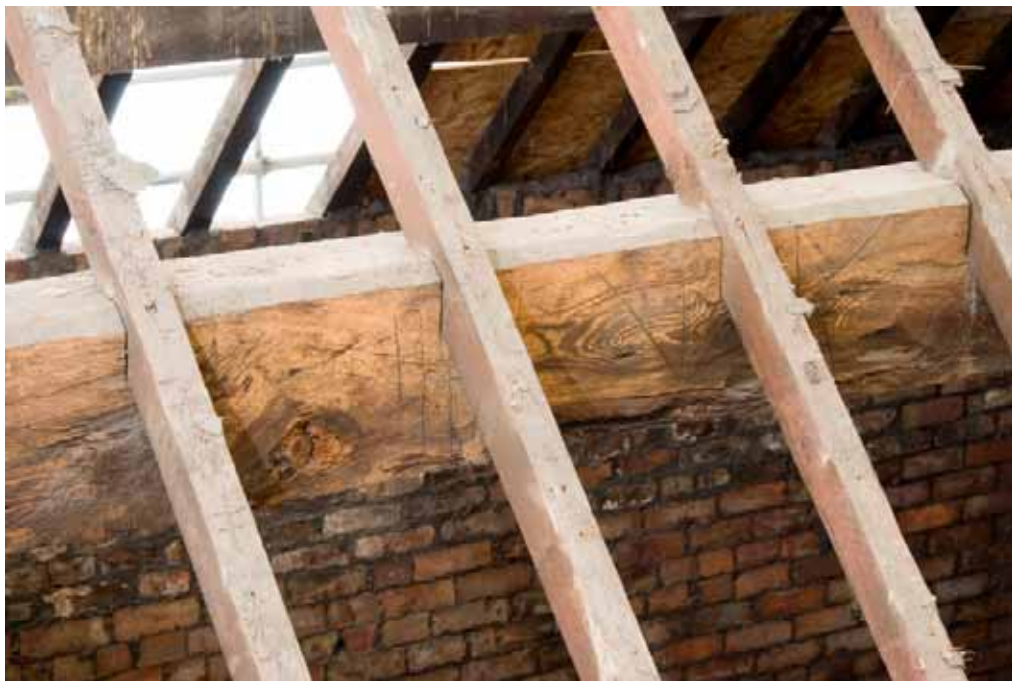
Plate 69: Baltic shipping marks on eastern purlin, Roof I
