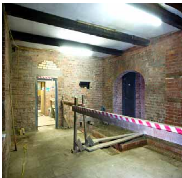
Plate 13: View of the Kitchen (G10), showing flue aperture and re-modelled doorway
