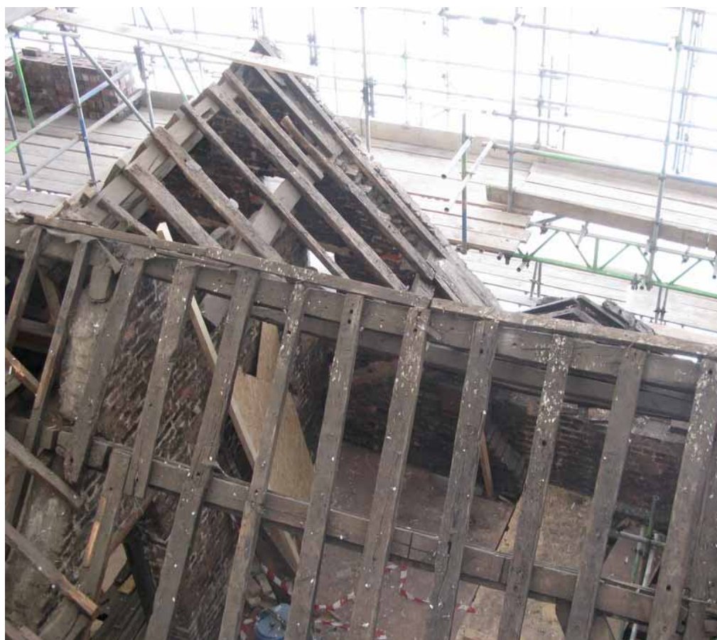
Plate 73: Small pitched gable of western tower (Roof K)
