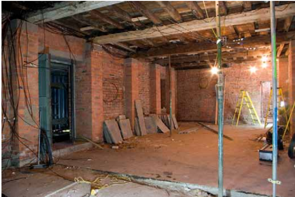
Plate 16: General aspect of the Radclyffe Room (G11B), with inserted piers and doorway
