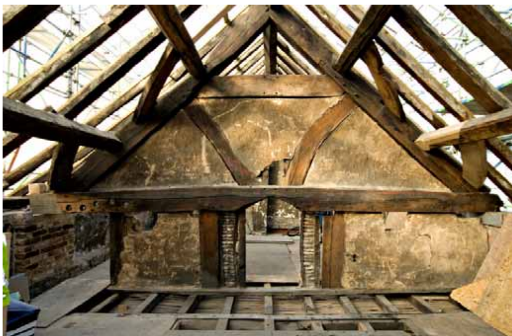
Plate 41: Lower face of northern truss of west wing, with remodelled doorway
