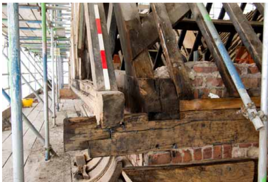
Plate 65: Repositioned truss and scarf-jointed wall-plate, southern gable, Roof F
