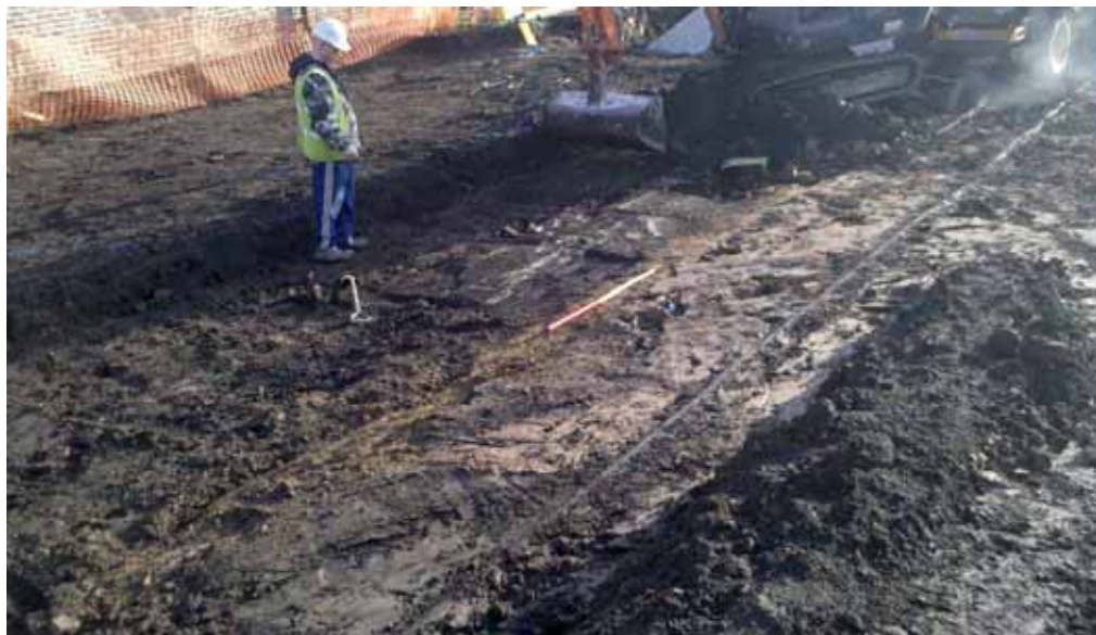
Plate 85: Working shot showing sandstone flags adjacent to wall 2
