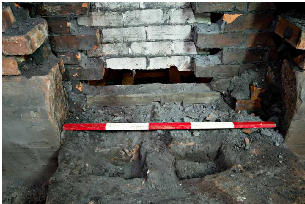
Plate 10: Removed section of Plinth, external south wall of Great Hall (G4)
