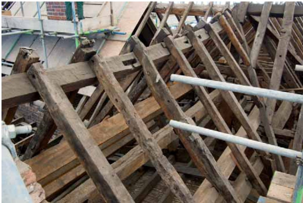
Plate 52: Re-used ridge purlin and common rafters, northern part of Roof C
