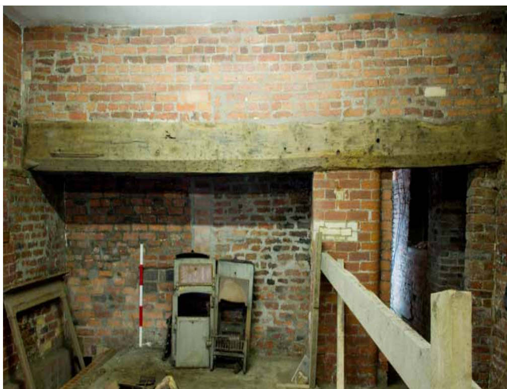
Plate 15: Inglenook fireplace in the Kitchen (G10)
