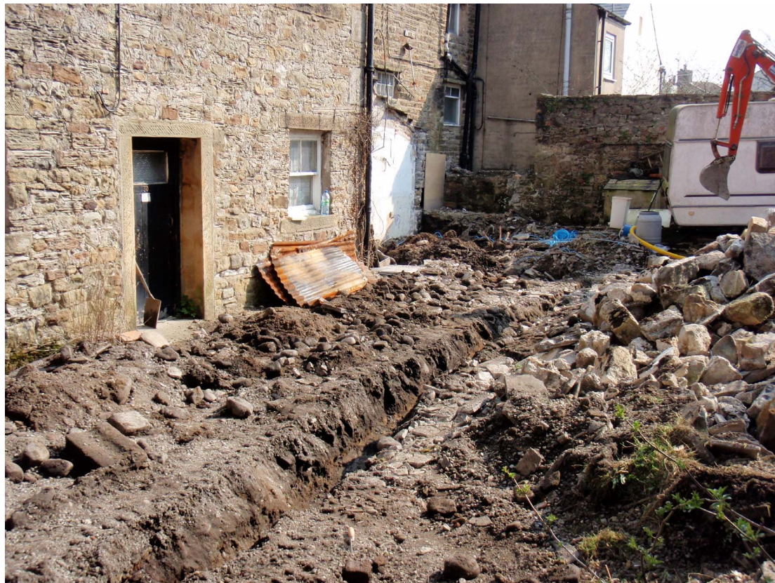
Plate 1: the rear of 29 Church Street during excavation
