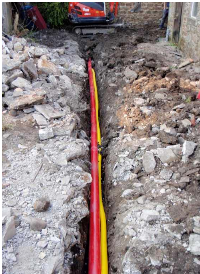
Plate 2: the rear of 29 Church Street after excavation
