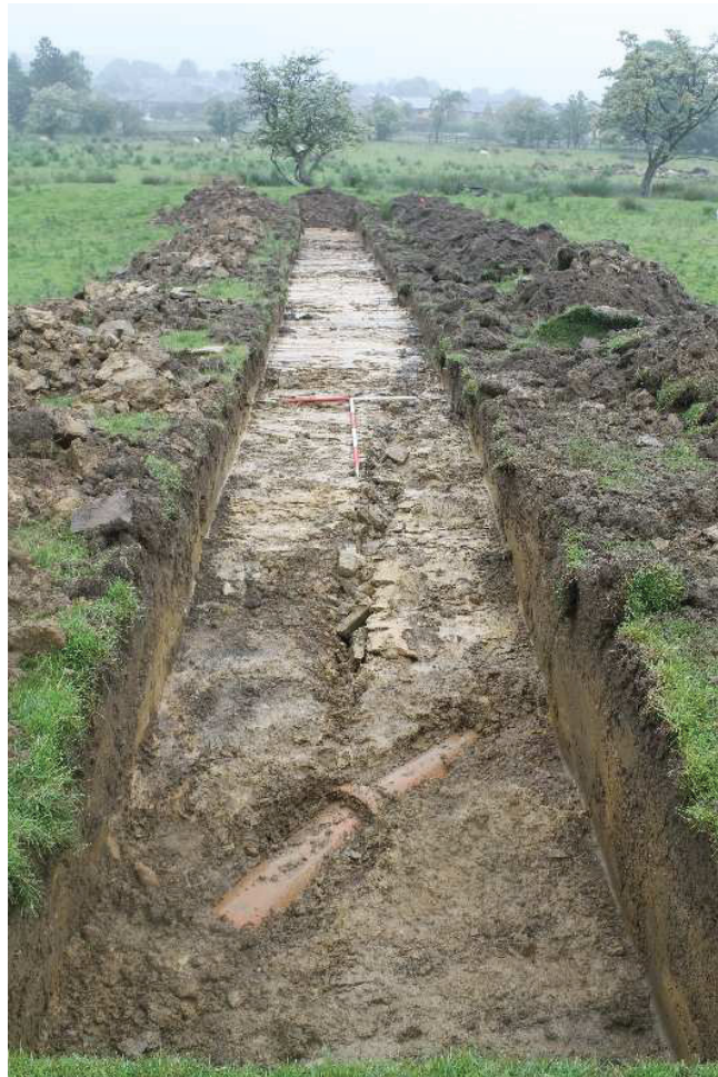
Plate 24: Trench 16, facing north
