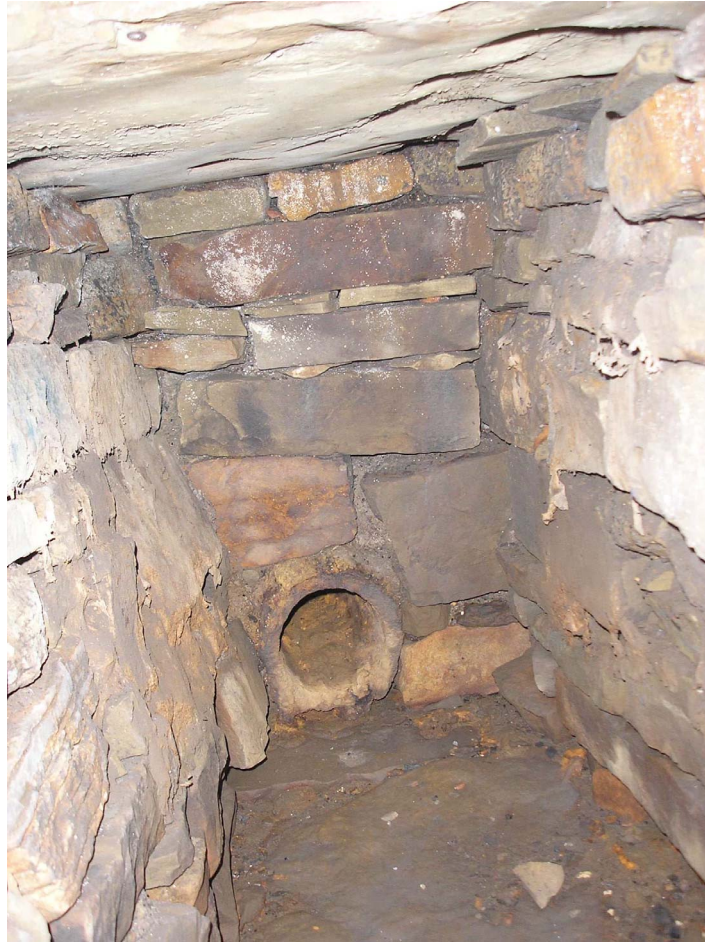
Plate 8: Culvert in Test Pit 2
