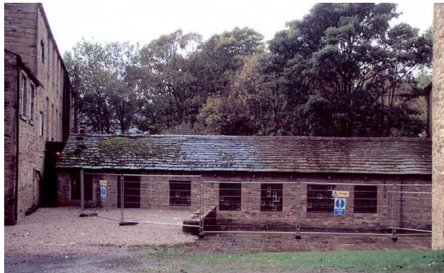
Plate 3: Looking west across site of boiler house
