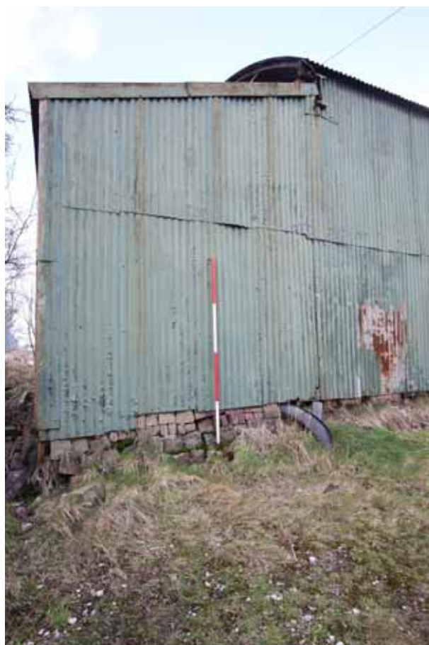
Plate 20: View of the south-east facing elevation of the rear extension, showing the made up ground level bricks
