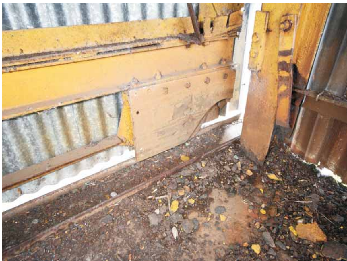
Plate 14: Sliding door mechanism, showing the roller in place on the rail
