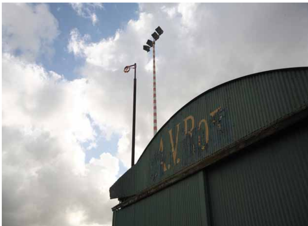
Plate 4: View of the flood light located to the south of the Avro Shed and the wind sock pole fixed to the south-east corner of the Shed
