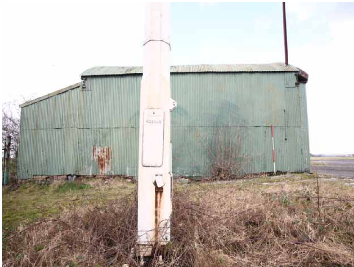
Plate 19: South-east facing elevation showing extension to the rear
