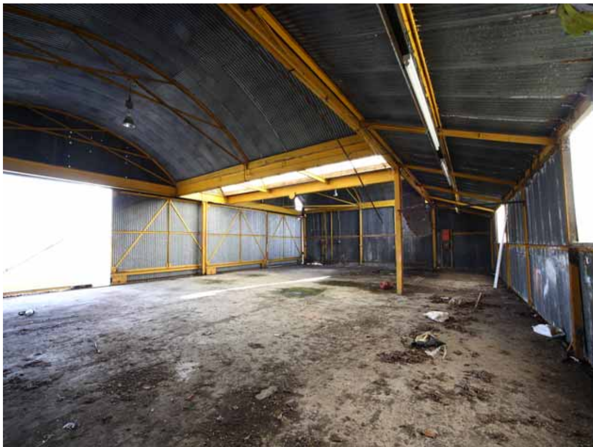
Plate 31: View south-east of the main Shed, Room 1
