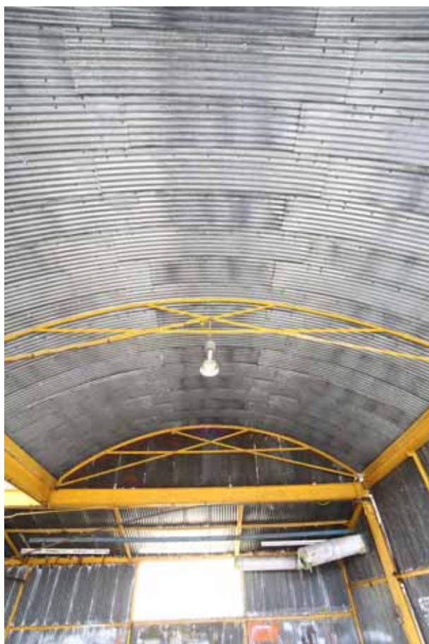
Plate 32: West view of trusses in north barrel vaulted roof
