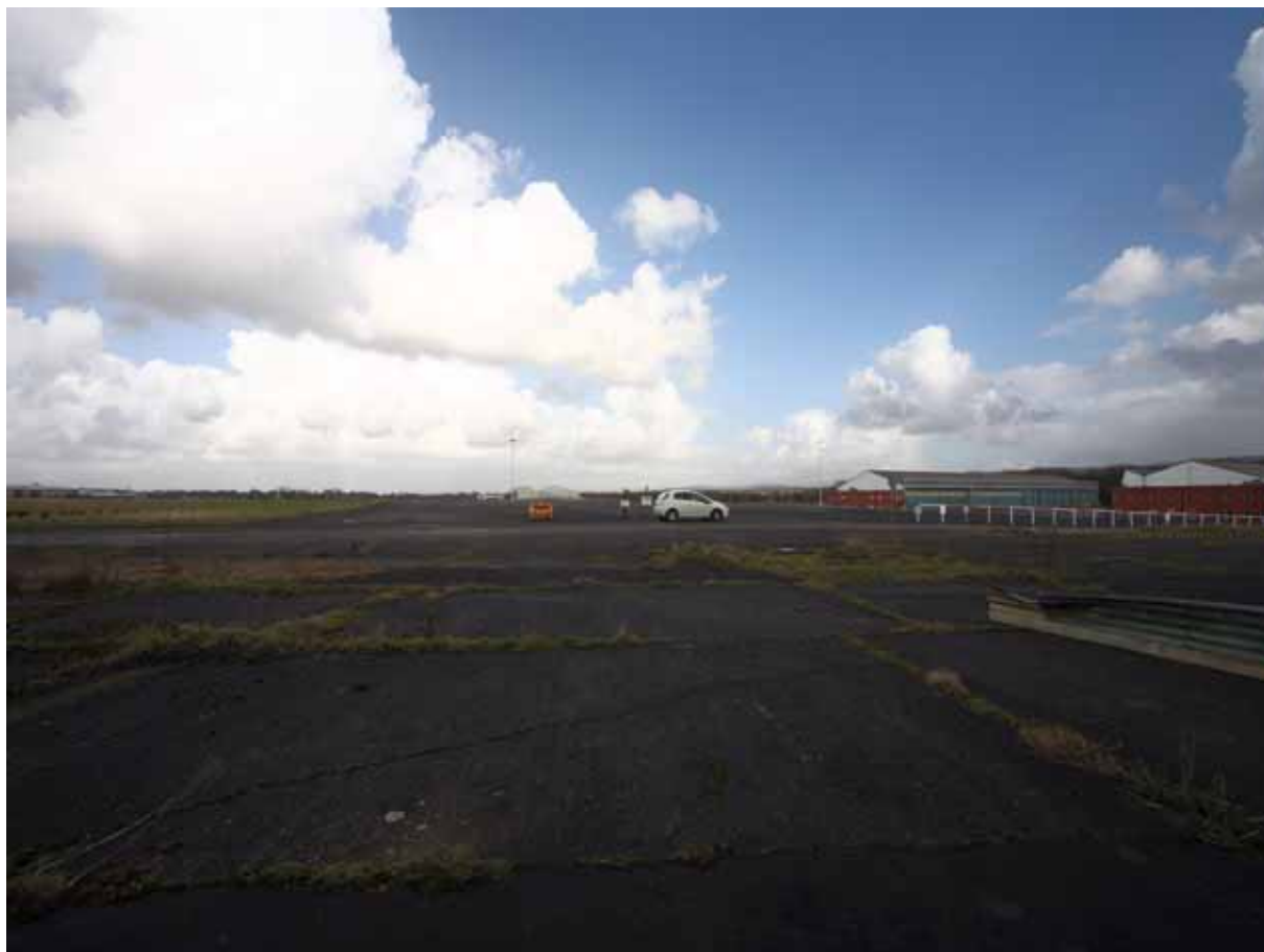
Plate 1: View north-east from the Avro Shed and workshop looking across the airfield
