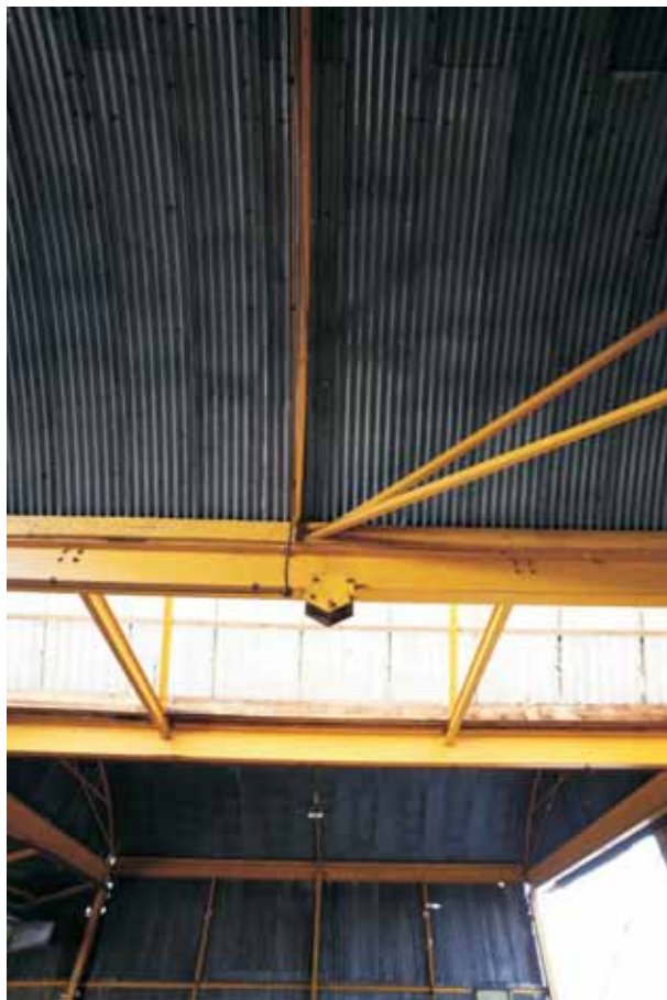
Plate 38: Sliding pulley bracket
