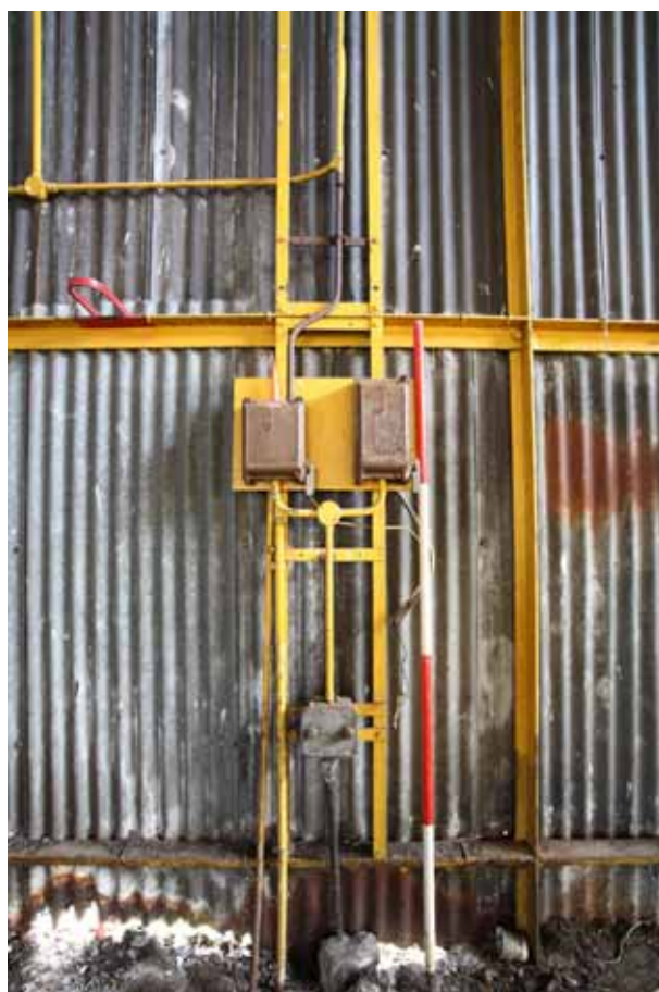
Plate 34: Electrical switches and trunking visible on south elevation, Room 1
