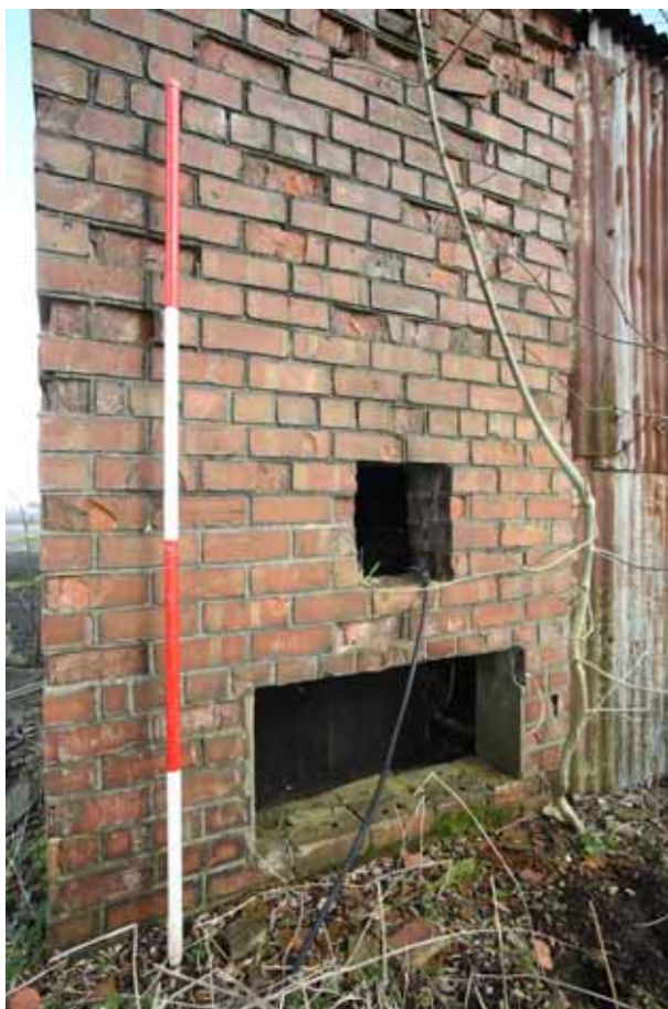
Plate 23: Apertures in south-west facing elevation of brick outshut
