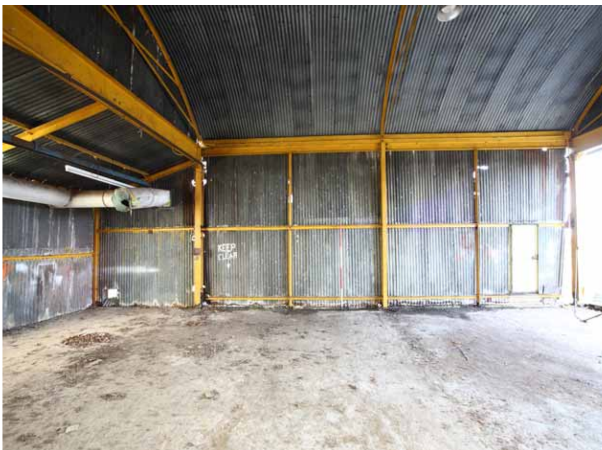
Plate 30: Internal view of north-west facing elevation
