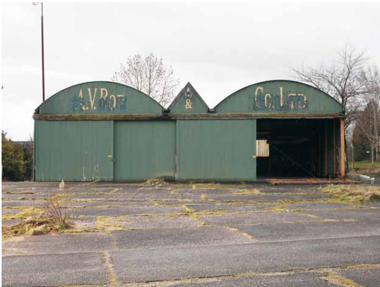
Plate 9: Principal north-east facing elevation of the Avro Shed
