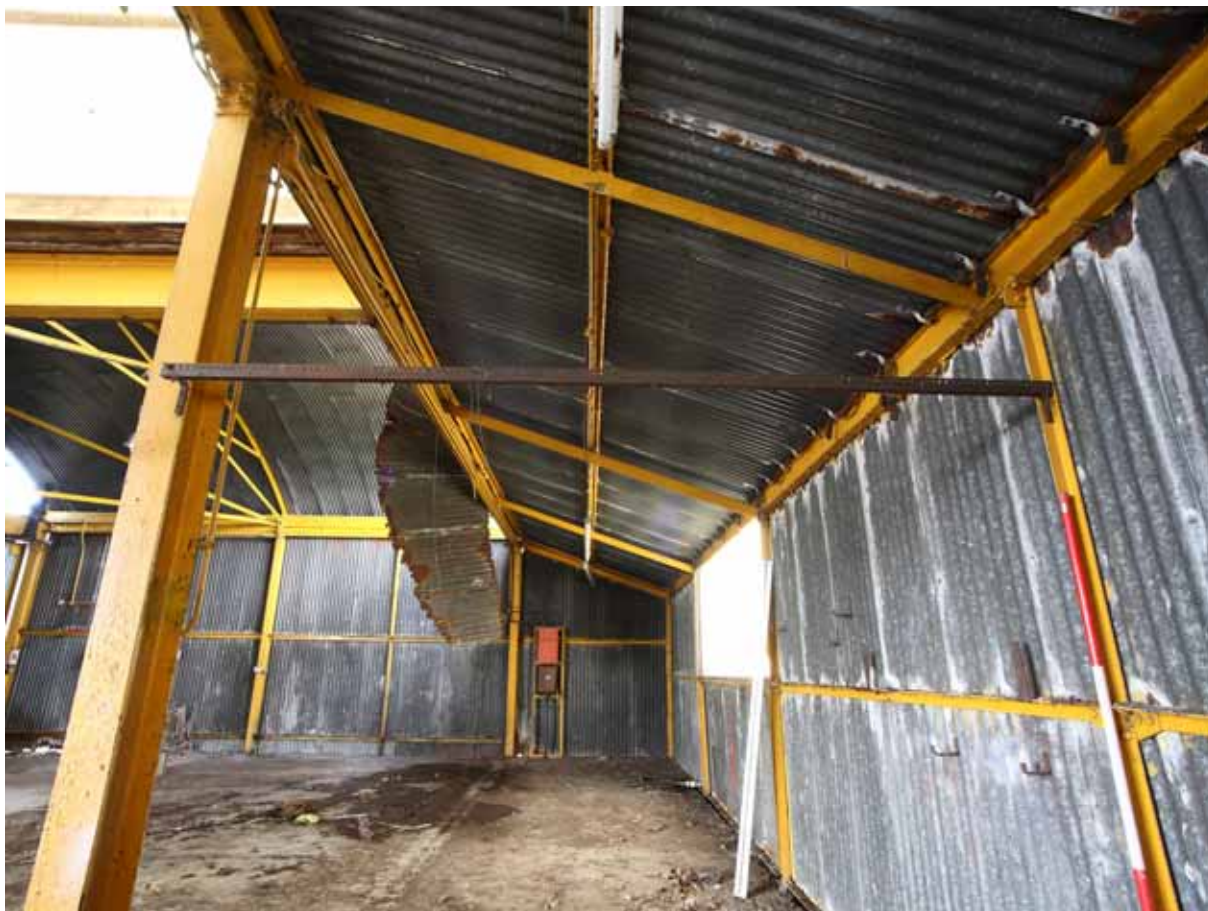
Plate 29: View south along the extension of the Shed, Room 1
