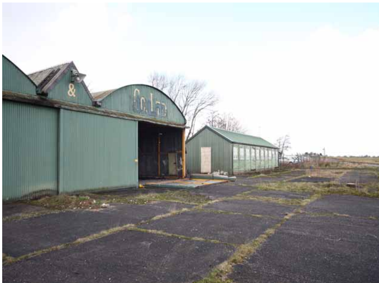
Plate 3: Green workshop north-west of the Avro Shed
