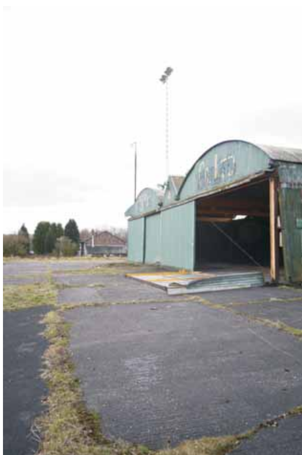
Plate 16: View of the north-east corner of the Shed
