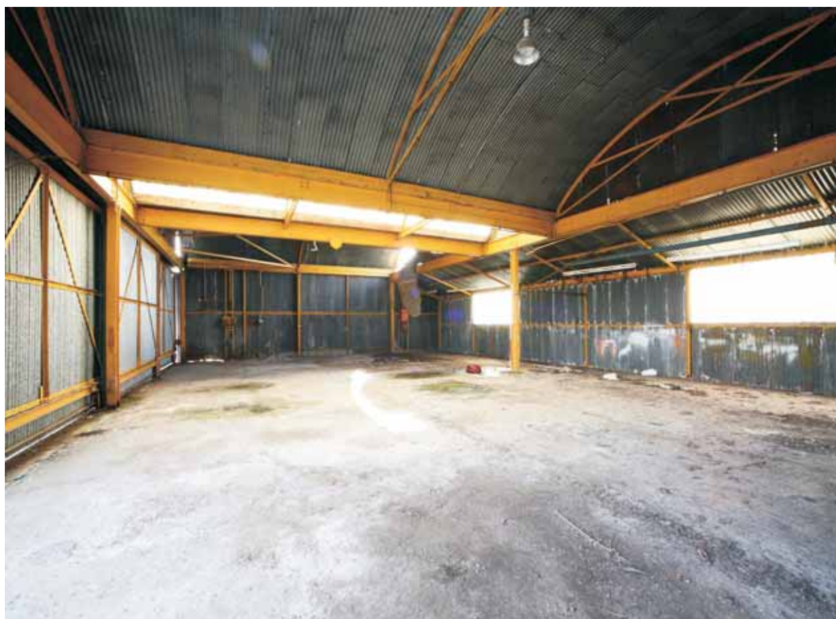
Plate 12: View through the building, facing south-west showing the internal structural frame
