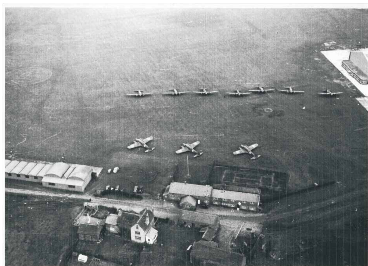
Plate 8: North-east facing view showing the Avro Shed and stores
