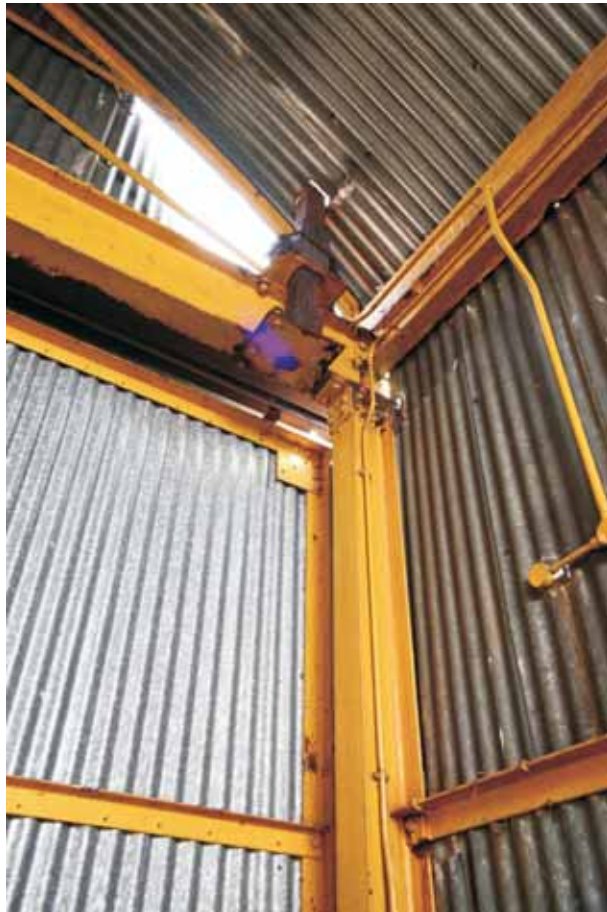
Plate 37: Bracket fitted internally for the wind sock
