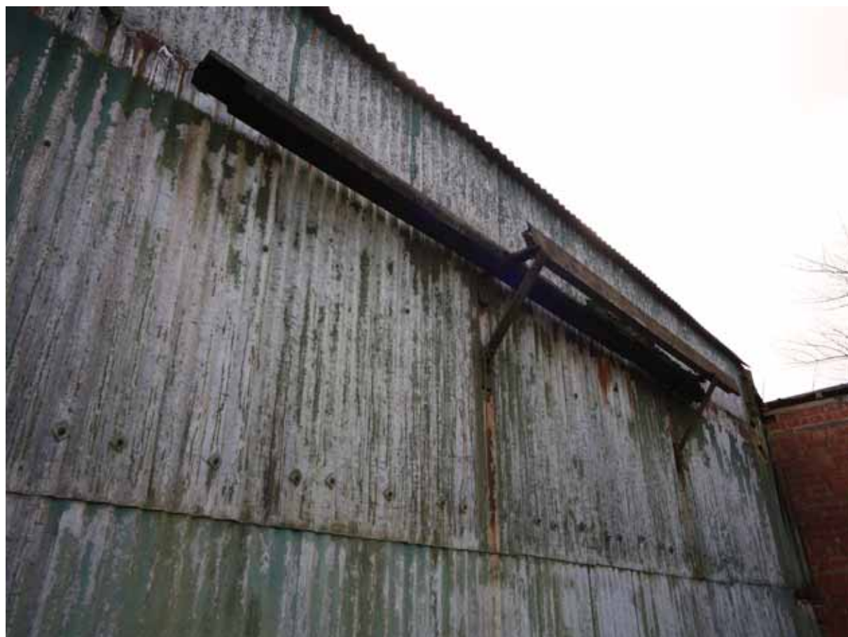
Plate 26: View of the brackets fixed to the north-west facing elevation
