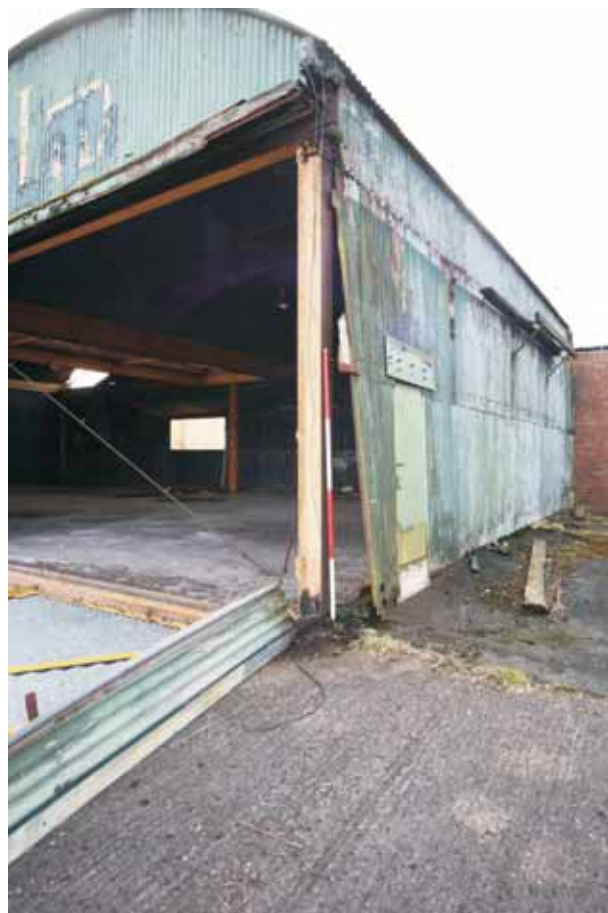
Plate 11: Additional access on the north-west facing elevation
