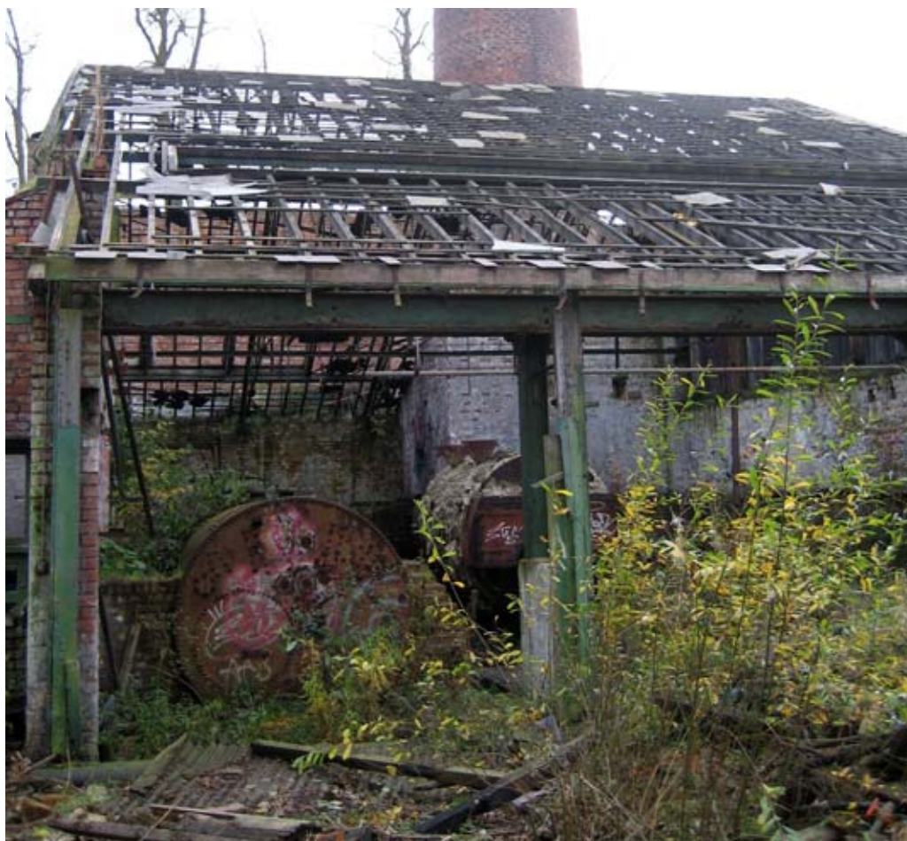
Plate 18: North-facing elevation of Building 8, showing in-situ Lancashire boiler
