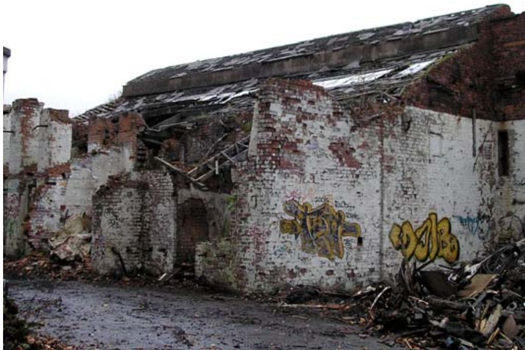
Plate 24: West- and south-facing elevations of Buildings 15 - 17
