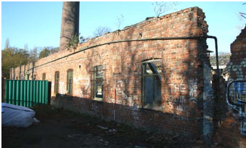
Plate 16: North-west-facing view of the south elevation of Building 7
