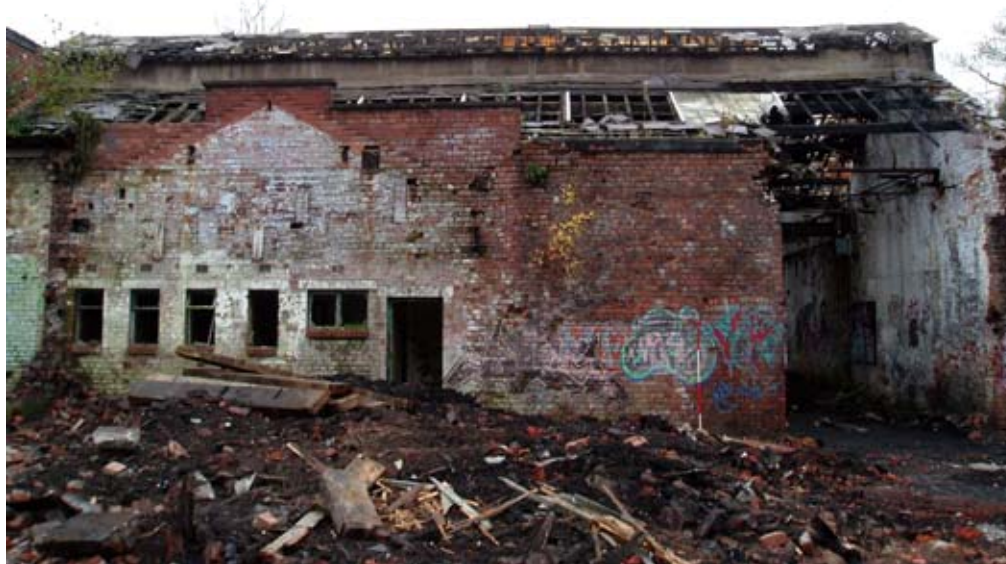
Plate 20: Scars of Building 11 visible on the east-facing elevation of Building 13
