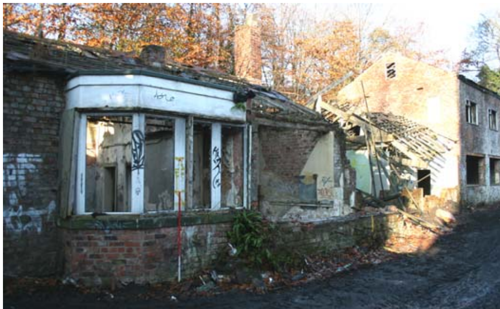
Plate 10: North-west-facing view of the east elevation of Building 1
