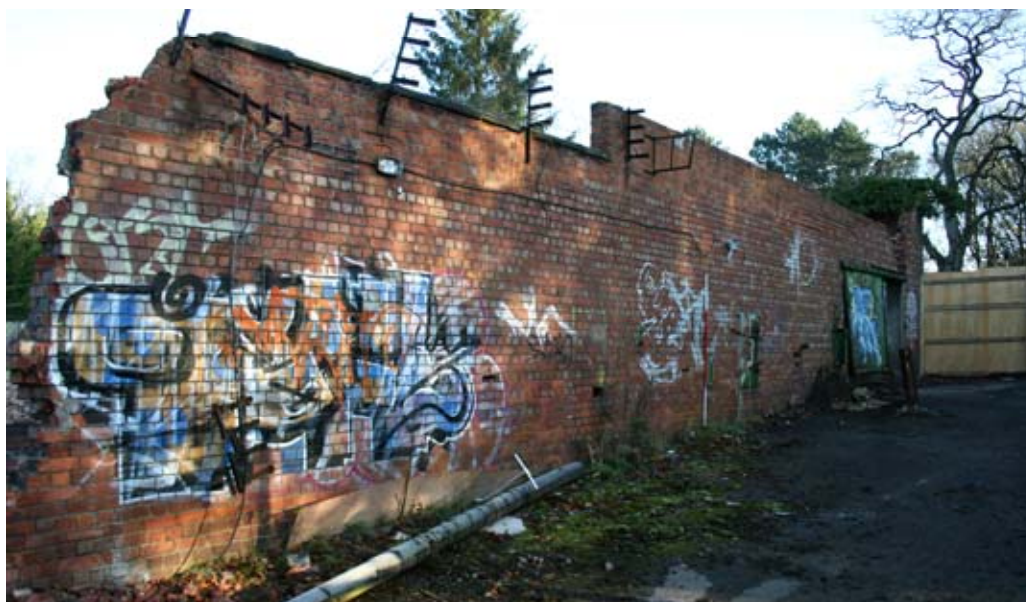
Plate 17: North-east-facing view of the south elevation of Building 9
