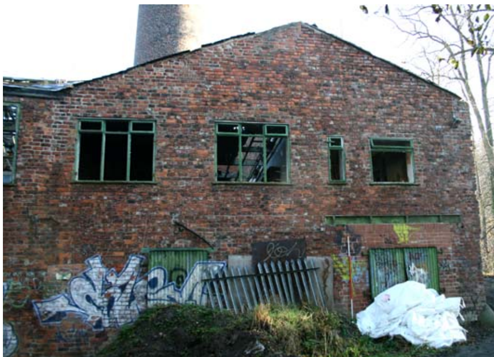
Plate 15: East-facing view of the west-elevation of Building 6
