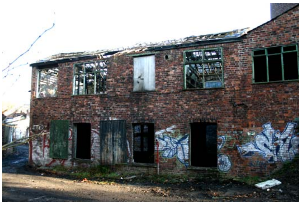
Plate 14: East-facing view of the west elevation of Building 5
