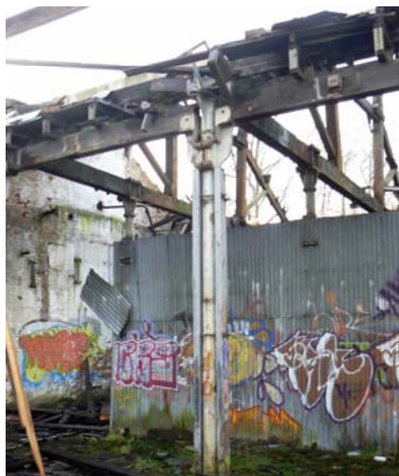
Plate 22: Columns within Building 13
