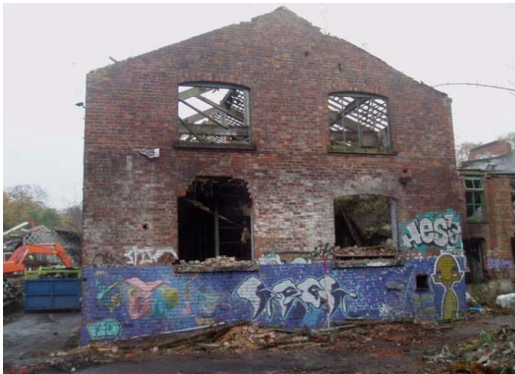
Plate 12: South-facing view of the north elevation of Building 4
