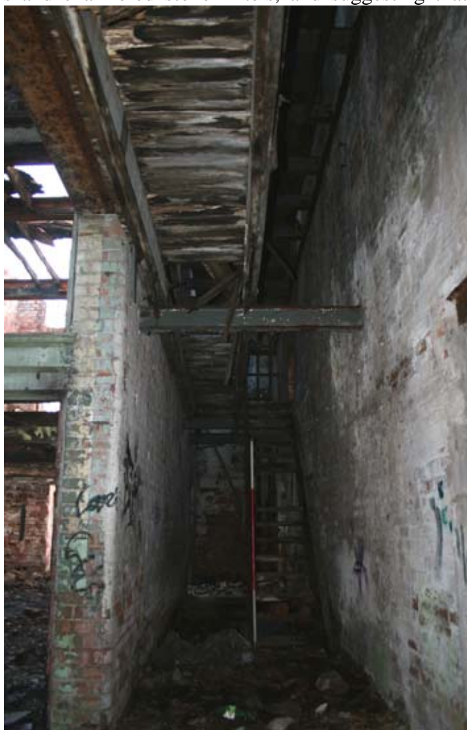
Plate 23: The Chemic Mixing and Starch Room (Building 14)
