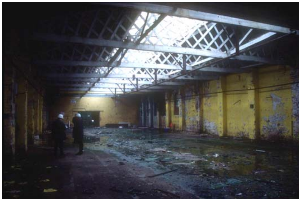
Plate 25: Interior of Building 19, taken in 1999 (reproduced courtesy of GMAU)
