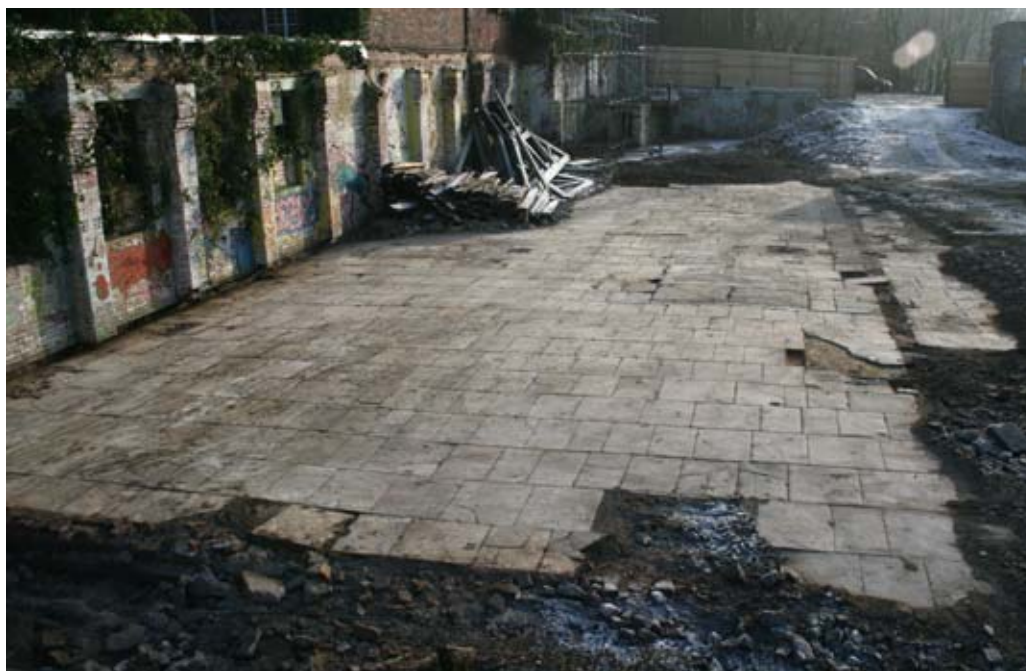
Plate 32: Flagstone floor exposed beneath concrete in Building 19, looking south
