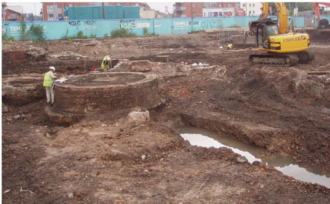
Plate 45: Late circular brick structures, looking north-east
