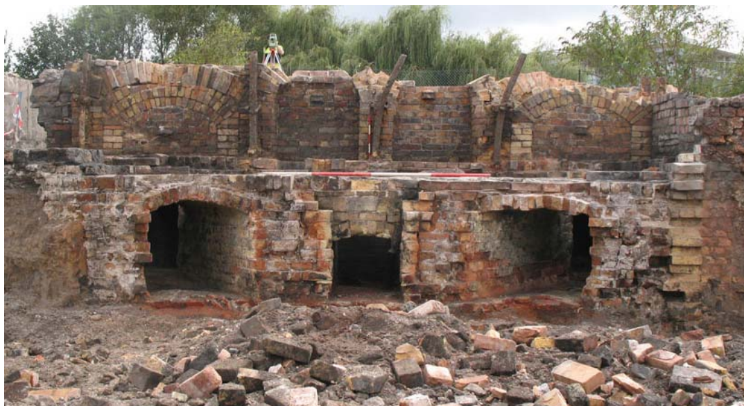
Plate 29: Elevations of flues in Furnace C, looking south
