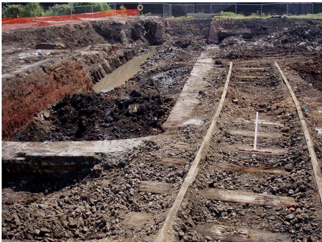
Plate 43: The north end of dock 1003 , with railway tracks adjacent, looking south
