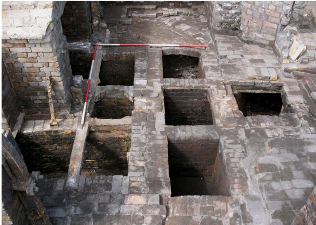
Plate 31: Furnace D, arrangement of access pits in switch room 3506, looking west
