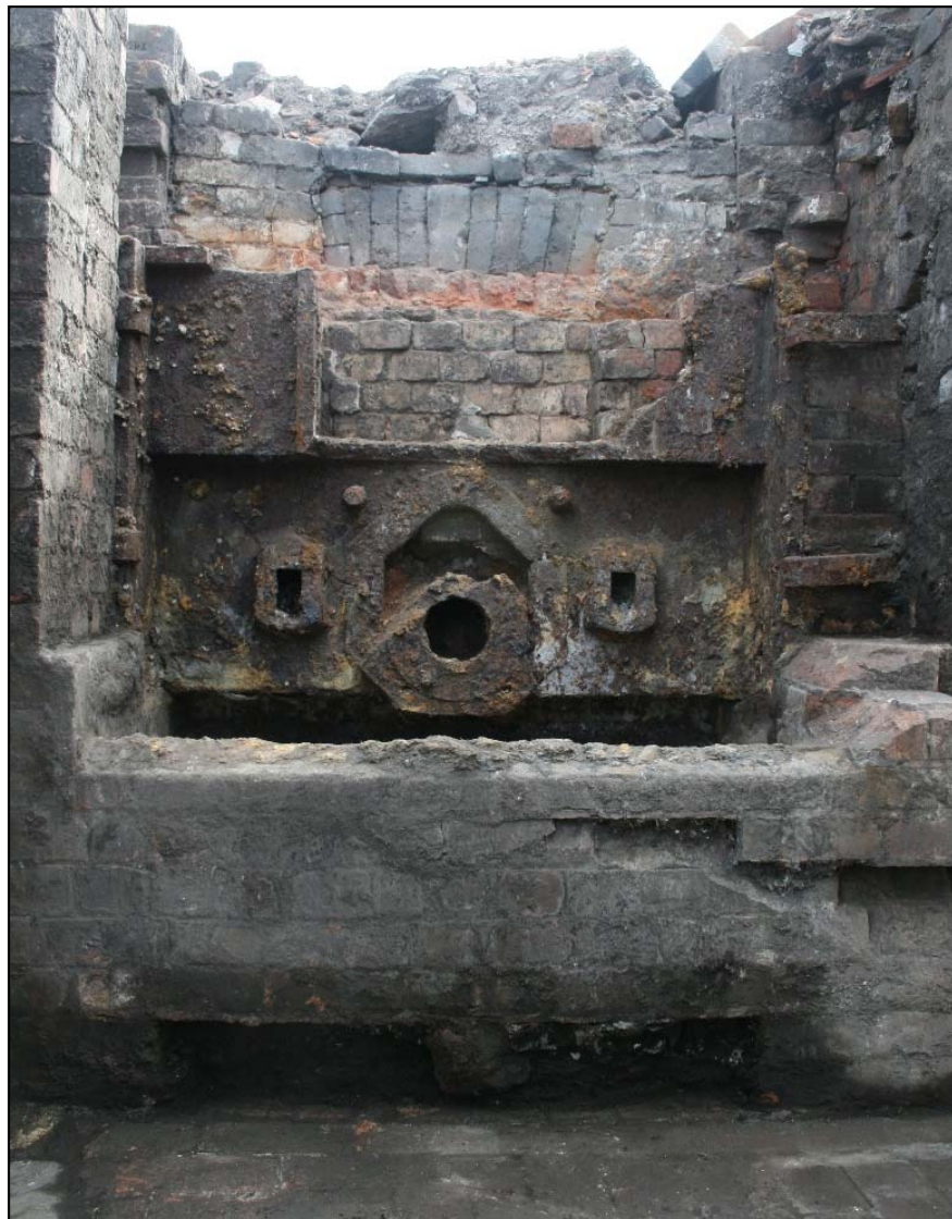
Plate 34: Detail of gas producer 3709 , face-plate elevation
