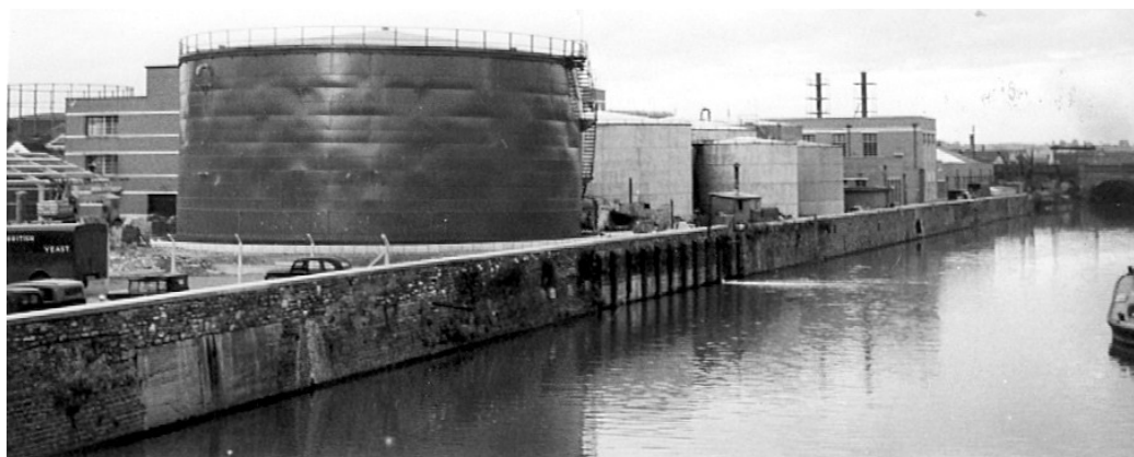
Plate 17: View of the open-area excavation site in c 1950, showing the yeast factory
