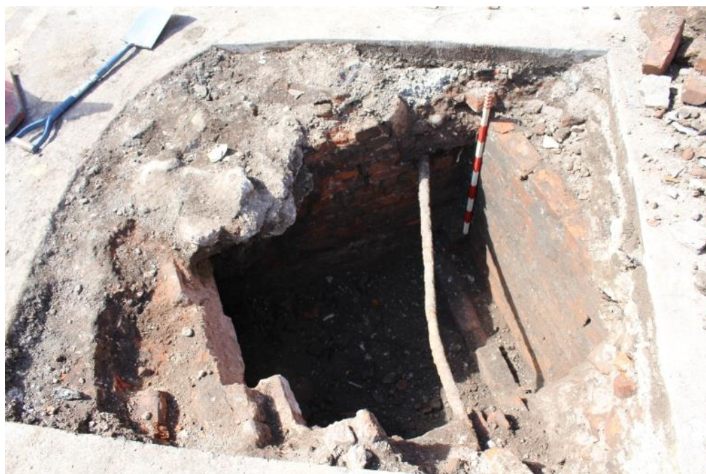
Plate 5: Trench 6, facing west, showing the brick-built cistern, which had a vaulted roof and had been backfilled with demolition rubble
