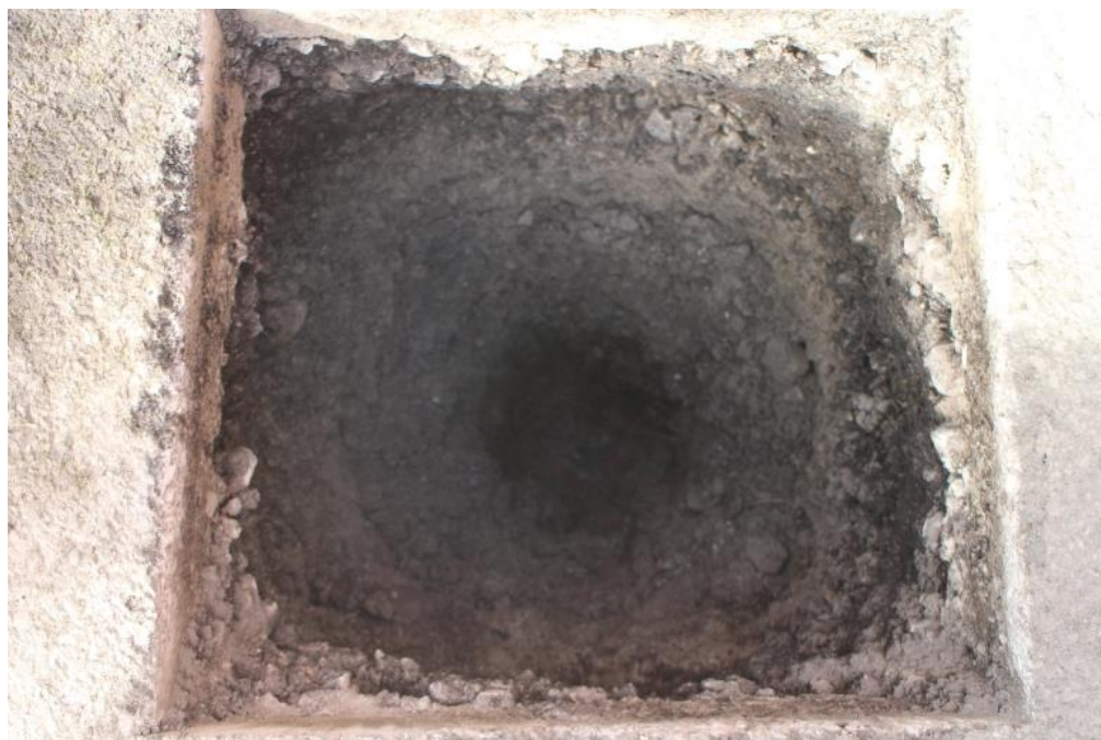
Plate 14: Borehole 19, Crook Street, to the rear of Goldsmith House, adjacent to the pavement
