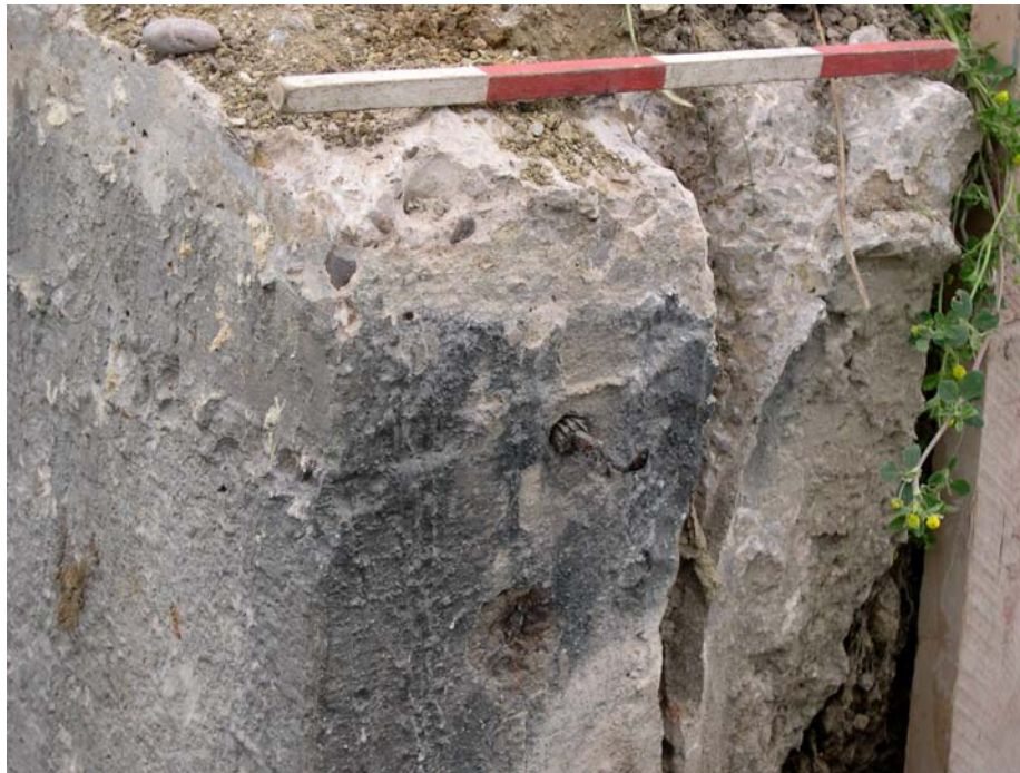
Plate 9: Hook for lighting festoon (Tunnel B)
