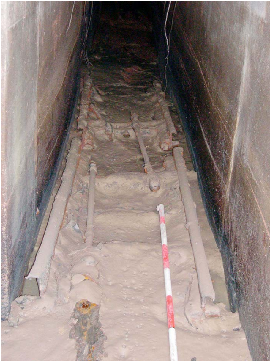
Plate 13: Railings within tunnel silt (Tunnel B)
