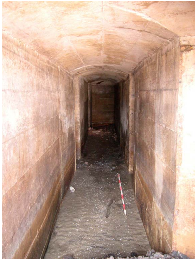
Plate 4: Tunnel C interior, showing construction markings (Tunnel C)
