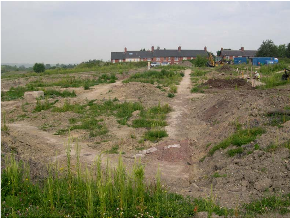
Plate 3: View from the east, showing the escape tower on Tunnel E3
