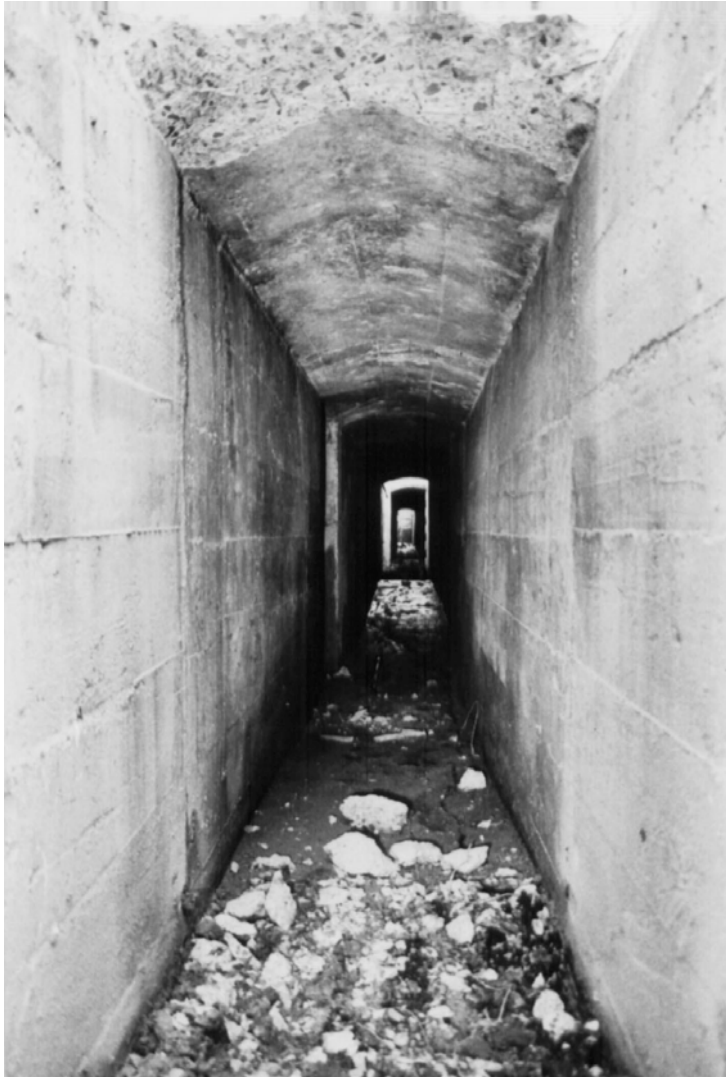
Plate 11: Longest tunnel (Tunnel B), looking west
