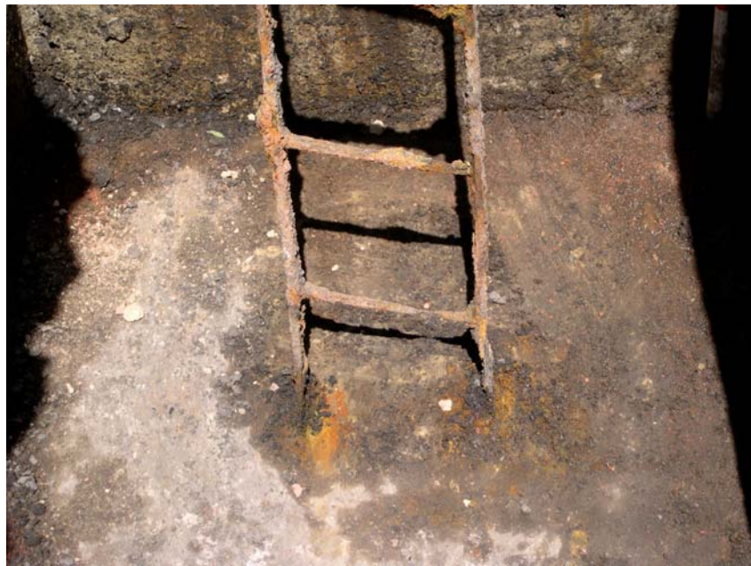
Plate 8: Base of ladder (Tunnel C)
