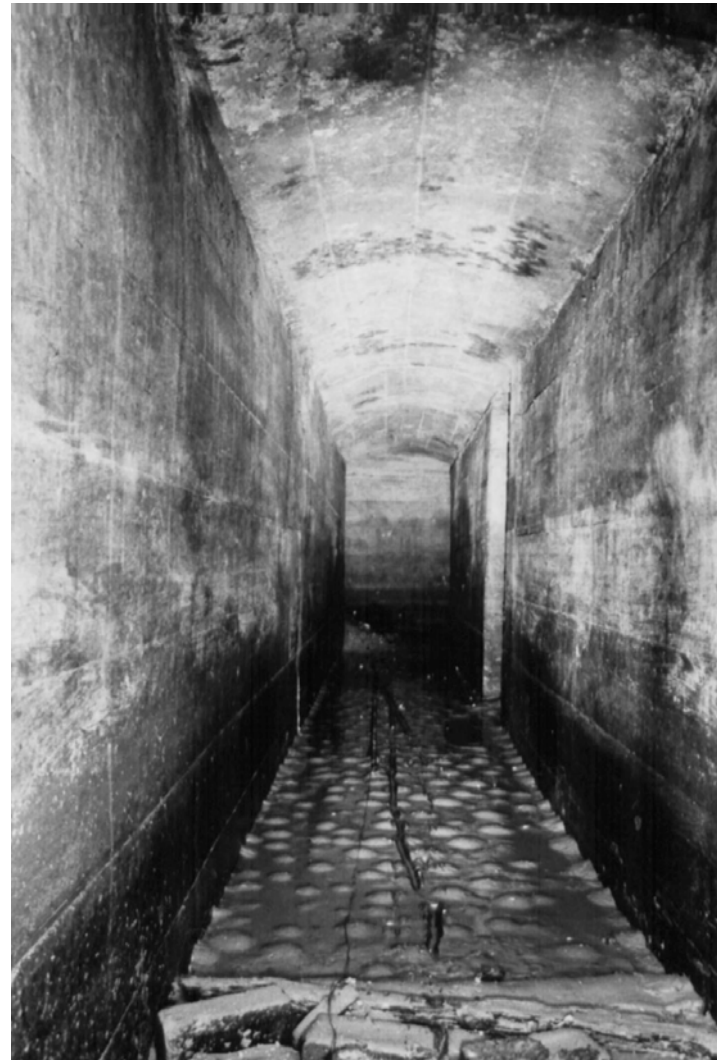
Plate 12: Undisturbed silt and pipe, looking south-west (Tunnel B1)
