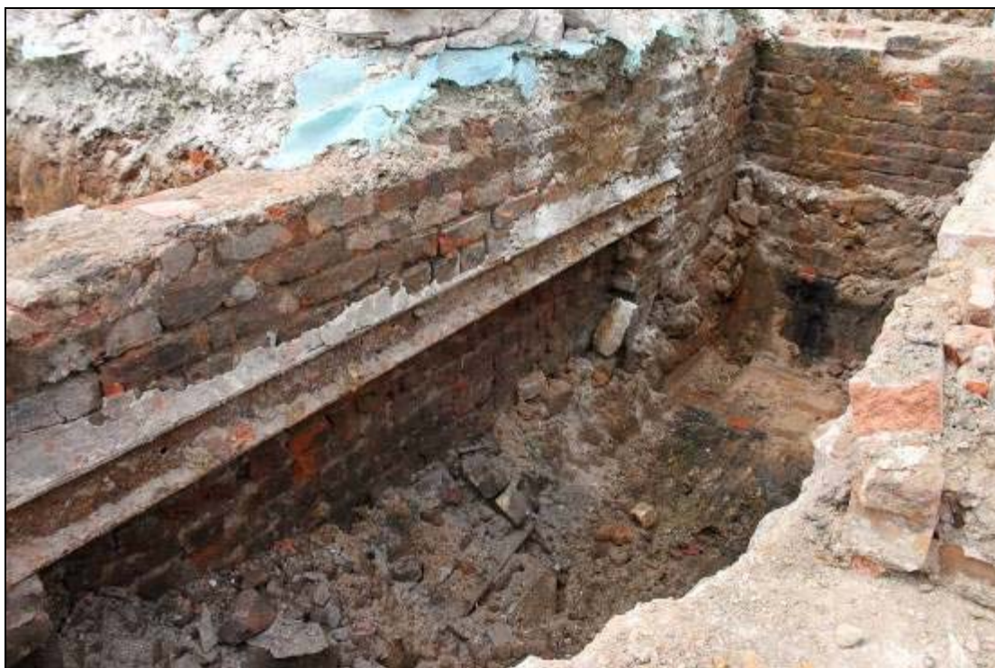
Plate 7: West wall of the boiler house, facing north-west
