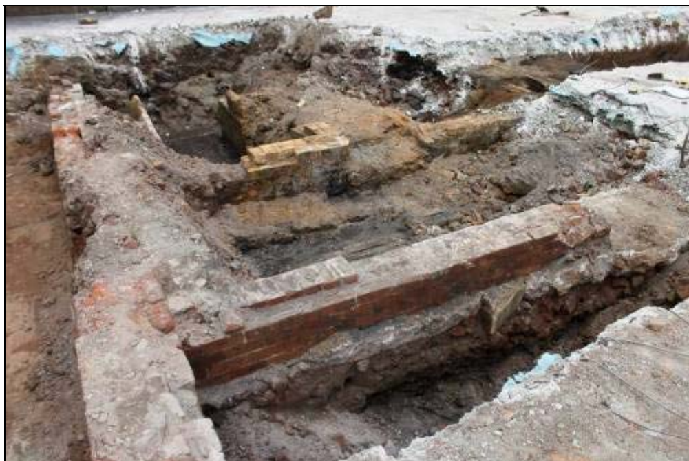
Plate 10: Western elevation of the mid-twentieth-century wall, facing south-east, with north wall of boiler house to left and boiler bays to rear
