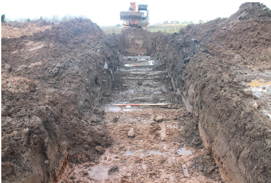
Plate 5: Machine-cut trench on the northern part of the site
