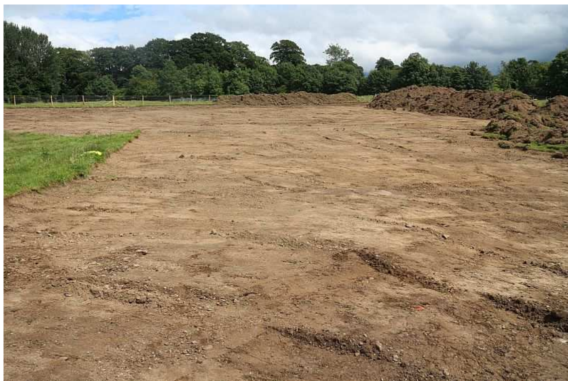
Plate 1: General view of the stripped compound and access track, facing south
