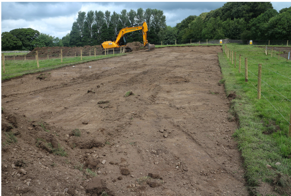
Plate 2: View of access track, facing north
