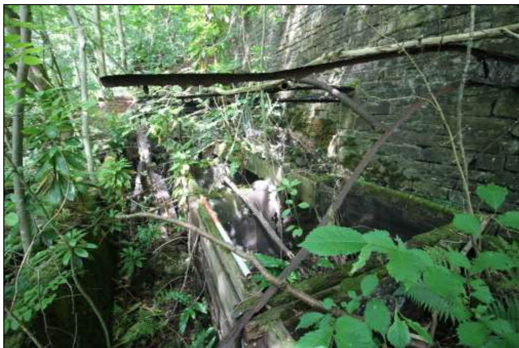
Plate 54: Timber tanks, facing north-west
