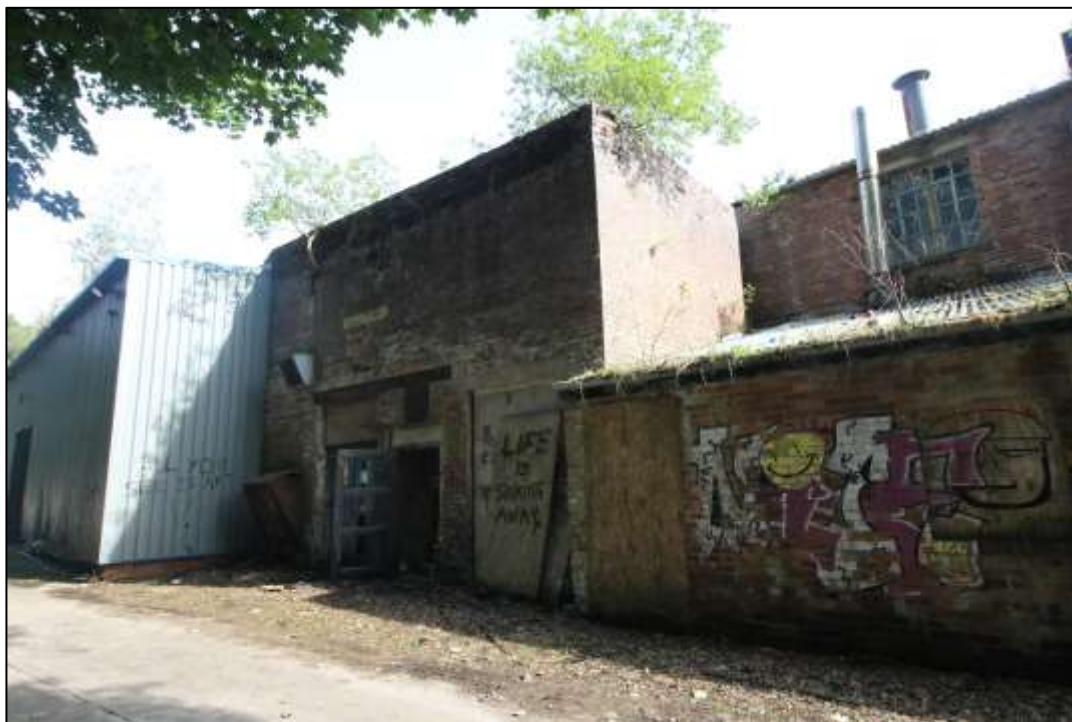
Plate 44: Engine house, facing north
