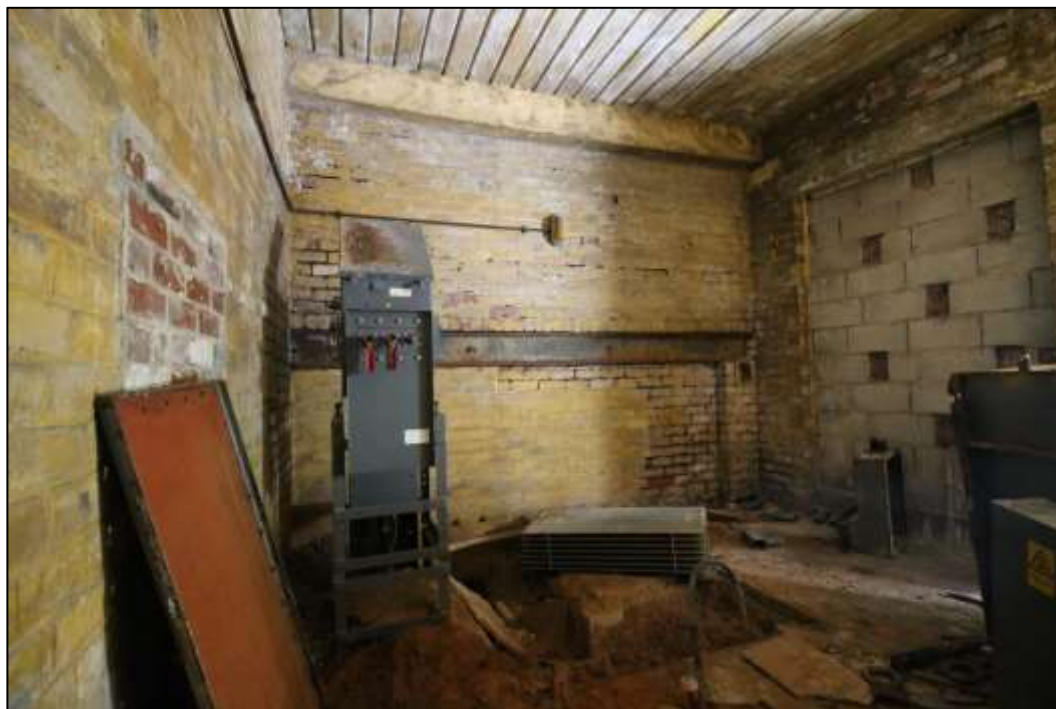
Plate 46: Interior of the smaller square cell, facing east
