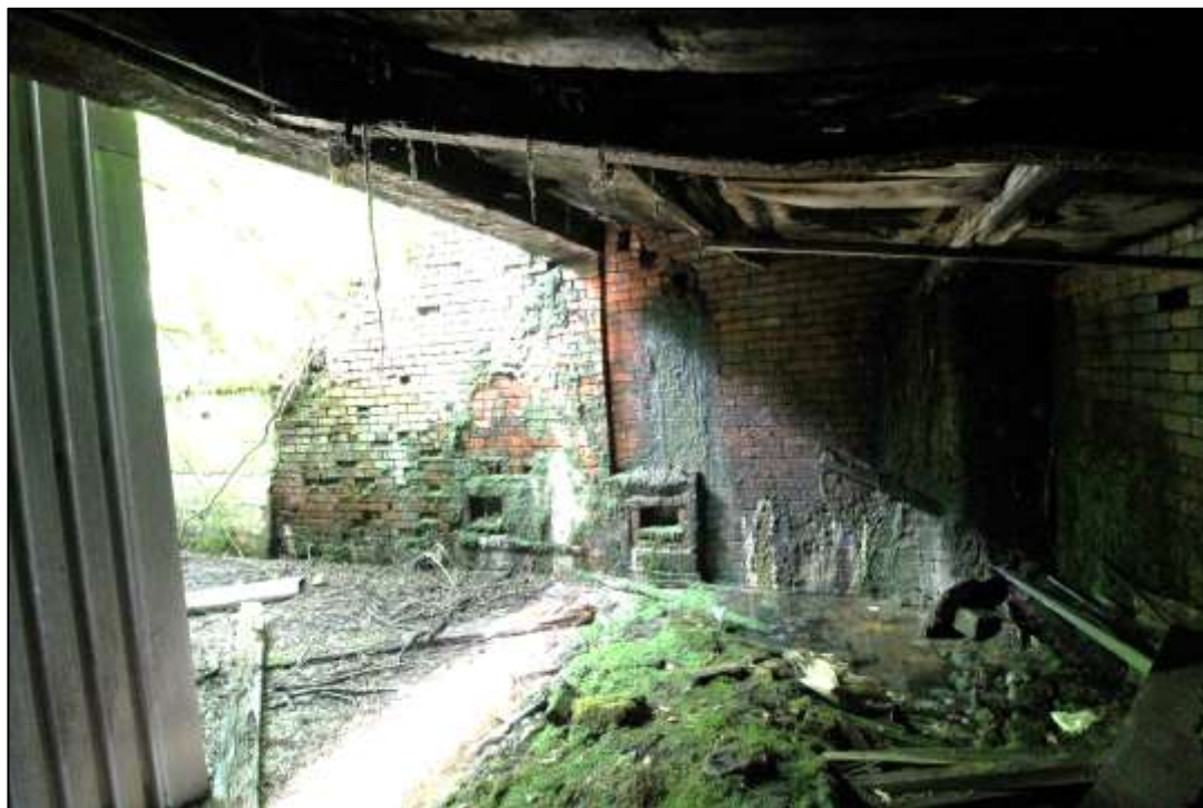
Plate 58: Open-sided brick-built structure, facing south-west
