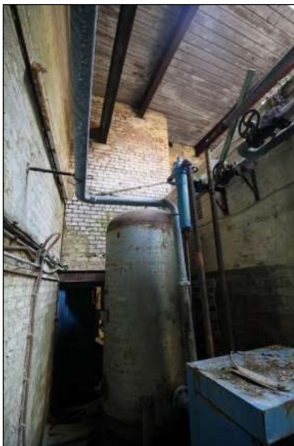
Plate 48: Circular tank in north-eastern corner of the larger cell
