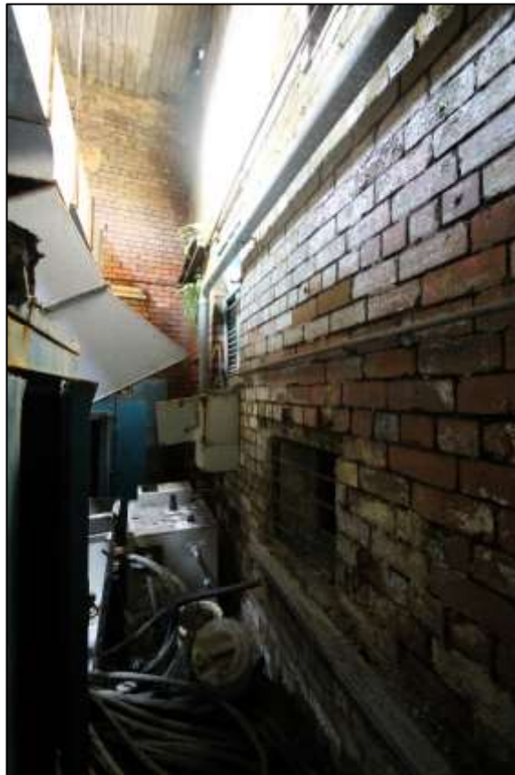
Plate 50: Western wall of the larger cell, showing blocked windows
