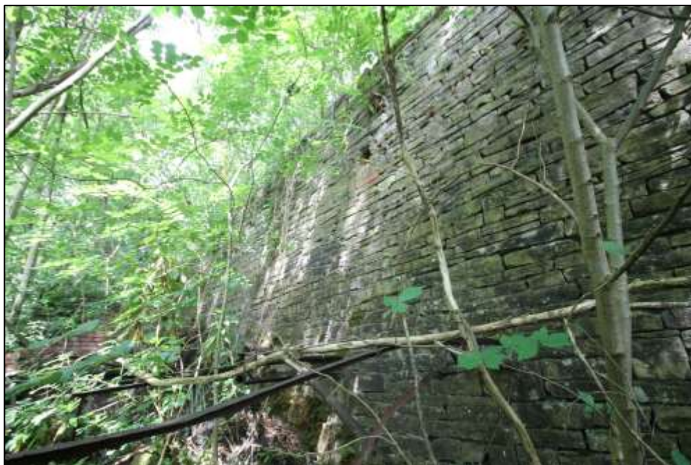
Plate 53: The early twentieth-century revetment wall
