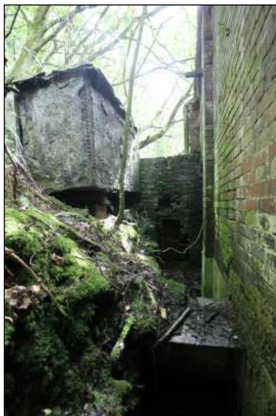
Plate 61: South-eastern end of narrow passage
