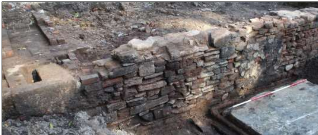
Plate 16: The large sandstone block (left) incorporated into the Phase 1 wall defining the northern bay of the mill/bleach works
