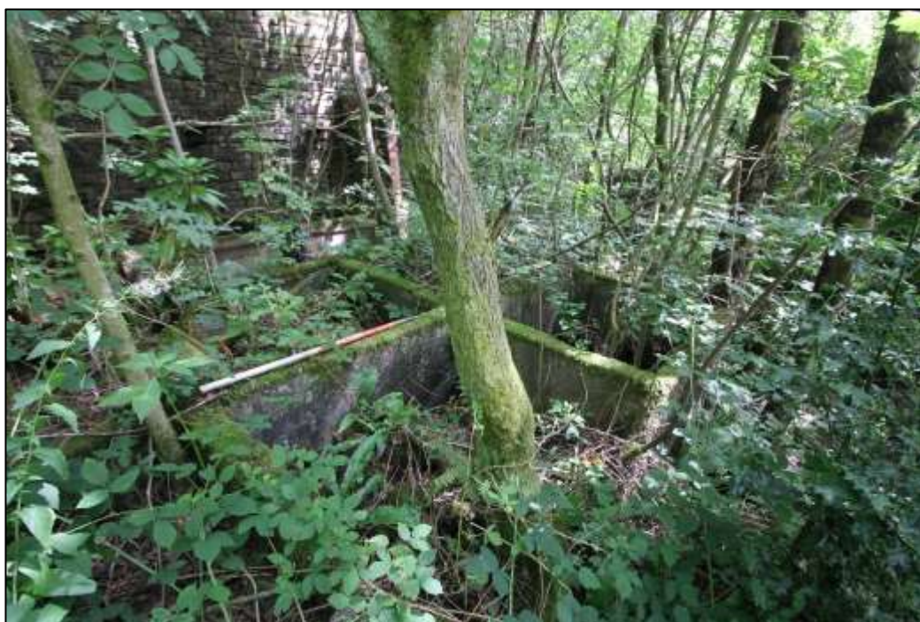
Plate 56: Concrete vats, facing east
