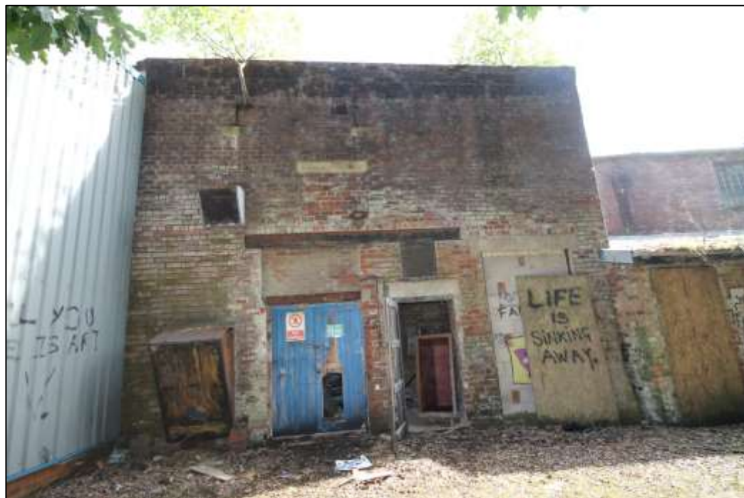
Plate 45: Southern elevation of the engine house
