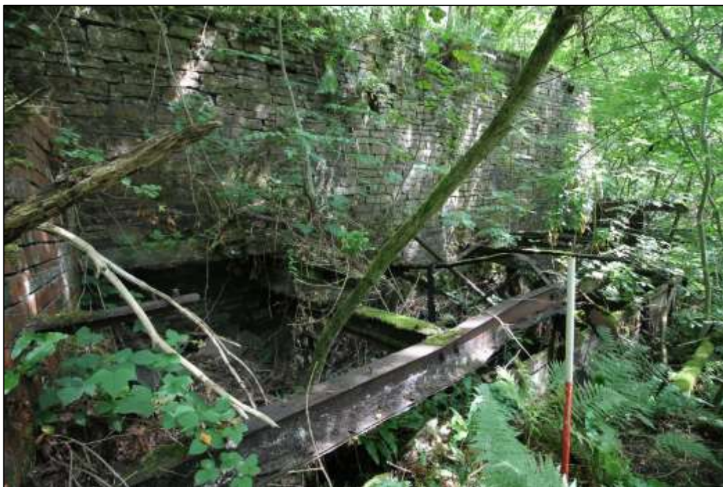
Plate 55: Steel frame above timber tanks, facing east
