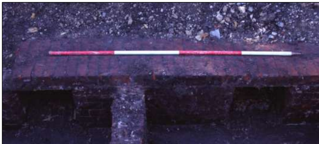
Plate 9: The openings on the southern elevation of the tank in Trench 5
