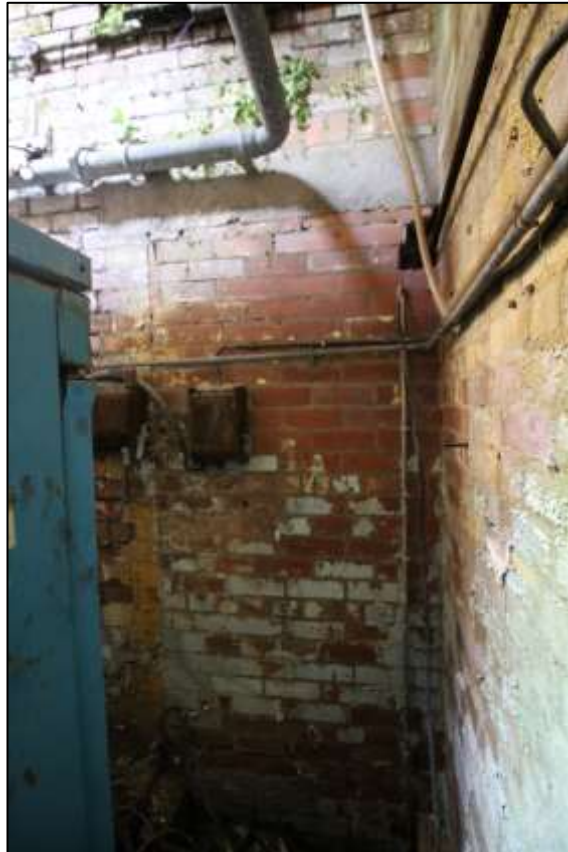
Plate 49: Blocked doorway on the western wall of the larger cell
