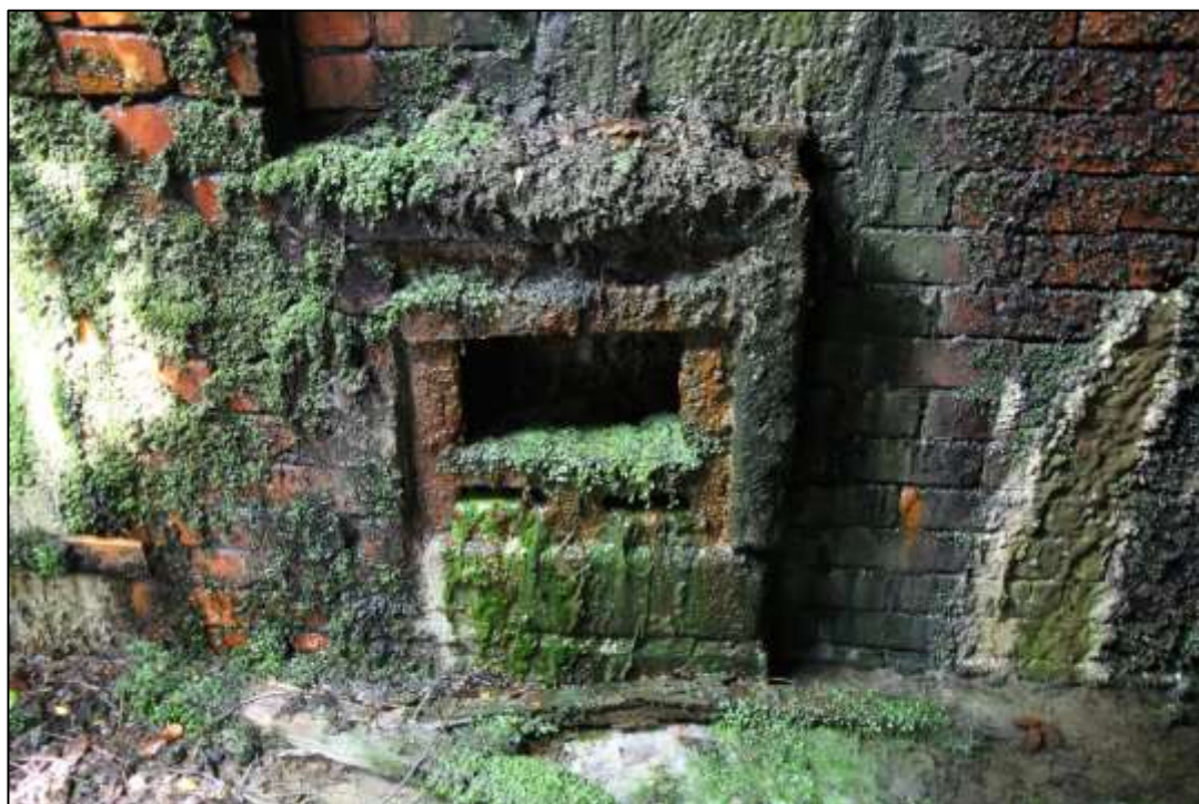
Plate 59: End bearing box on north-western wall of open-sided building
