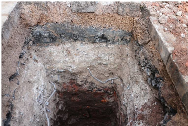
Plate 14: BH 20, looking north
