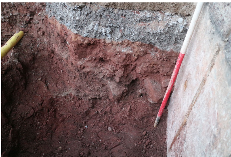
Plate 17: Extension trench to BH 101, looking north-east, showing sandstone rubble adjacent to the outer face of the basement retaining wall of the Forum shopping centre
