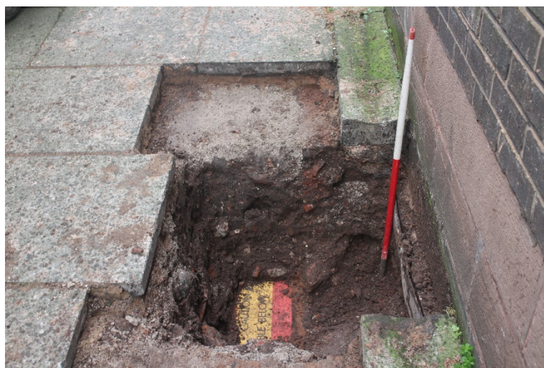
Plate 6: TP 6, looking east
