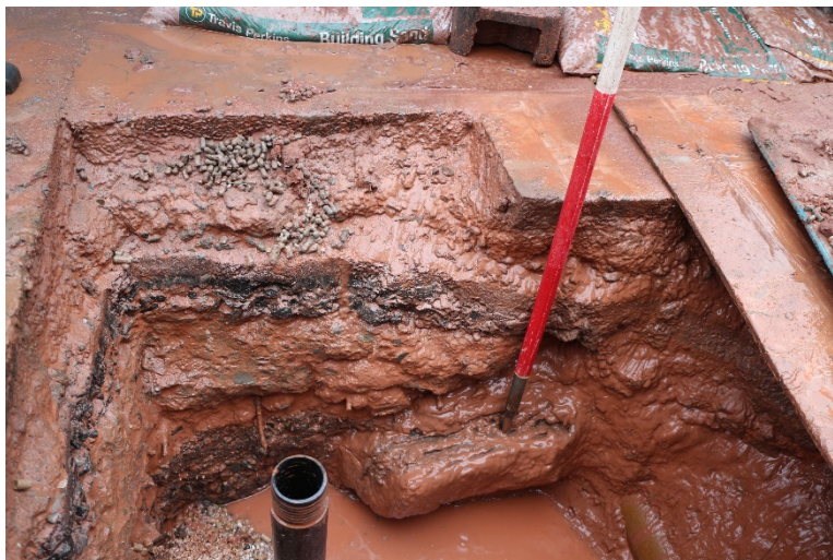
Plate 11: Start hole for BH 12, looking east, showing sandstone block in deposit 1205
