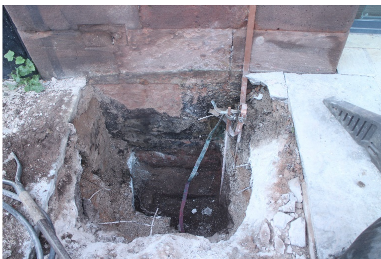
Plate 1: TP 1, looking west
