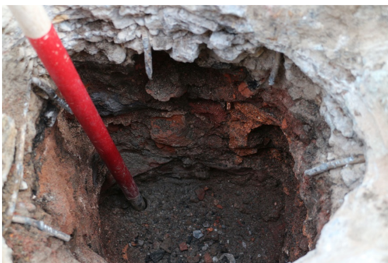
Plate 12: BH 13, looking east
