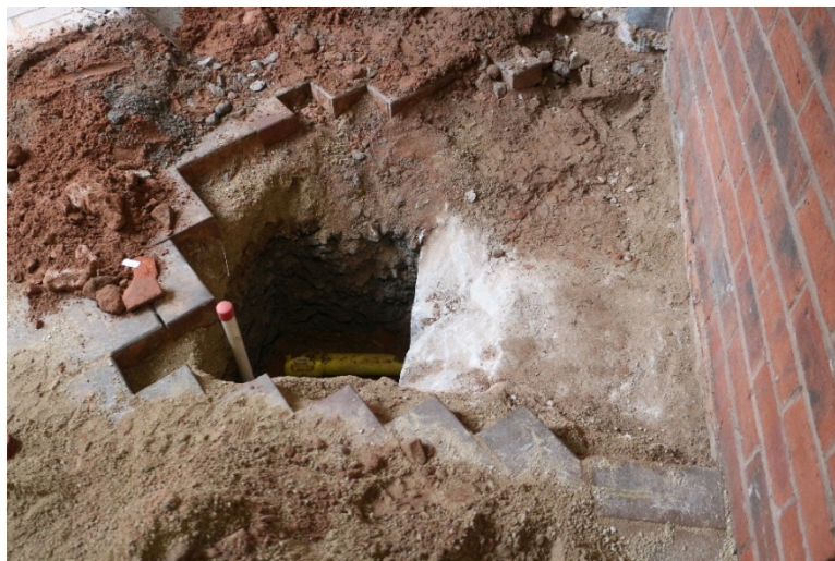
Plate 3: TP 3, looking south-west
