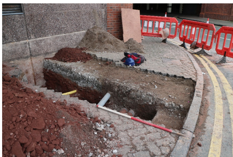
Plate 15: Extension trench for BH 101, looking south-west, showing utilities
