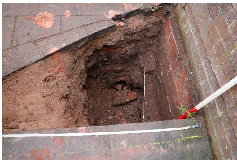
Plate 2: TP 2, looking east
