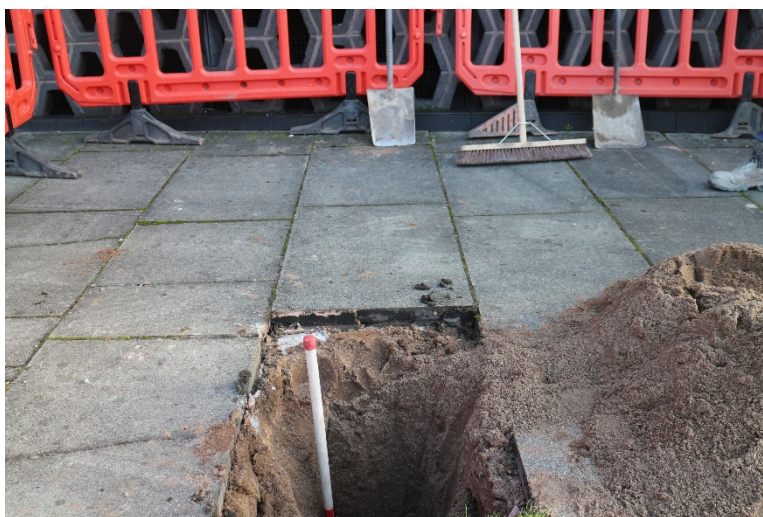
Plate 13: BH 16, looking east
