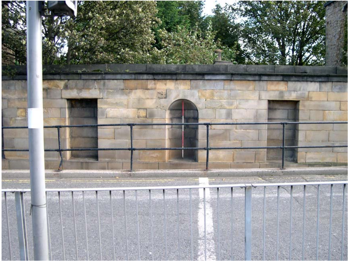
Plate 8: Detail of the front (north) elevation of the east link wall
