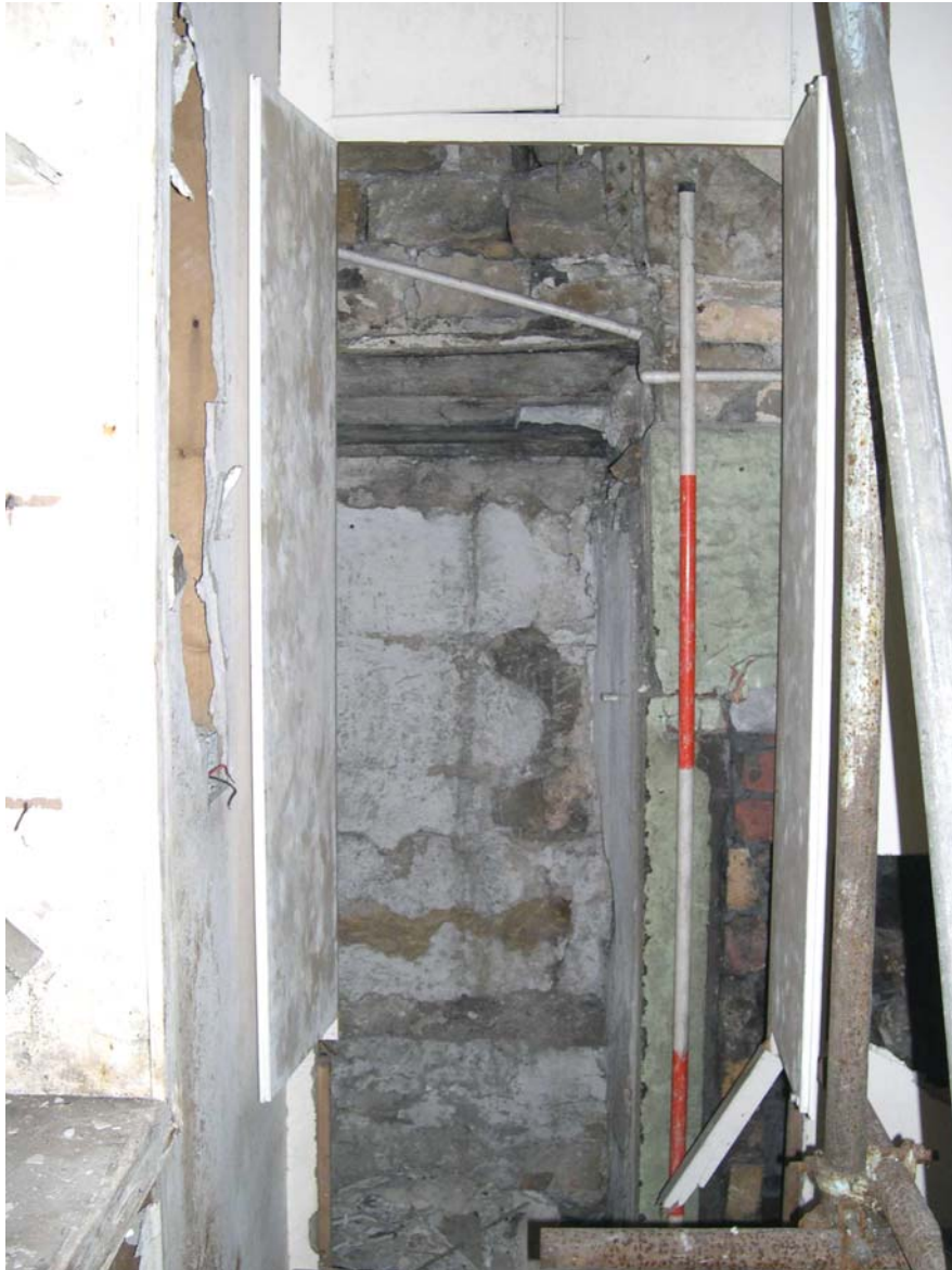
Plate 23: Part of the fireplace and built-in cupboard, Room 12, west Bridge House
