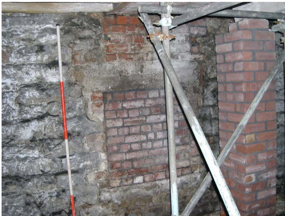
Plate 12: Blocked apertures and inserted brick pillar in Room 2, east Bridge House
