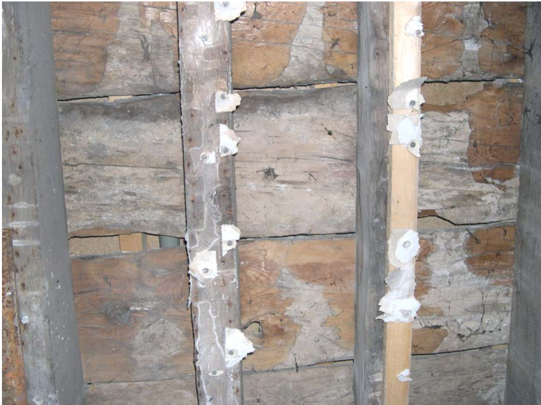
Plate 22: An example of early hand-finished floorboards exposed in the ceiling of Room 5, west Bridge House
