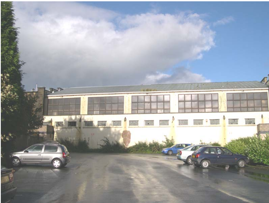
Plate 27: North end of west external elevation of baths
