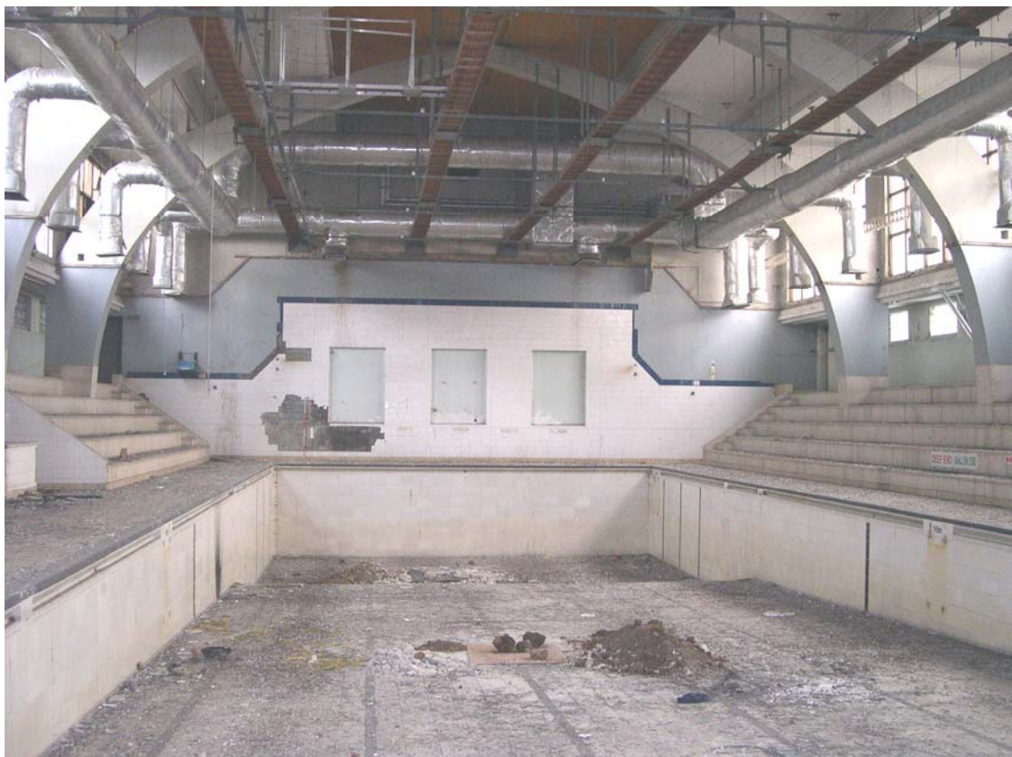
Plate 33: General view of main pool (Room 19) looking south, baths
