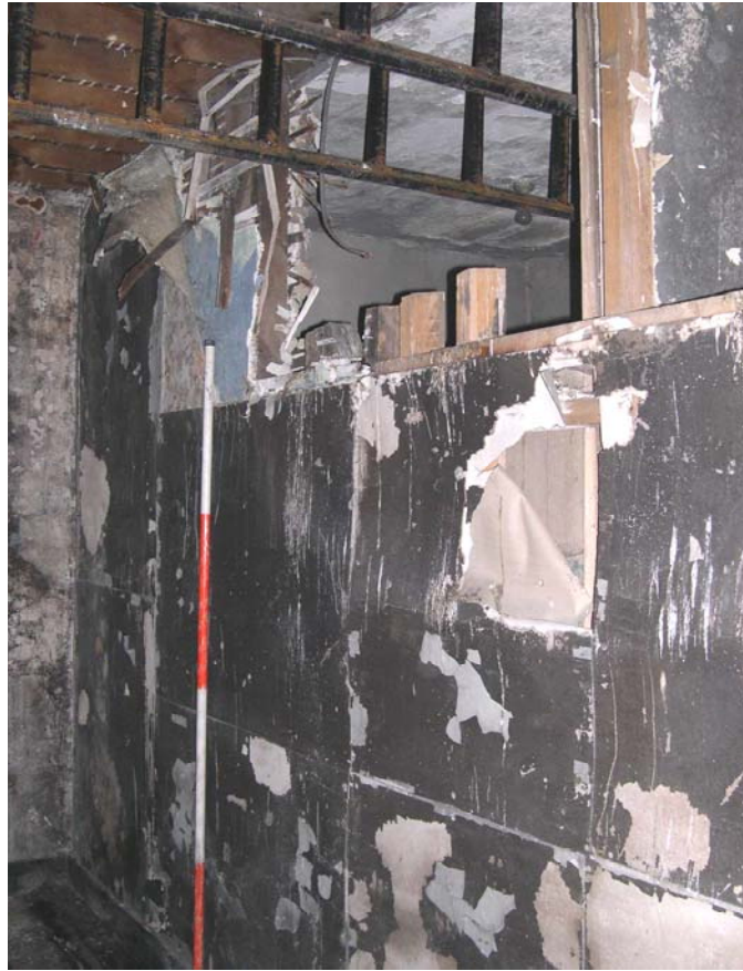
Plate 24: Junction of modern and early partitions between Rooms 14 and 18 , west Bridge House
