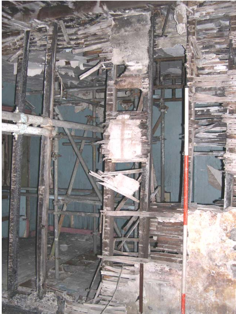
Plate 17: Exposed partition wall between Rooms 13 and 14 , east Bridge House
