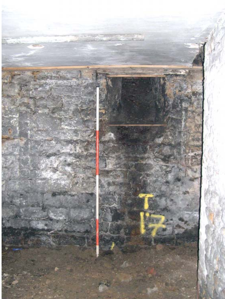
Plate 11: Coal chute in Room 1, east Bridge House
