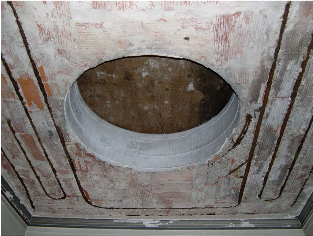
Plate 36: Example of the reinforced ceiling structure and skylight, Room 5, baths
