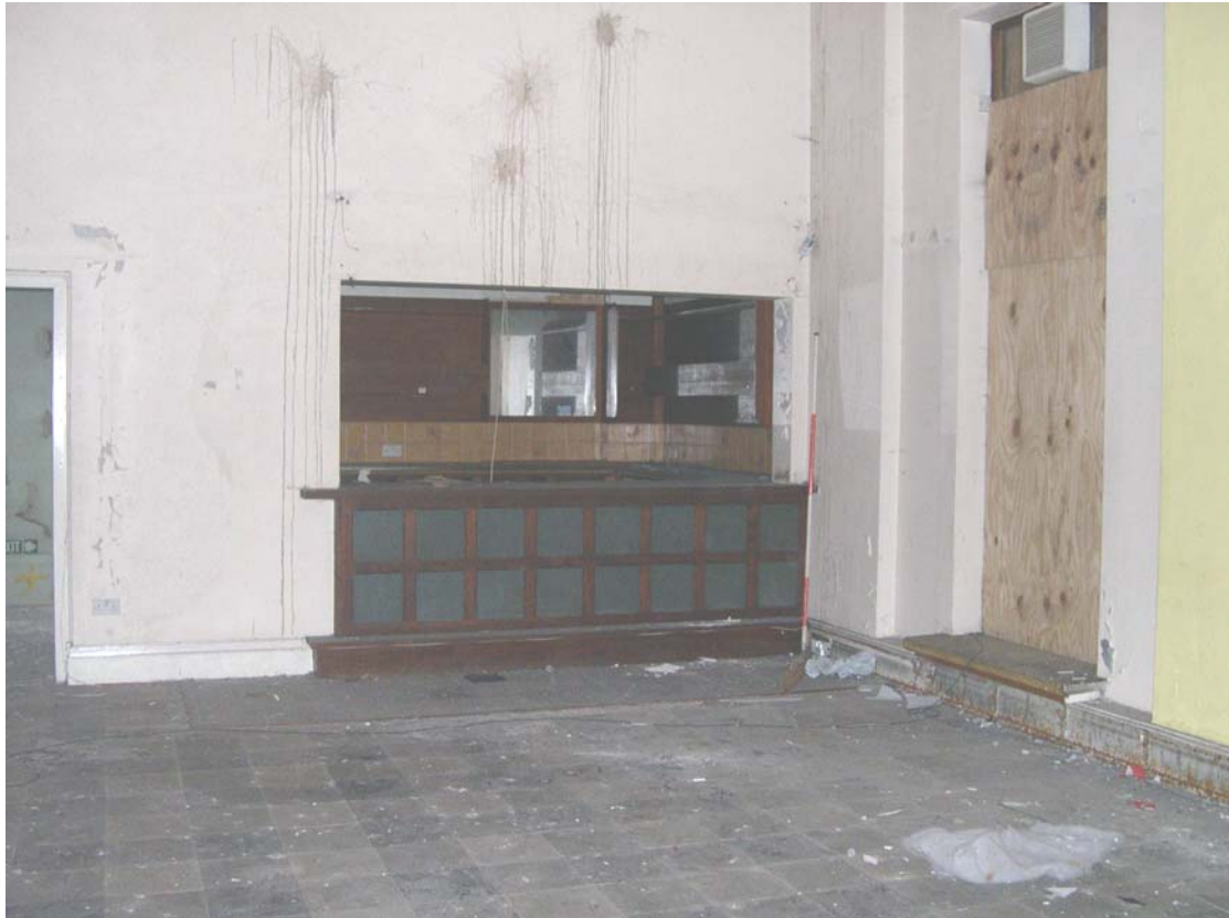
Plate 38: General view of second floor bar area (Room 30), looking west, baths
