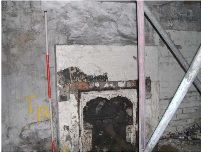
Plate 13: Fireplace with large stone surround and inserted iron surround, Room 5, east Bridge House
