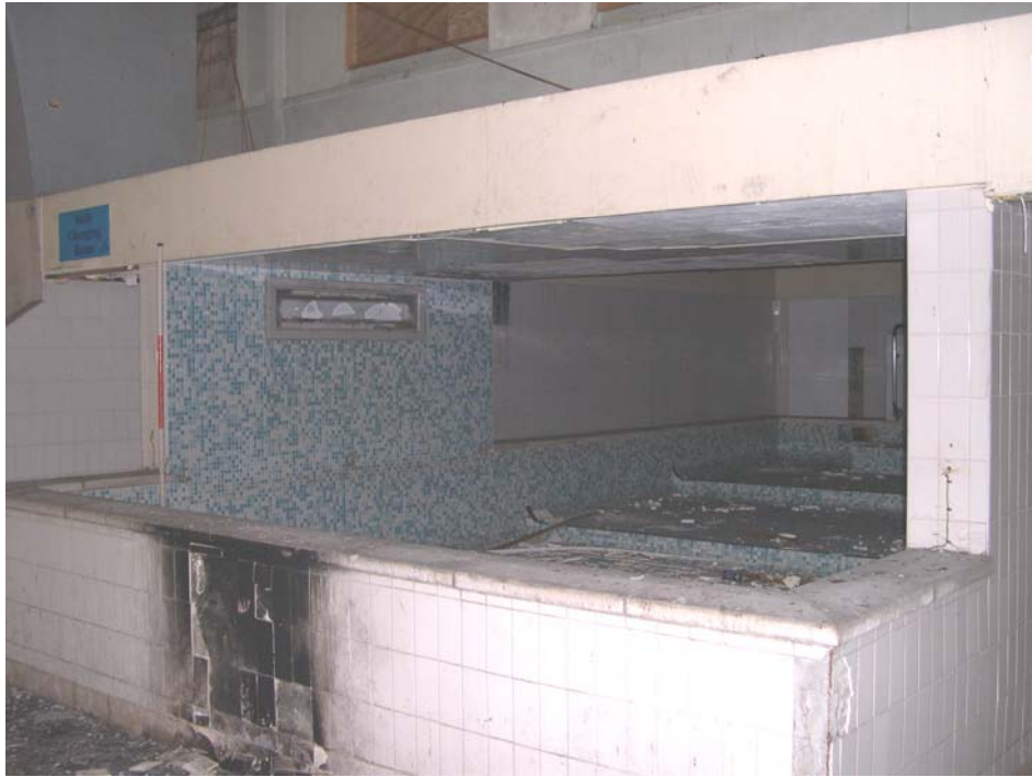
Plate 34: Learner/disabled pool on east side of main pool (Room 19 ), baths
