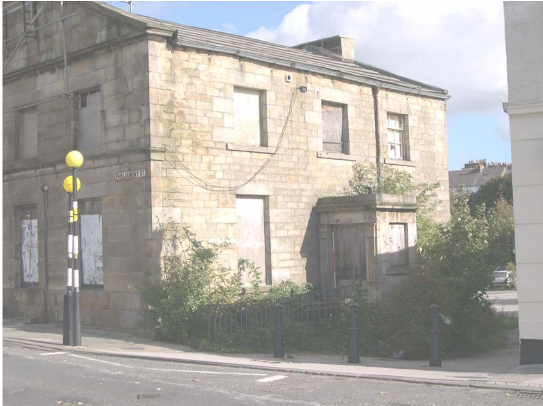
Plate 6: front (west) external elevation of west Bridge House showing blind windows
