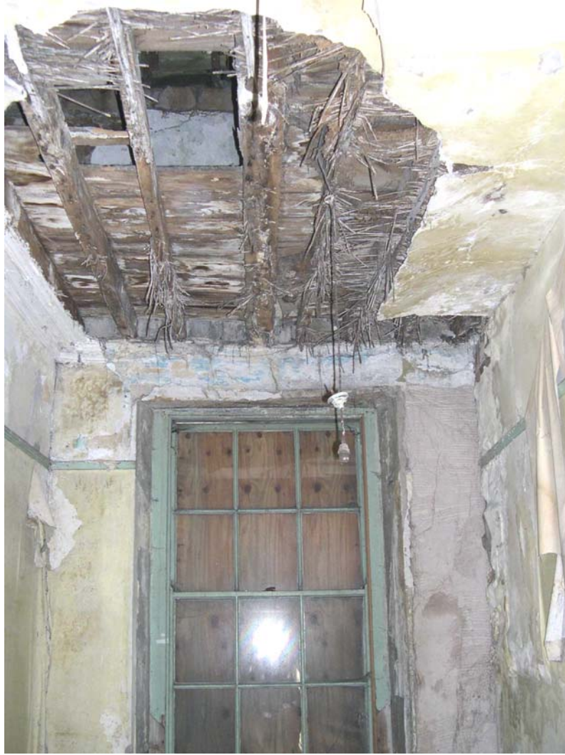
Plate 19: Exposed reed-plaster ceiling and window in Room 11 , central Bridge House
