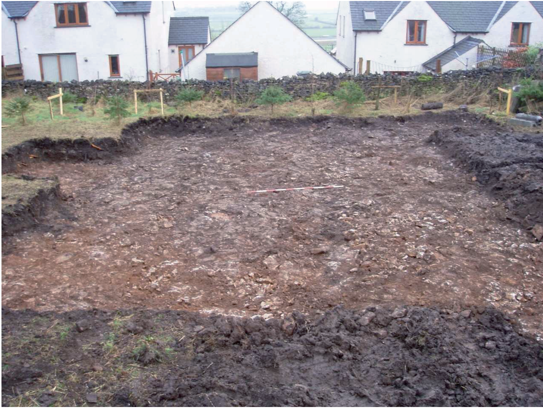
Plate 1: evaluation area after stripping, looking south
