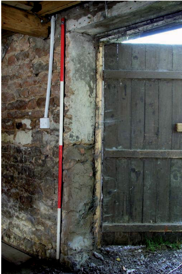
Plate 6: Doorway into Room 3 showing modified lower jambs
