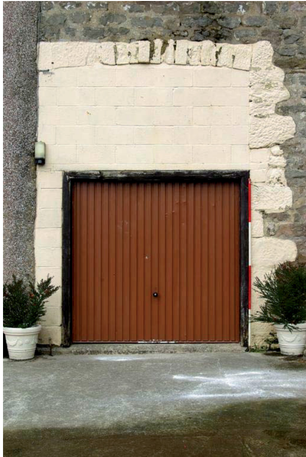
Plate 5: The main barn door on the south elevation
