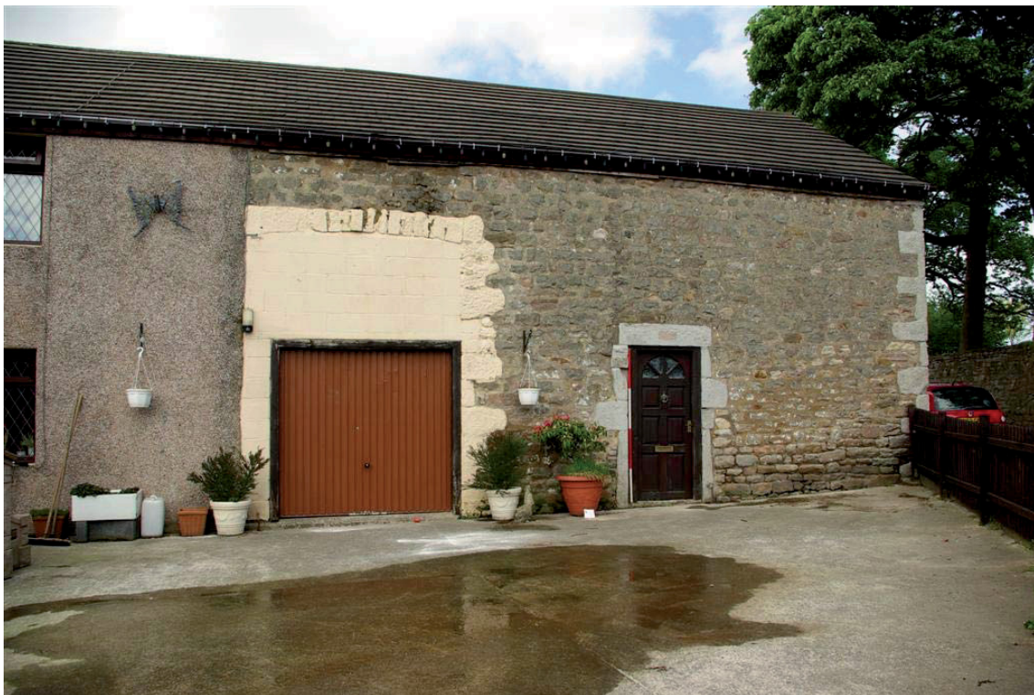
Plate 2: The south elevation of the barn
