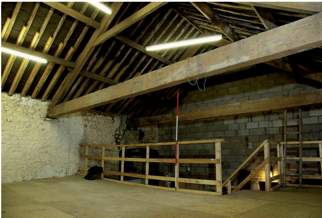
Plate 11: View of Room 4 facing west towards Room 1
