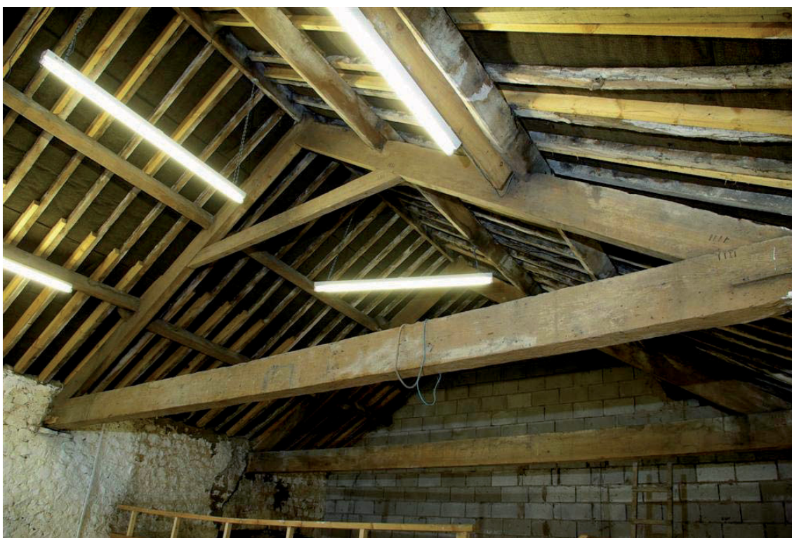
Plate 12: The roof as viewed from Room 4
