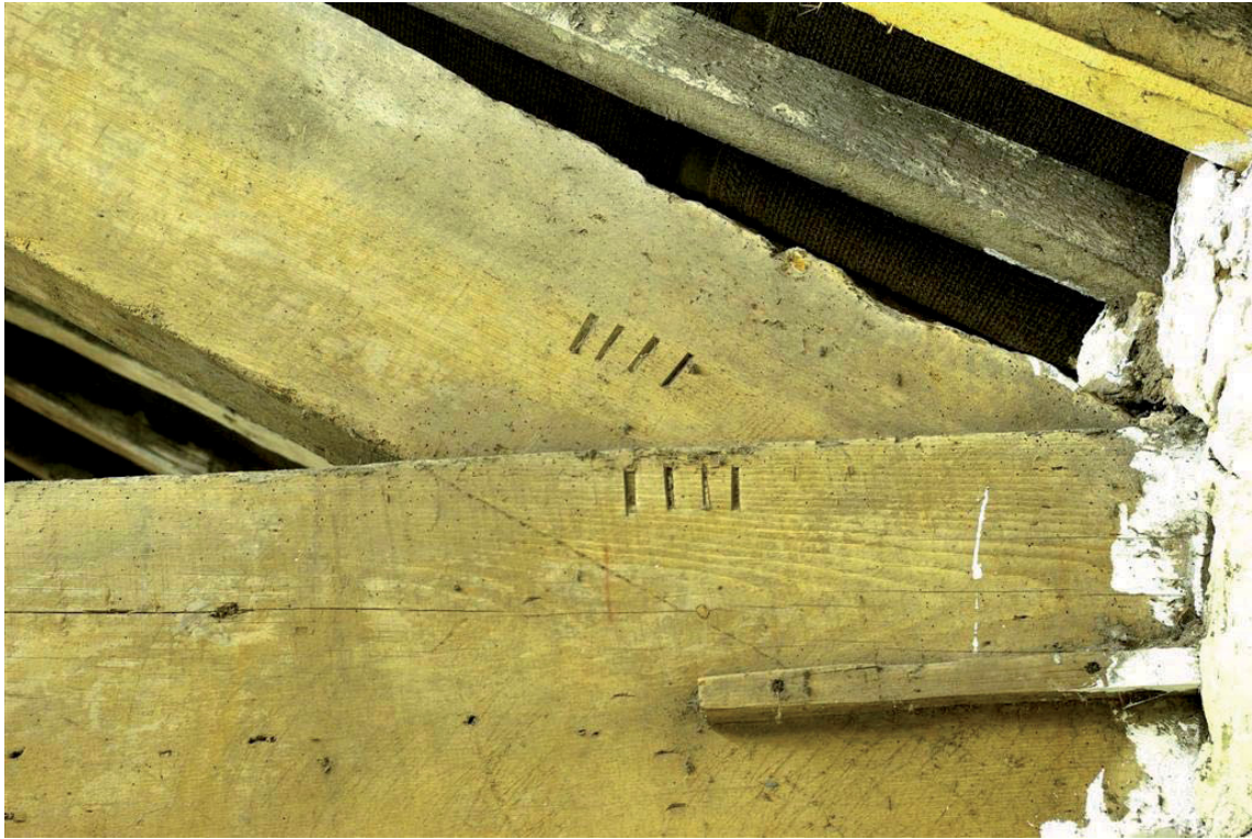
Plate 13: Example of the carpenter's marks
