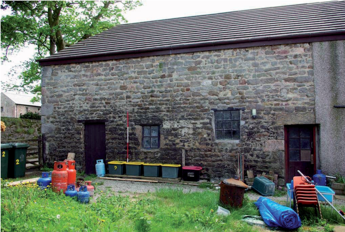
Plate 3: The north elevation of the barn
