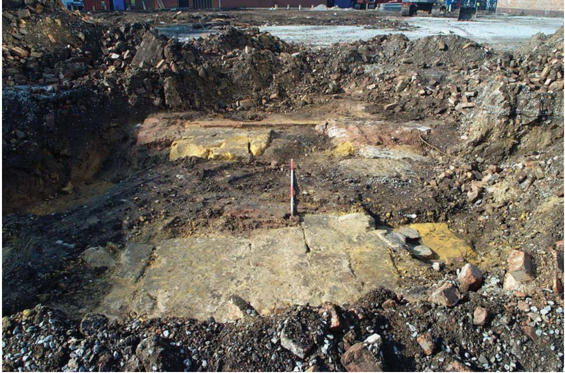
Plate 3: Northern section of wall foundations 701 (foreground) and 702 , viewed from the south-west
