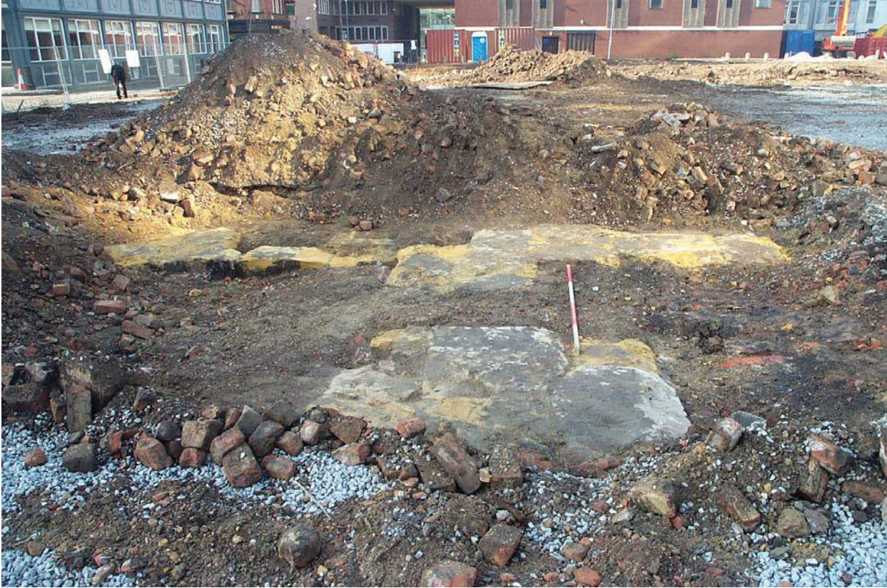
Plate 5: Wall foundations 705 (foreground) and 706 viewed from the north-east
