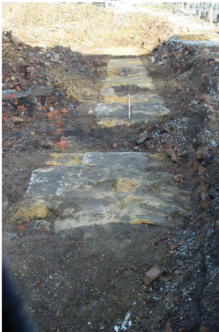
Plate 4: Wall foundations of 703 , 704 and 705 (foreground) viewed from the south-east
