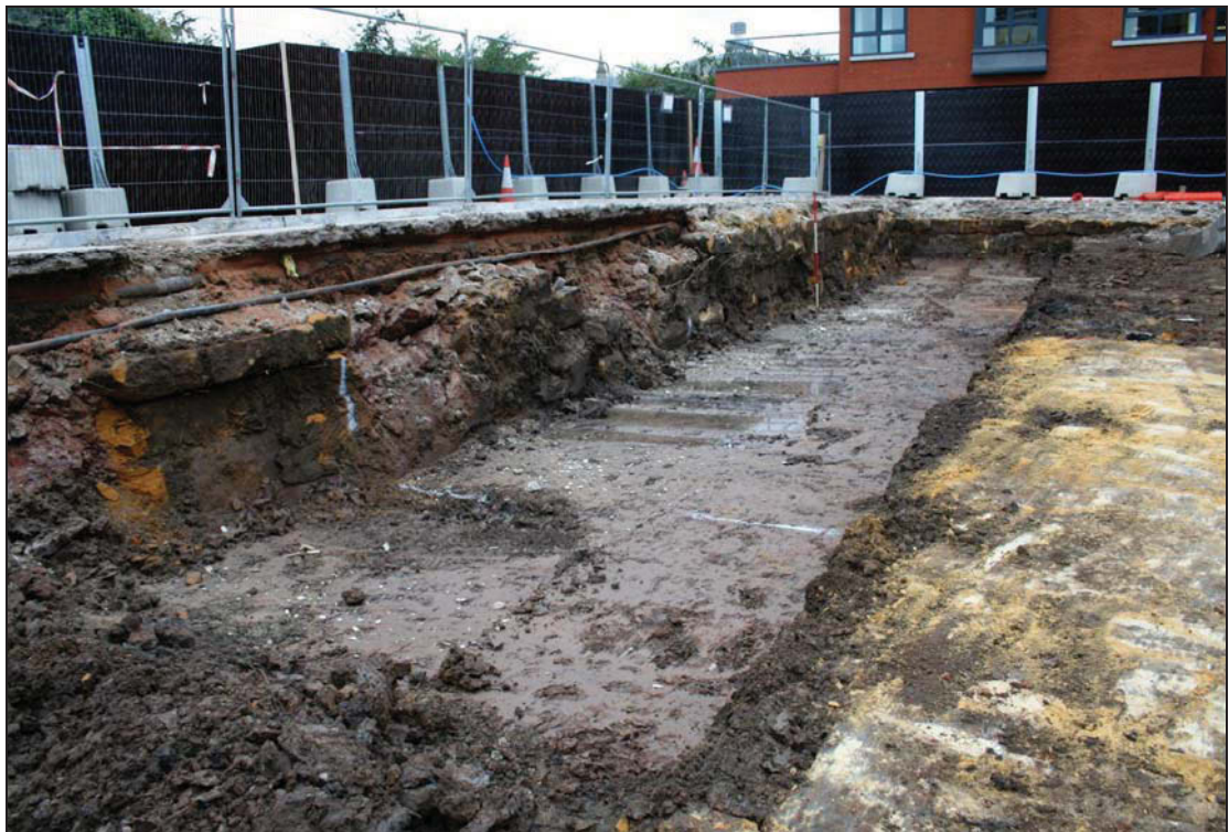
Plate 19: South-east end of graveyard perimeter wall 324
