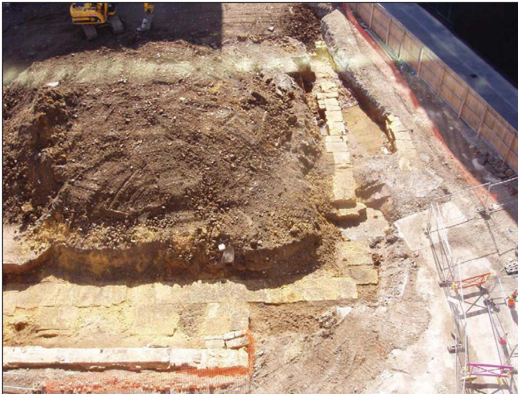
Plate 15: Foundations for the north-east corner of St Paul's Church
