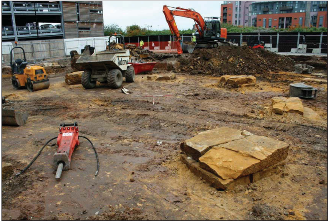
Plate 16: Supporting plinths 307 for the dome of St Paul's Church
