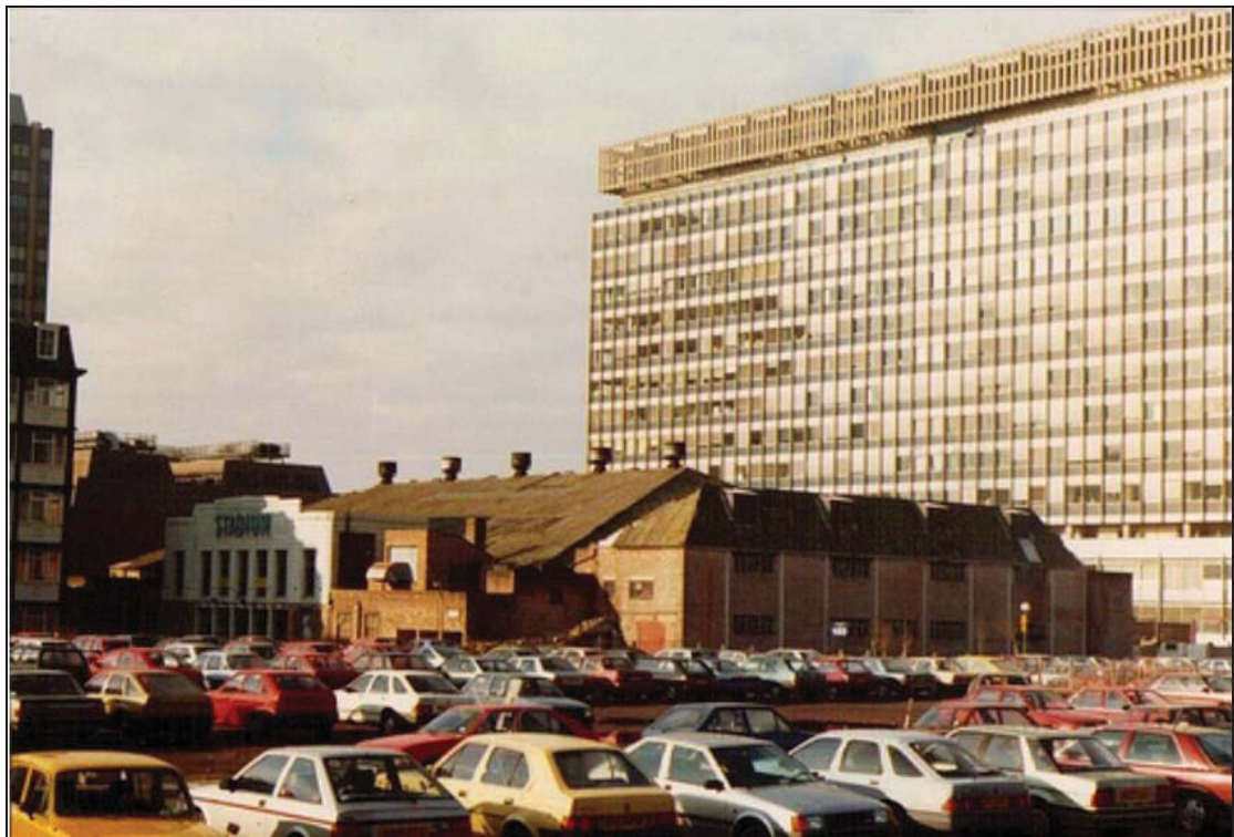
Plate 11: Liverpool Stadium looking west, February 1987 (copyright PG Mayer)
