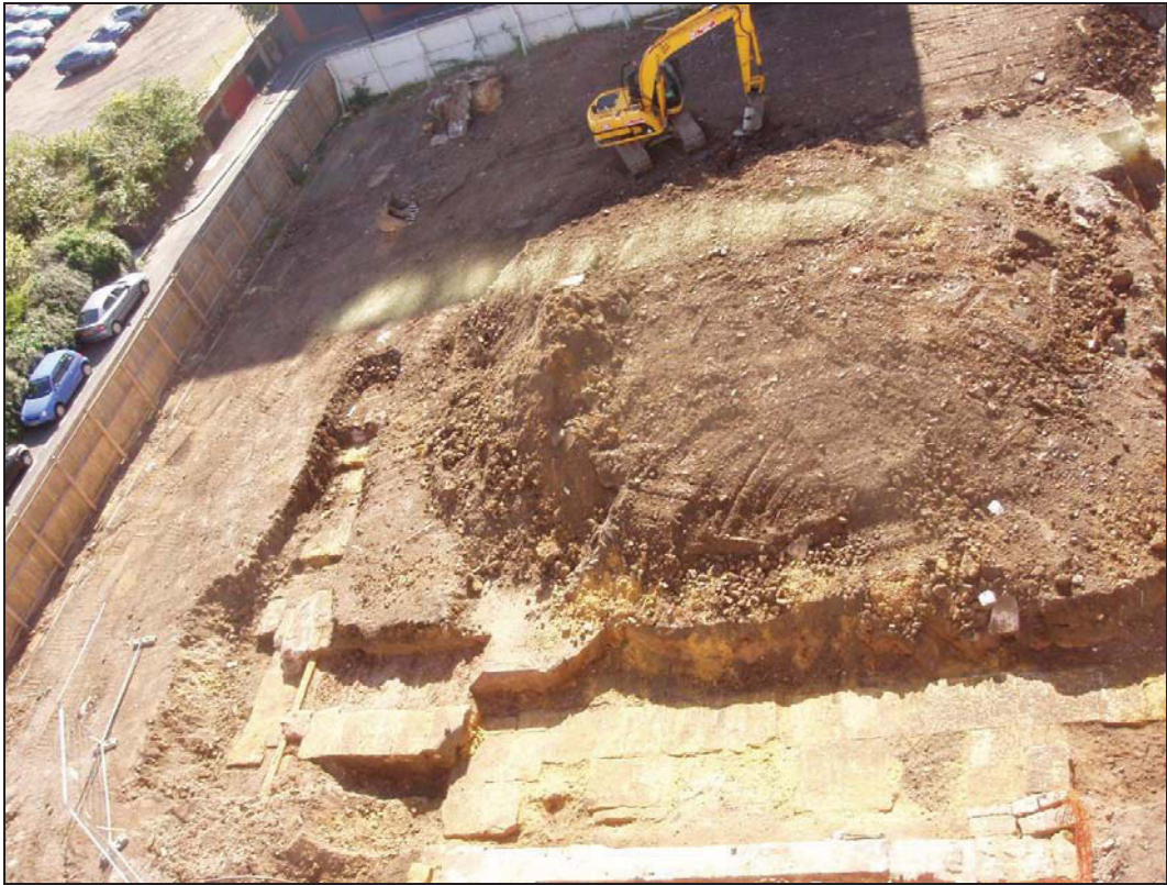
Plate 12: Foundations for the north-east corner of St Paul's Church
