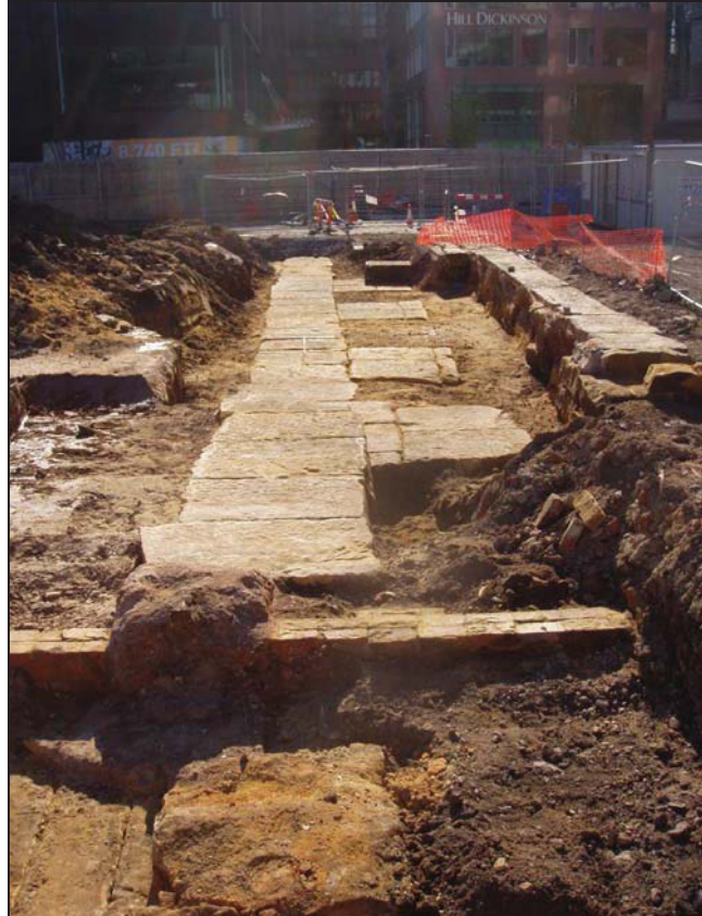
Plate 13: Foundations for the north end of St Paul's Church
