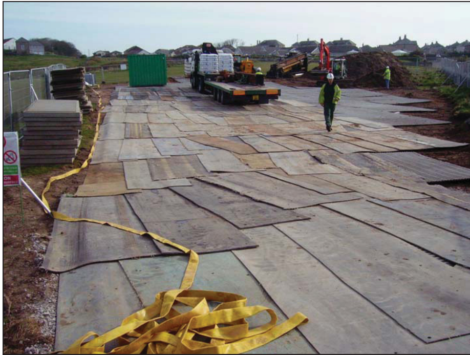
Plate 3: Area of topsoil strip adjacent to Old Smithy Lane, looking north-west
