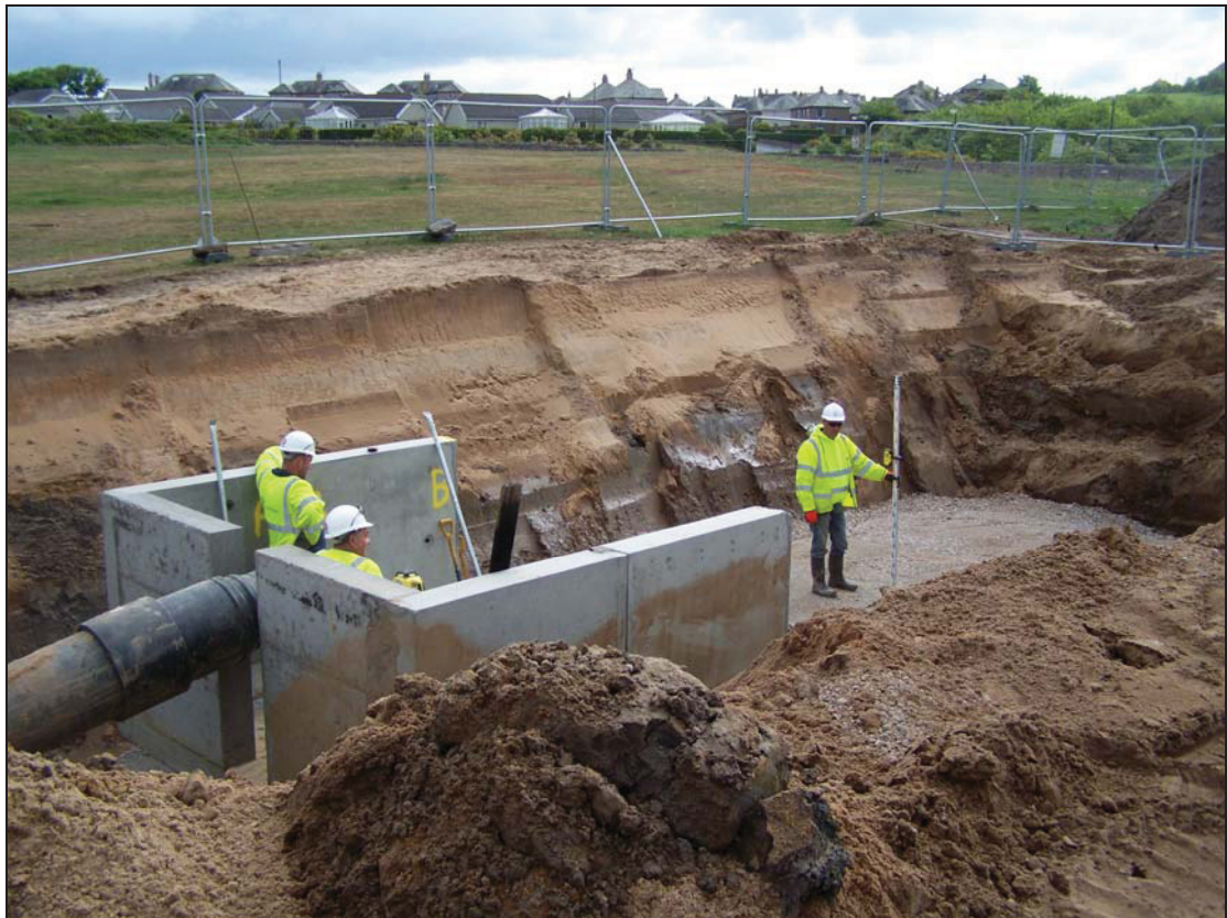
Plate 6: Extension to pit for drilling rig, looking north-west
