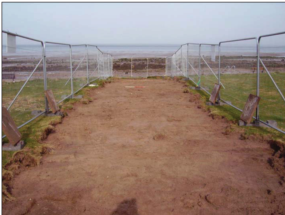
Plate 4: Area of topsoil strip perpendicular to sea wall, looking north-east
