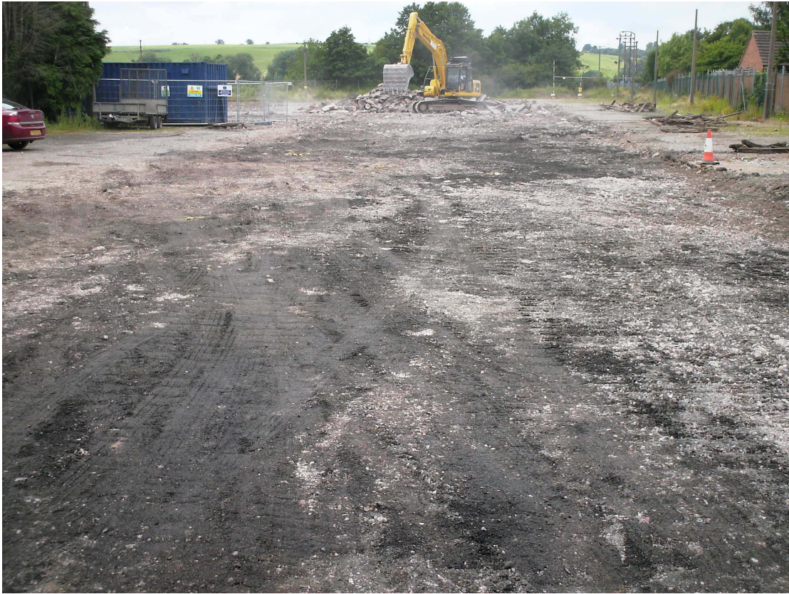
Plate 1: Concrete surface removed from western plot
