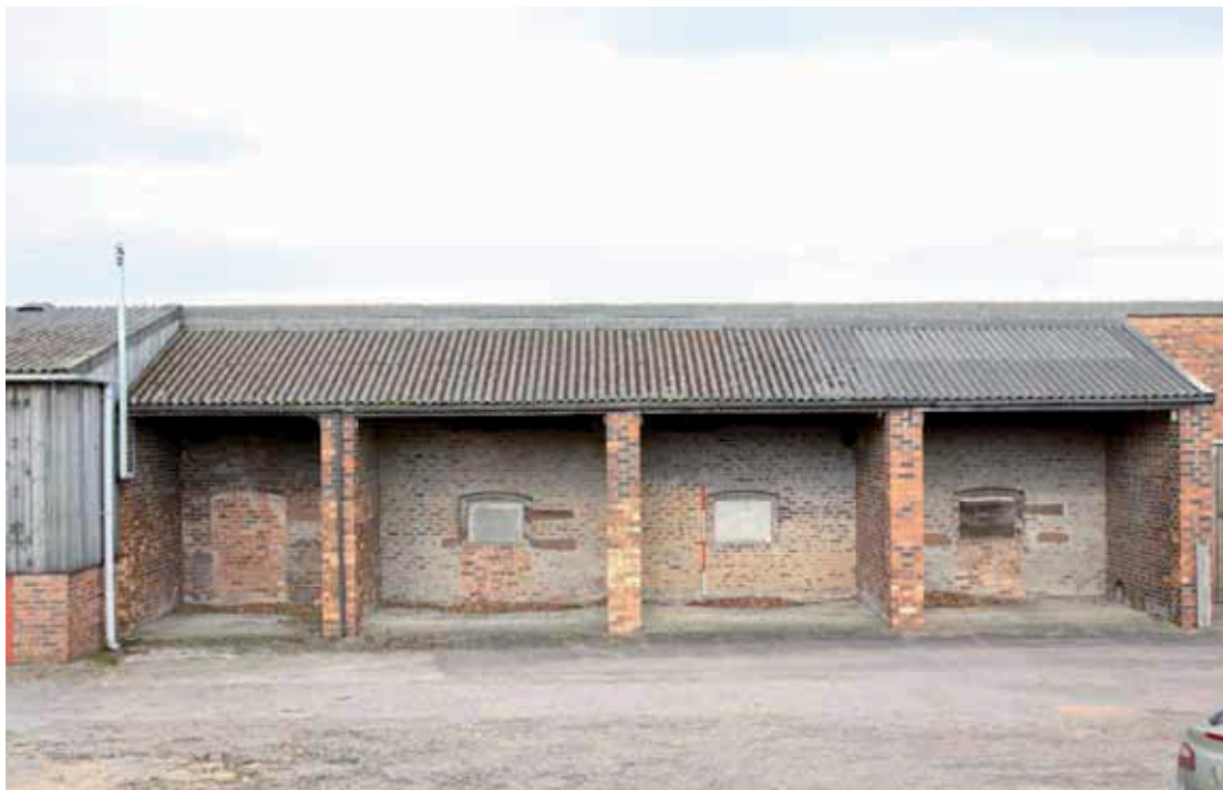
Plate 30: Building 2 incorporated into Building 5, showing a series of blocked doorways
