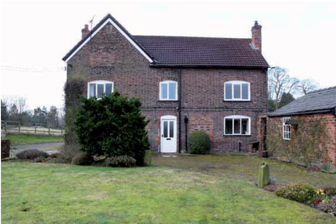
Plate 2: Front elevation of the farmhouse, one of the blocked doorways is evident, as is the blocked window at attic floor level, and the datestone
