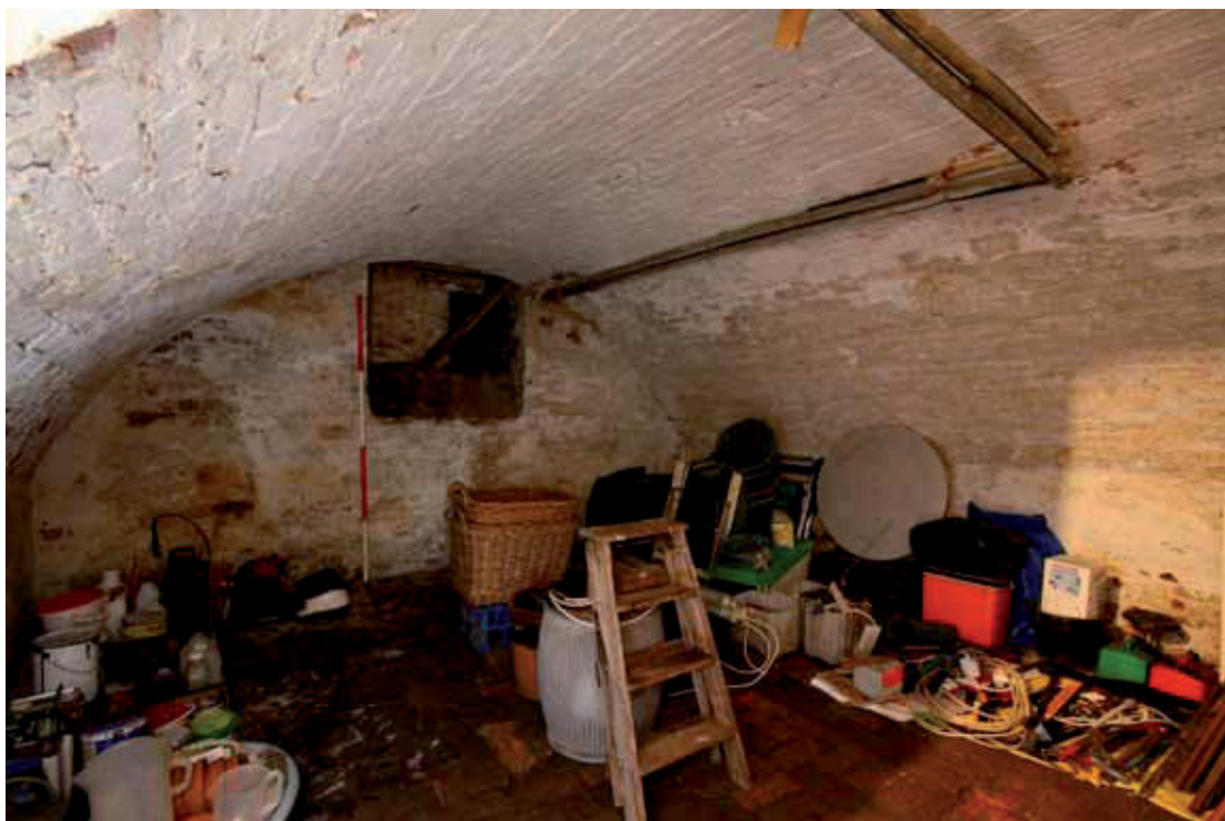
Plate 17: Cellar with coal chute in front wall
