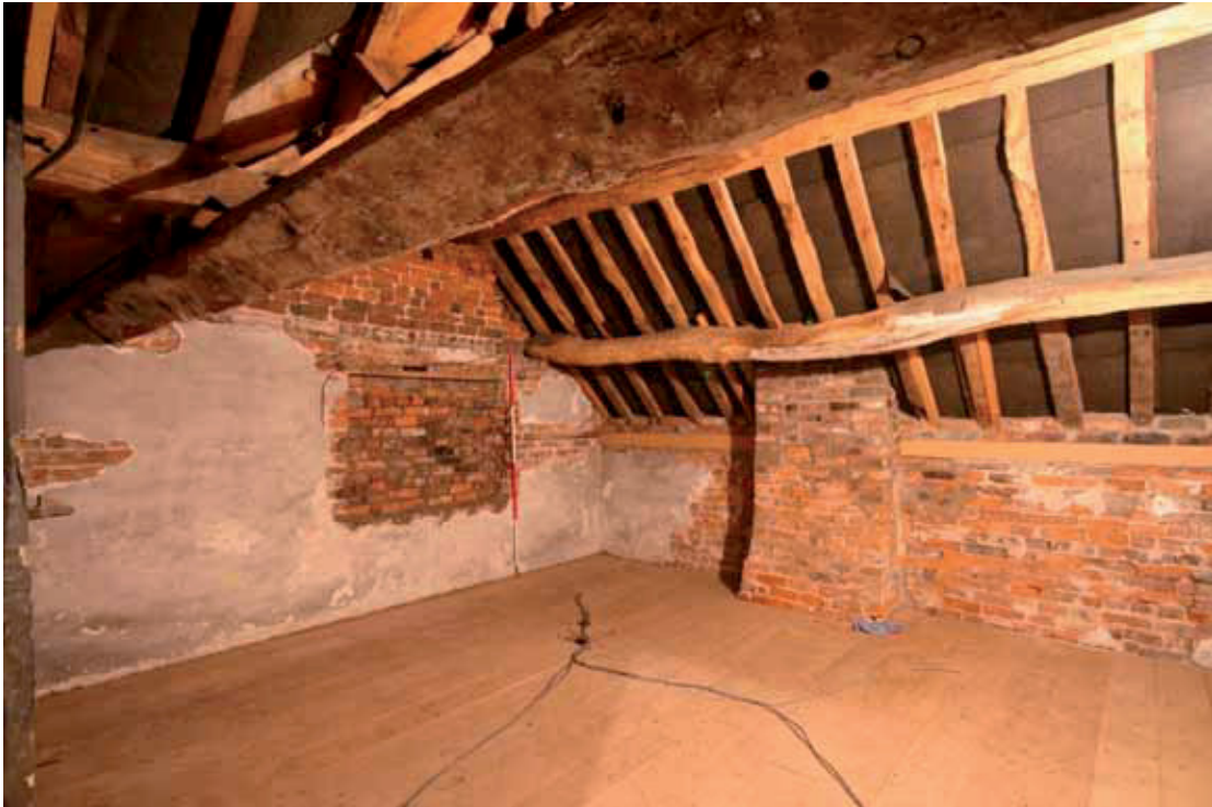
Plate 13: Blocked window within the attic, and partially re-built flue
