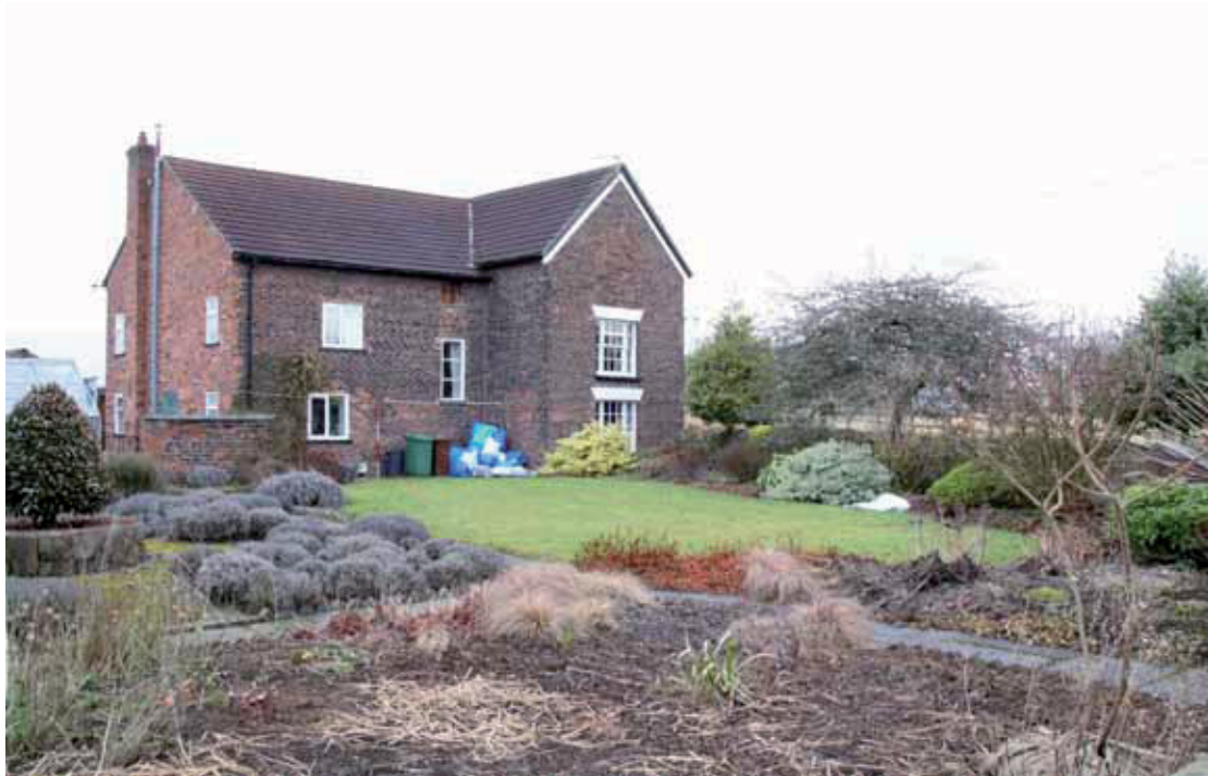
Plate 3: Rear view of farmhouse showing projecting wing with sash windows, new gable to the north-west
