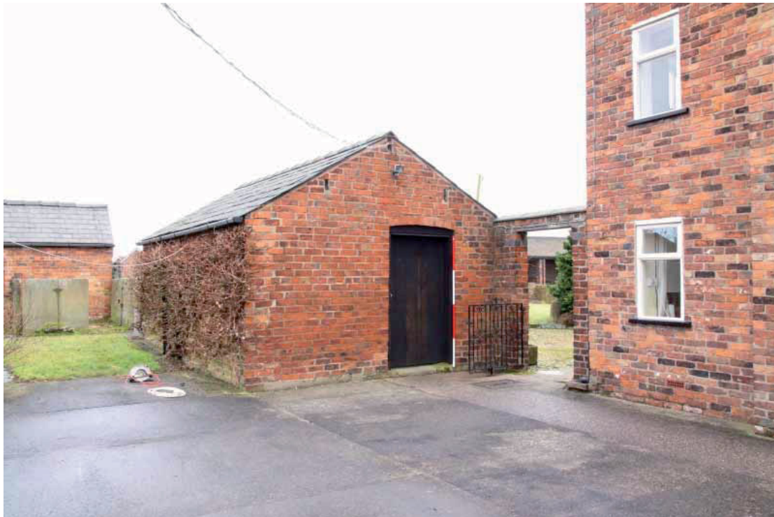
Plate 20: Garage with roof purlins evident in elevation
