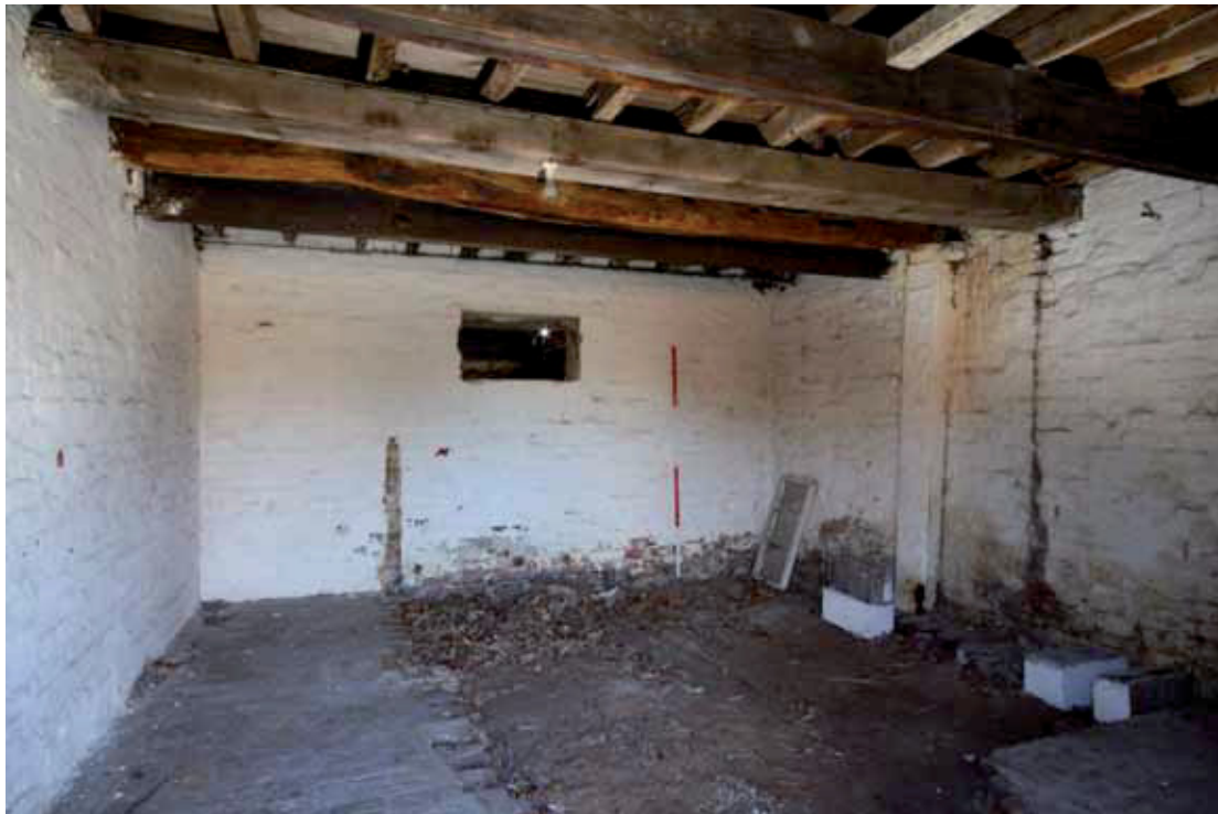
Plate 26: Cart shed within the first bay of the barn (Building 1)
