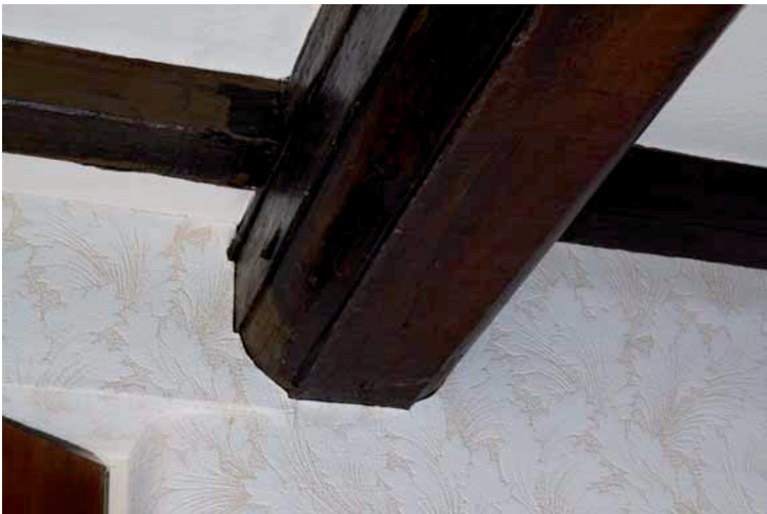
Plate 6: Detail of an ovolo-chamfered beam
