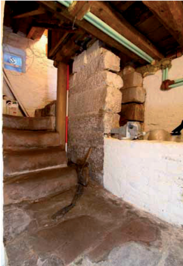
Plate 16: Detail of staircase in the cellar
