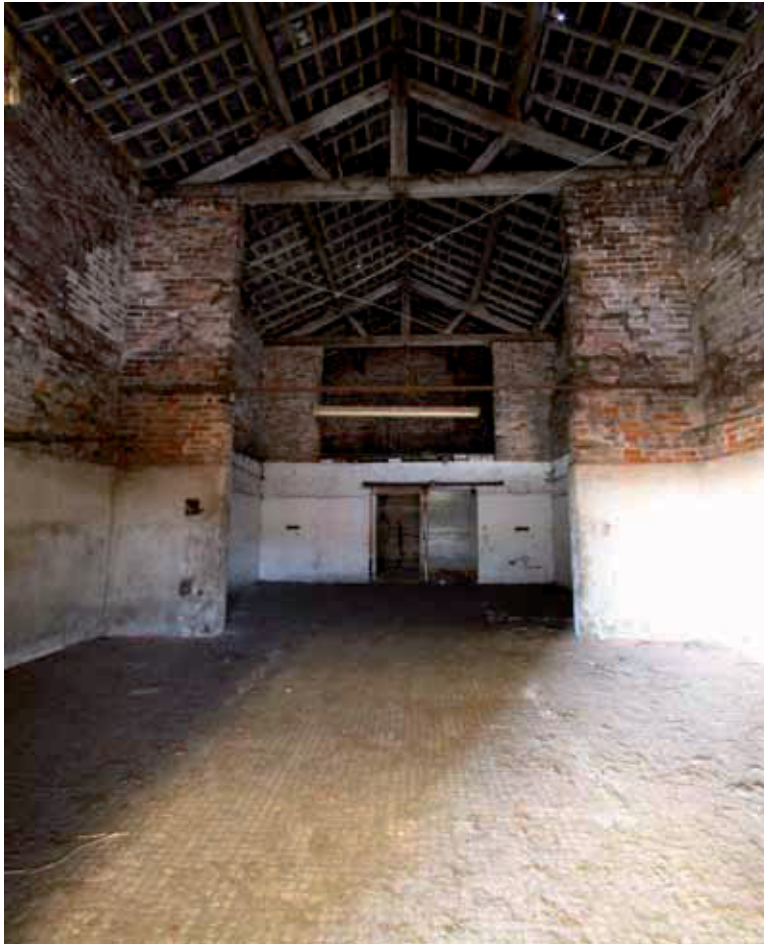
Plate 28: Open interior of the barn (Building 1) showing king-post trusses supported on brick buttresses
