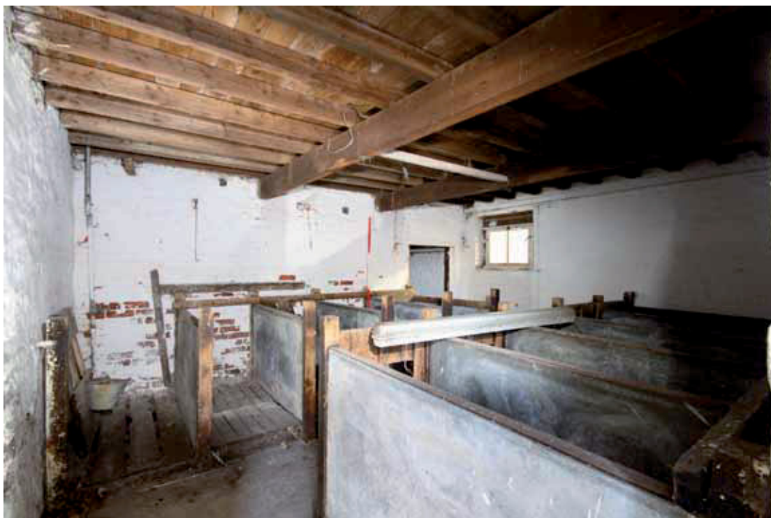
Plate 27: Calf shed with modern beams over
