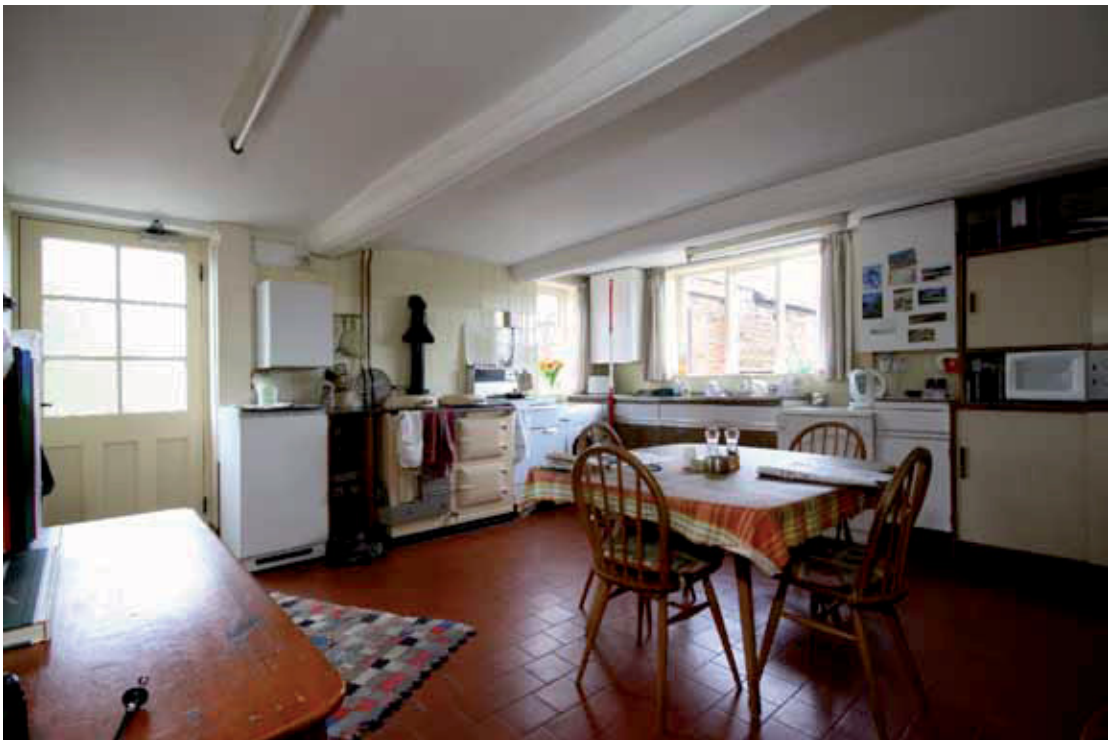
Plate 8: Kitchen with range and painted ovolo-chamfered beams
