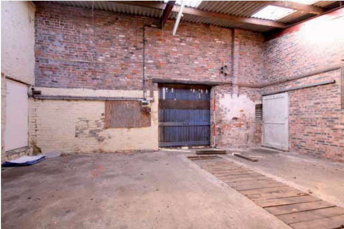
Plate 34: Interior of Building 4 with inspection pit in floor
