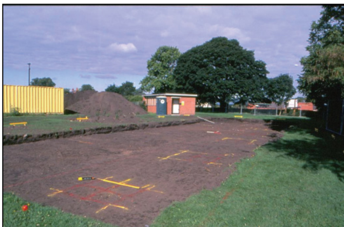
Plate 4: Completed strip for the new park management building, looking west.
