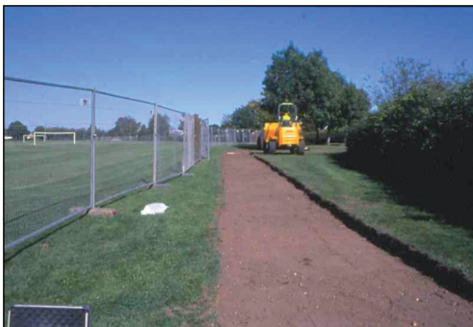
Plate 8: Working shot during path stripping in Area B, looking north-east.
