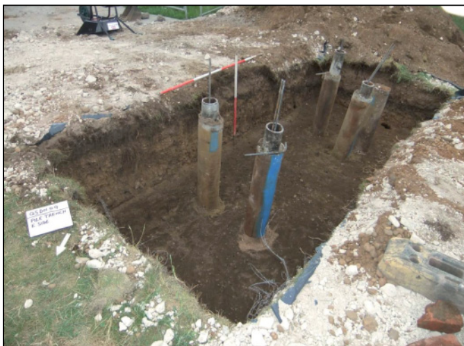
Plate 12: The completed eastern pile cap trench, looking south.
