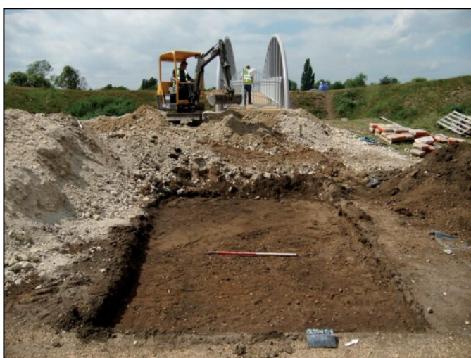
Plate 16: The topsoil strip for the eastern bridge approach, looking north-west.
