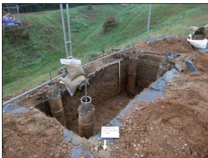
Plate 14: The completed western pile cap trench, looking south.
