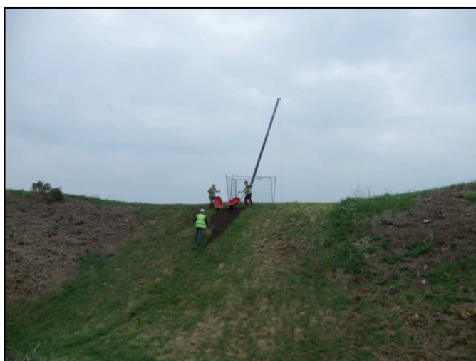
Plate 17: The scar repair process: excavated material from the pile cap trenches being transferred by wheelbarrow.
