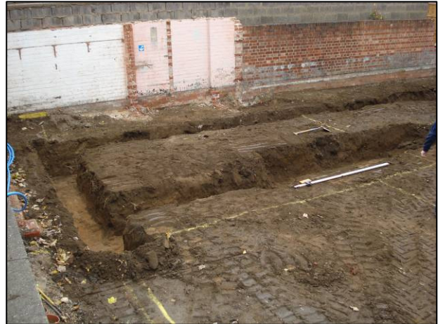
Plate 2 Excavated footings, Looking north.
