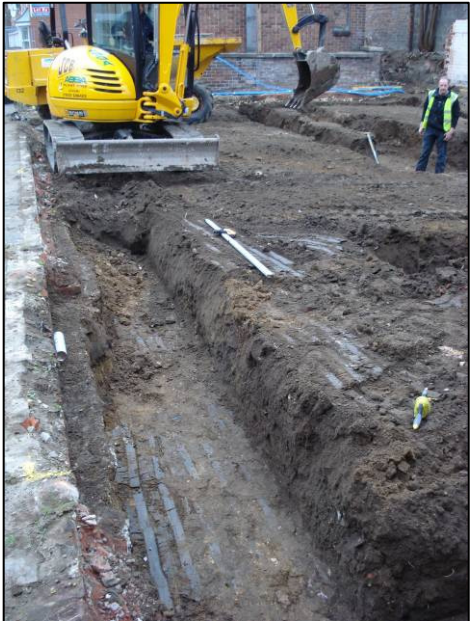
Plate 4. Excavation of footing within east-west Run of drain [008].
