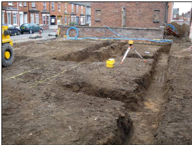
Plate 3. Excavated footings looking south-west. Soakaway [006] in foreground truncated by machine.
