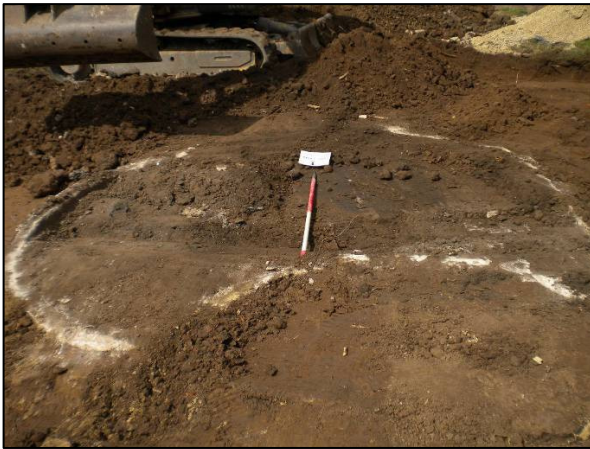
Plate 8: Concrete feature [305], probably an ornamental pond, exposed during machine stripping of Area 3; looking north.
