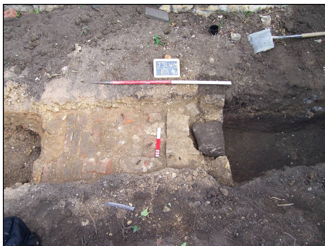
Plate 7: Limestone stable wall 110, with brick floor fragment 111, exposed in the service trench, looking north.
