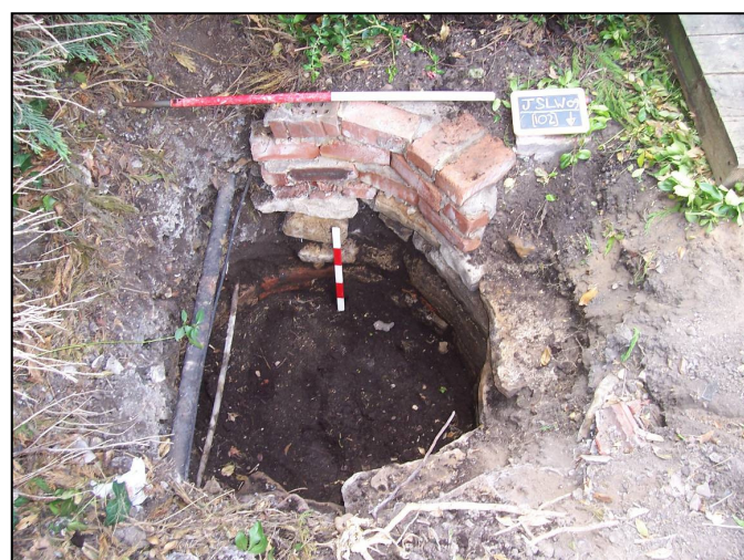
Plate 6: Well 103, showing the modern brick well head above the original limestone and brick construction.
