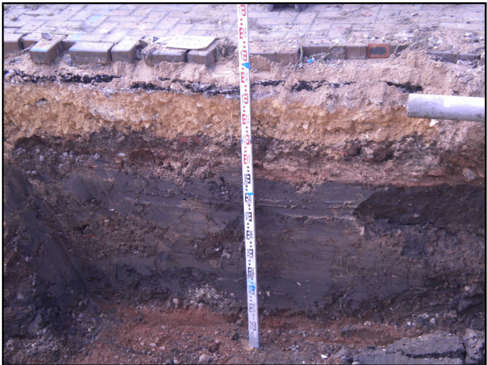
Plate.7 shot showing depth of made ground (113) and levelling deposits after removal of Victorian wall footings (114) at base of trench at southern end of site.
