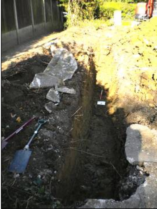
Pl. 1 Western foundation trench of the new extension (looking north).
