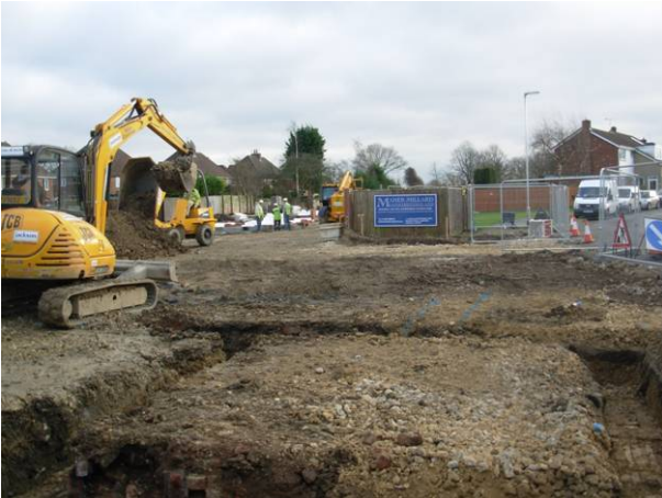
Plate 3 General site shot showing the excavation of footings in Plot 1
