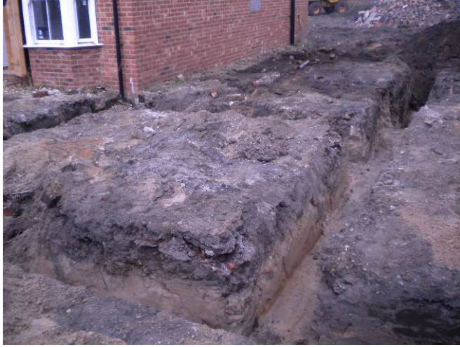
5. Excavated footings looking north-west.
