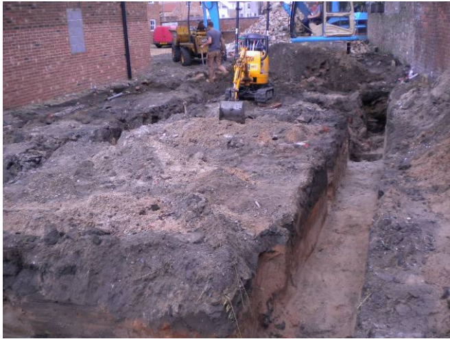
6. Excavated footings looking north-east.
