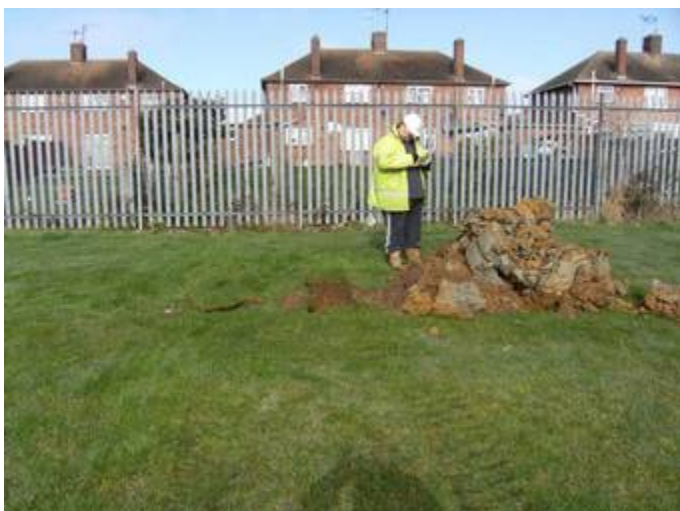
3. Geotechnical monitoring in progress, looking NW
