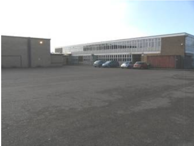
1. General view of the site, looking S
