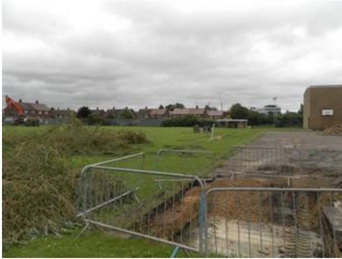
10. The site during CPR test-pit monitoring, looking N
