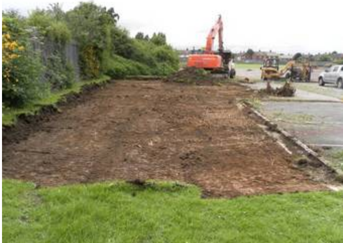
16. Topsoil stripping along the western edge of the site, looking NE
