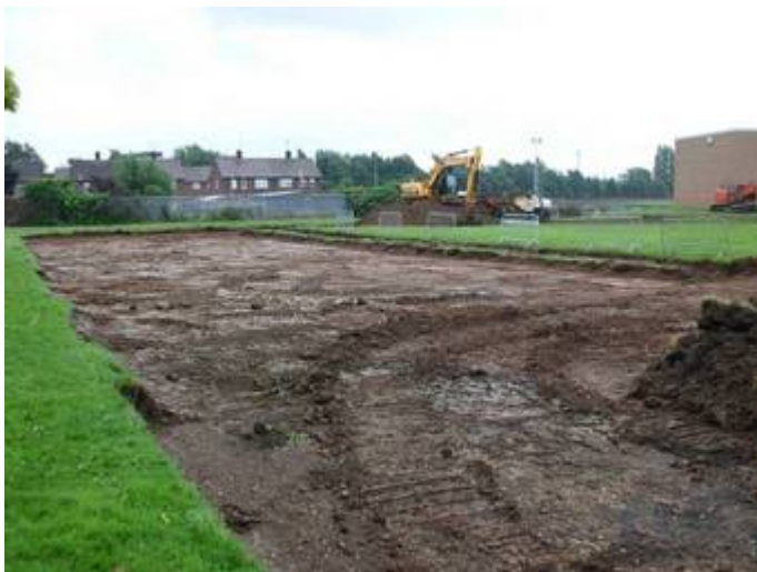
15. Topsoil stripping for the new SEN building, looking NE
