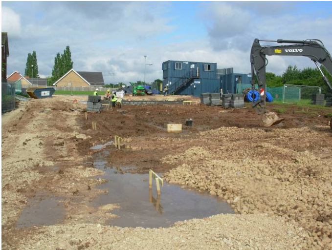
10. General view of plots 7-9, showing the poor ground conditions on the site
