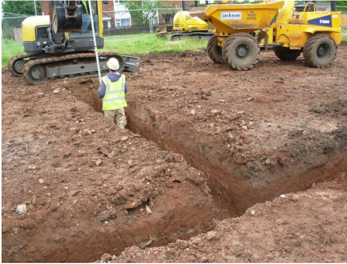
3. Working shot of house plots 3 and 4
