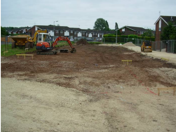
1. General view of the site during ground reduction
