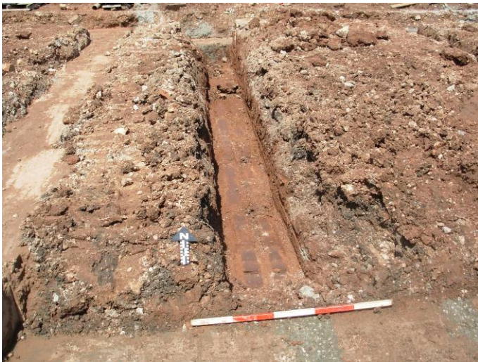
8. Sample section of Plot 5 footings, looking north
