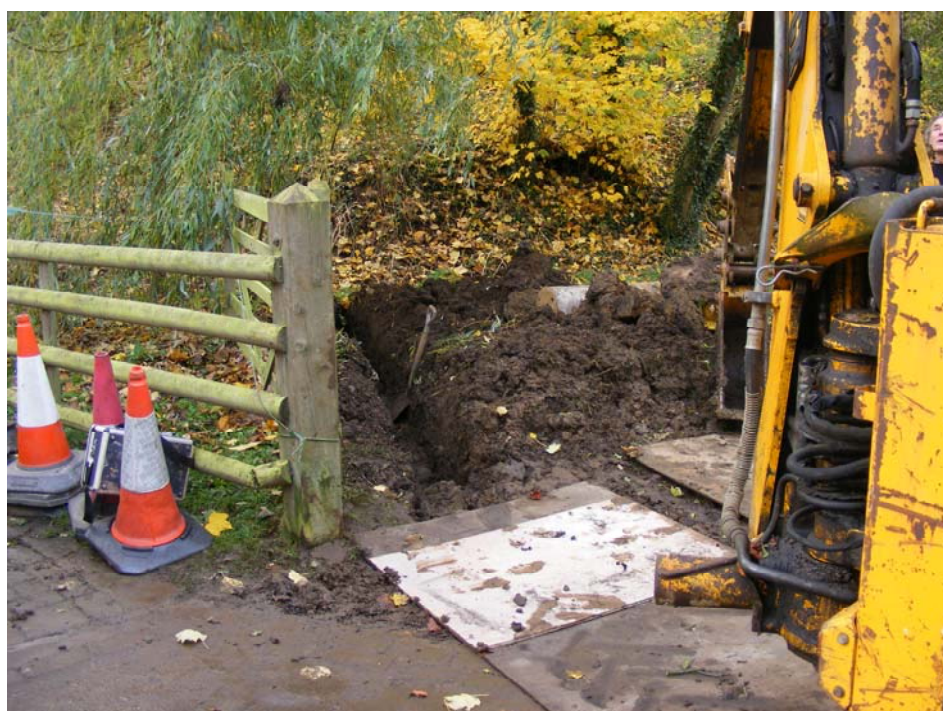
Plate 2: Services trench continued
