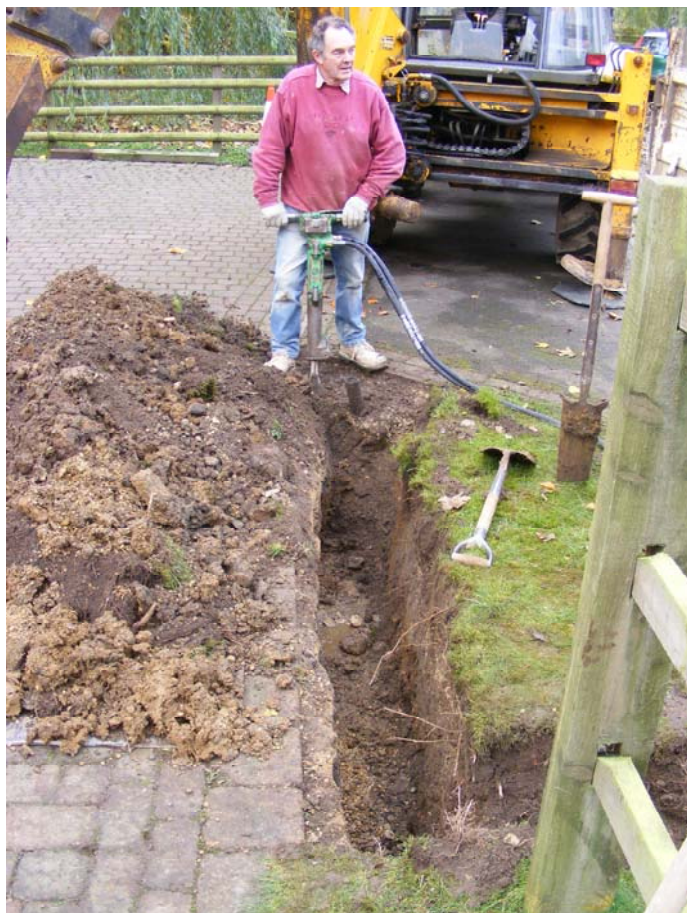
Plate 1: Services trench being excavated
