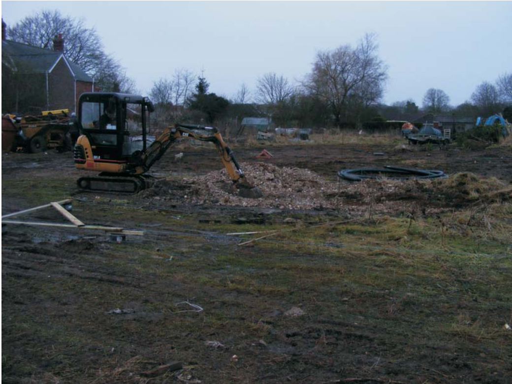
Photo No.1 Location of the proposed new build, within the southeast corner of the site. Chalk rubble hardcore being removed by the machine. Looking southwest.
